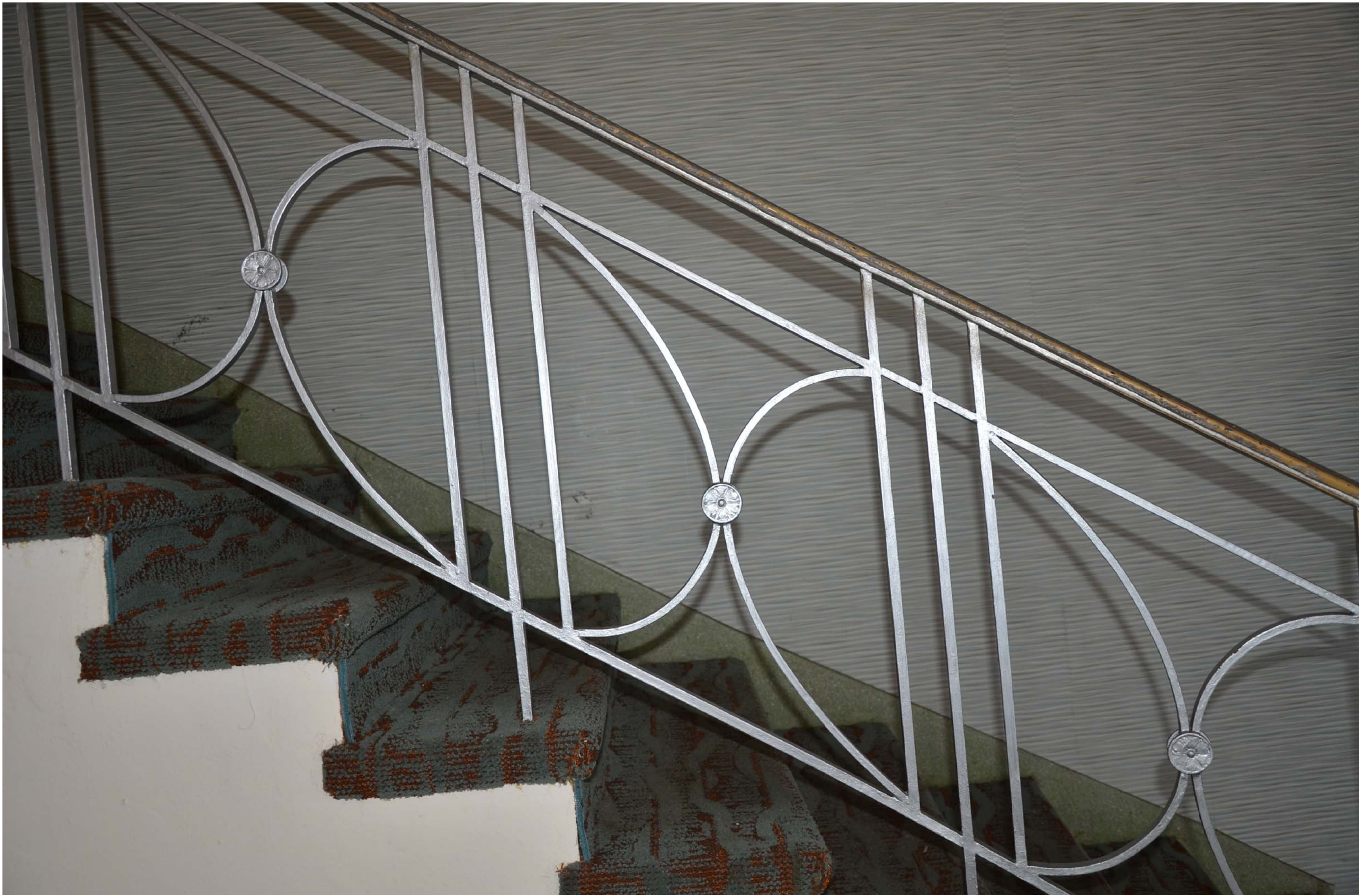
HISTORIC STAIR AND RAILING - KEYNOTE 7
