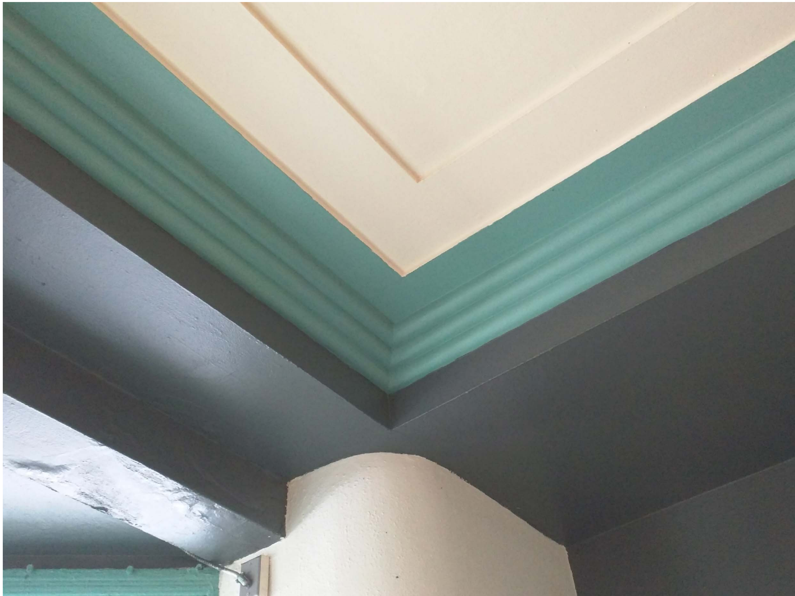
HISTORIC CEILING MOLDINGS AT RESTAURANT - KEYNOTE 8
