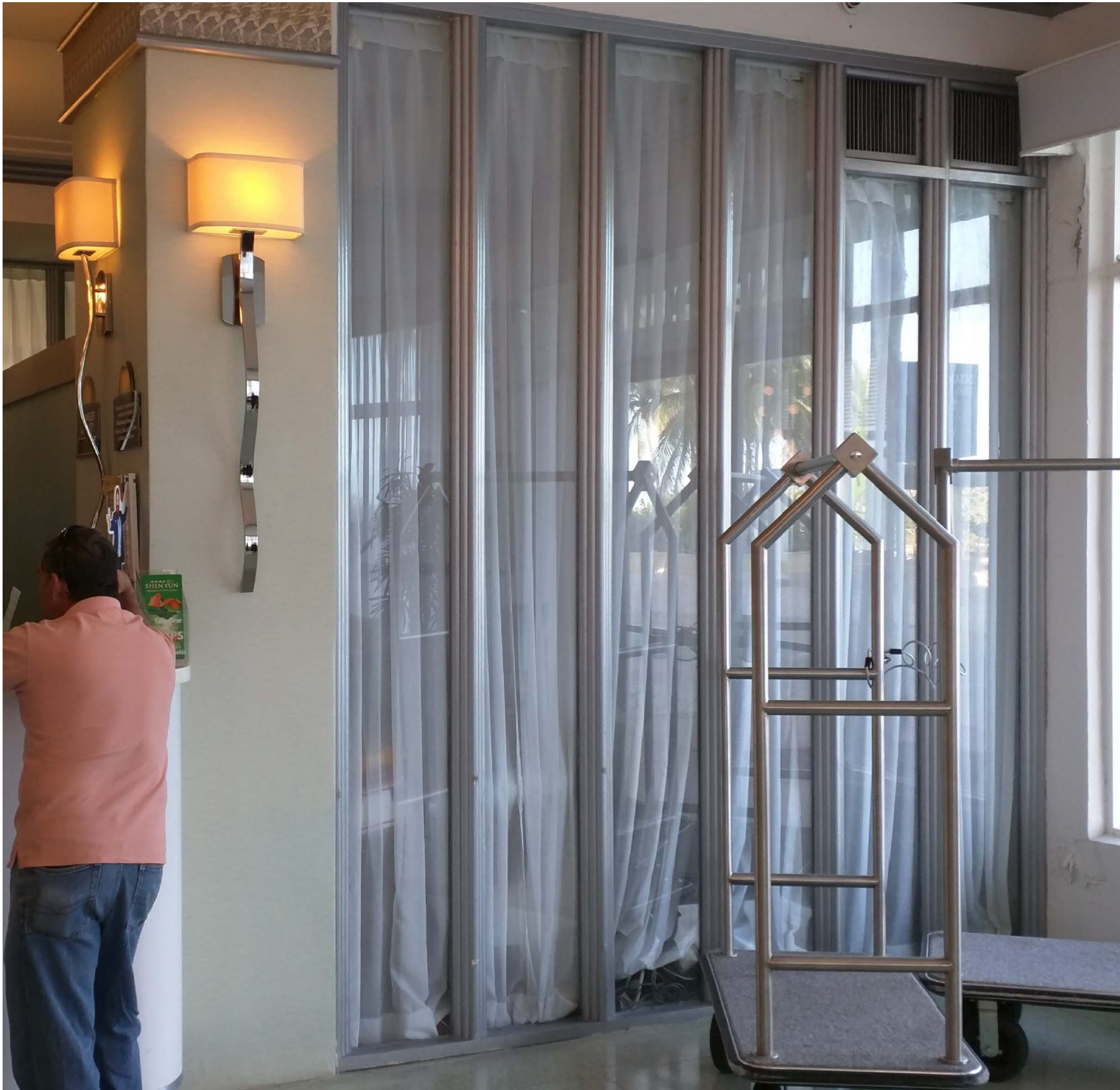
HISTORIC DECORATIVE WINDOW FRAMES - KEYNOTE 10
