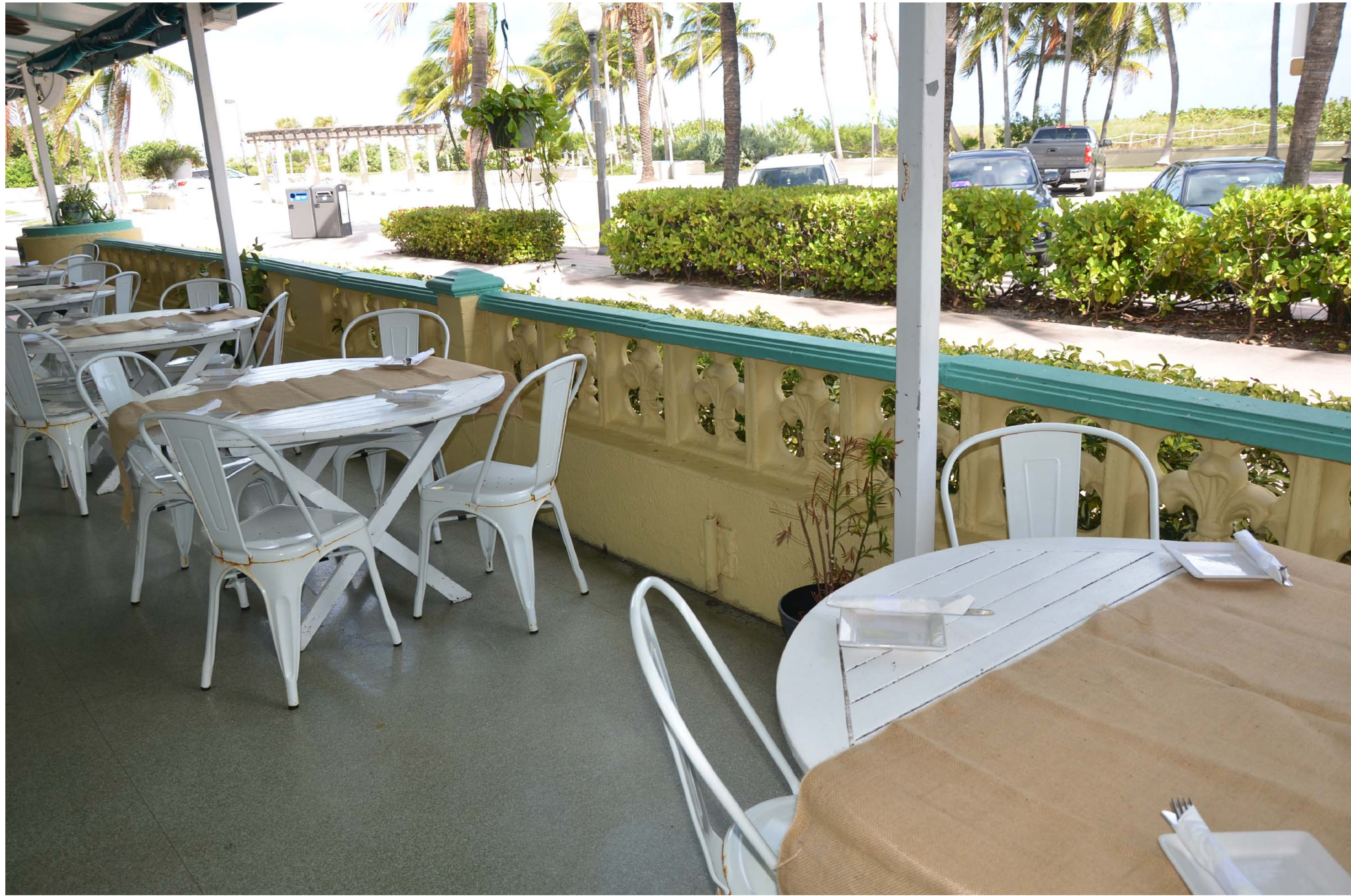
HISTORIC VERANDA GUARD RAIL - KEYNOTE 29
