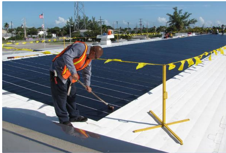
Picture 4: Installation of thin film solar panels at the Florida Keys Eco-Discovery Center.
