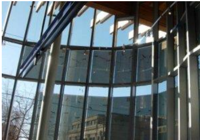
Picture 5: Thin film solar cells on windows at the Neighborhood Service Center in Seattle, WA.
