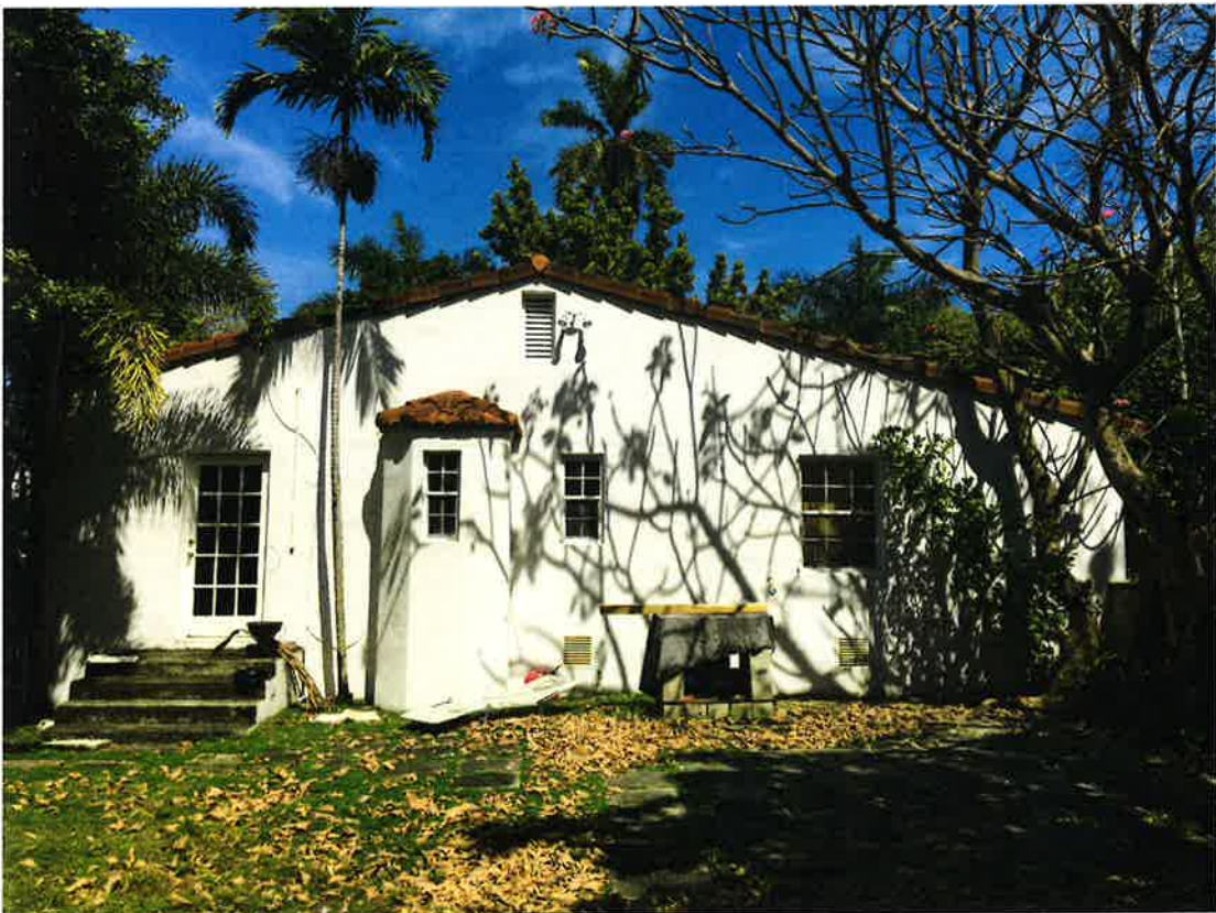
03 - SOUTH SIDE FACADE
