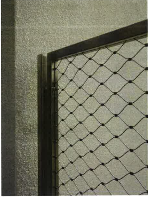
METAL WIRE MESH FOR ALL RAILINGS M-01
