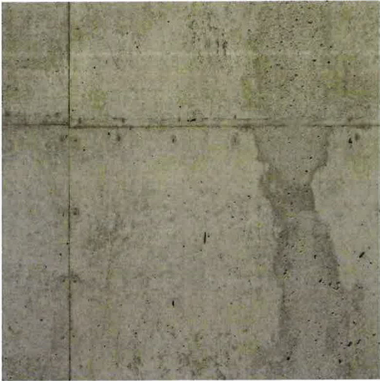
EXPOSED CONCRETE C-02
