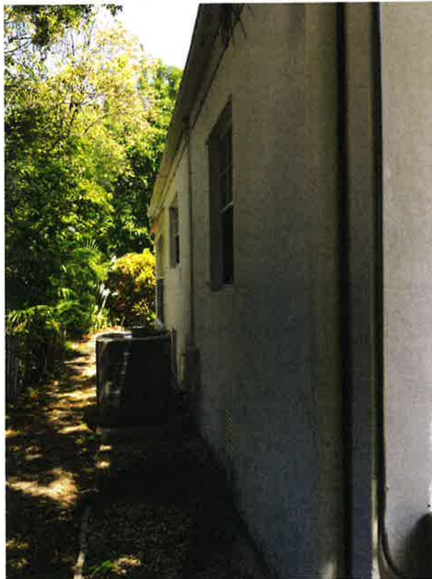
04 - INTERIOR SIDE YARD (03/16/2017)
