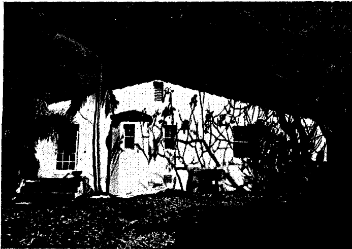
03 - SOUTH SIDE FACADE
