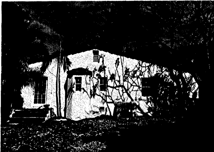
03 - SOUTH SIDE FACADE
