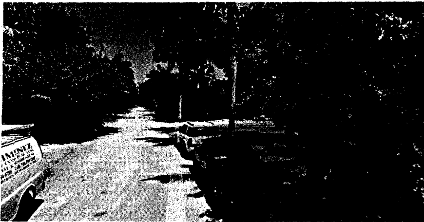
03 STREET VIEW LOOKING WEST
