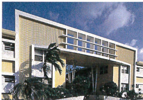
350 South Shore Drive/Miami Beach 1954 A common building type in North Beach, the two-tier condo is unified by a strong facade frame comprised of decorative struts or parapet walkways, often convex as in this case, and often mixing two-toned, cladded and textured surfaces.
