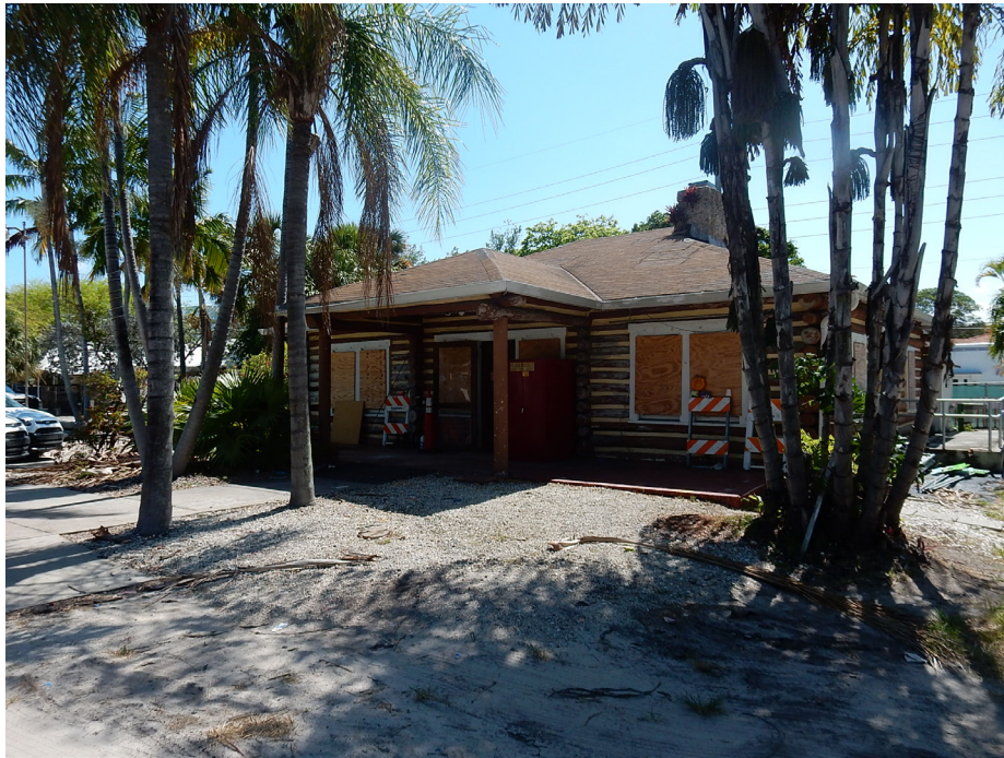
Log Cabin Exterior - East
