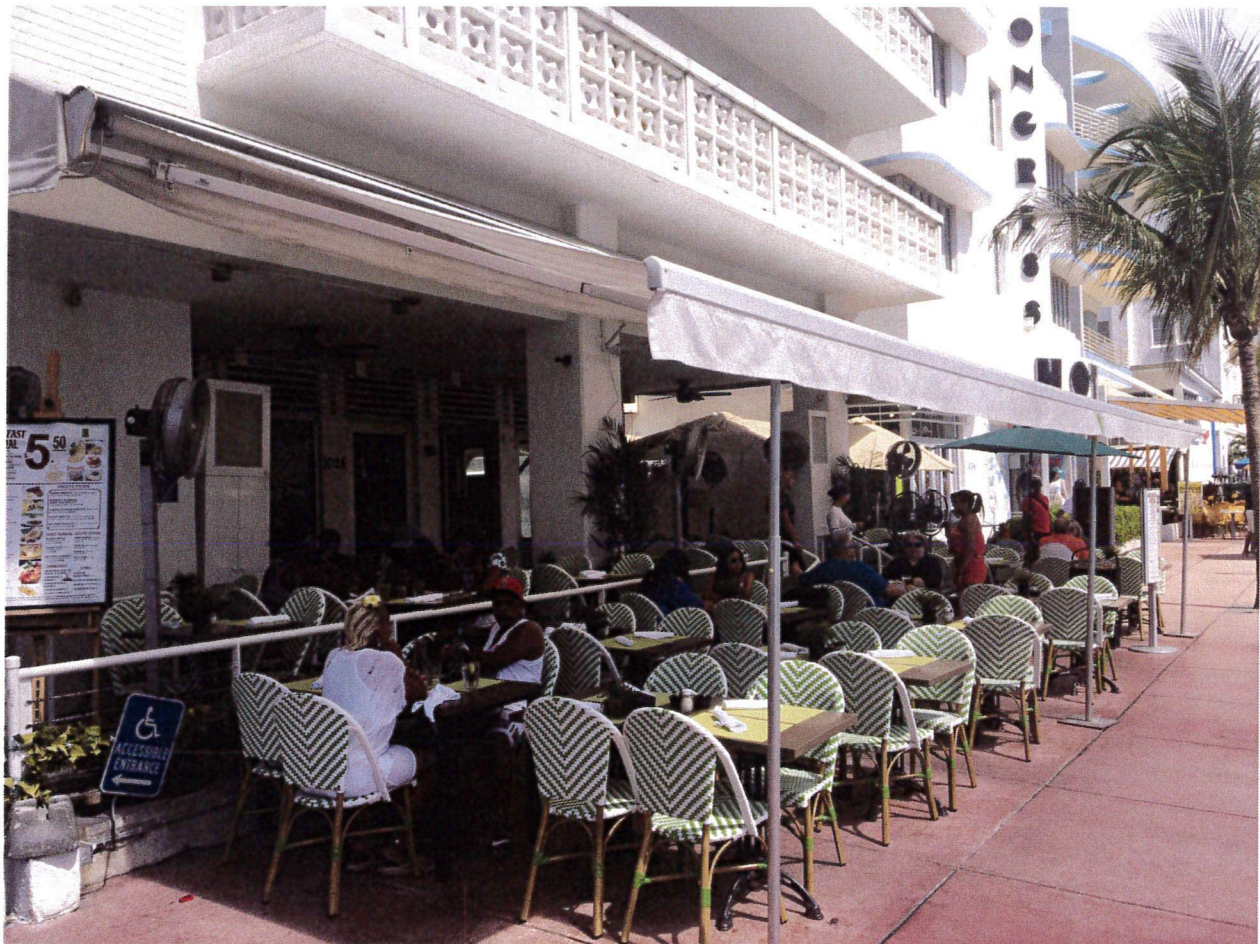
Unpermitted retractable awning structure with vertical supports in the right-of-way attached to an unpermitted fixed awning structure, August 2017
