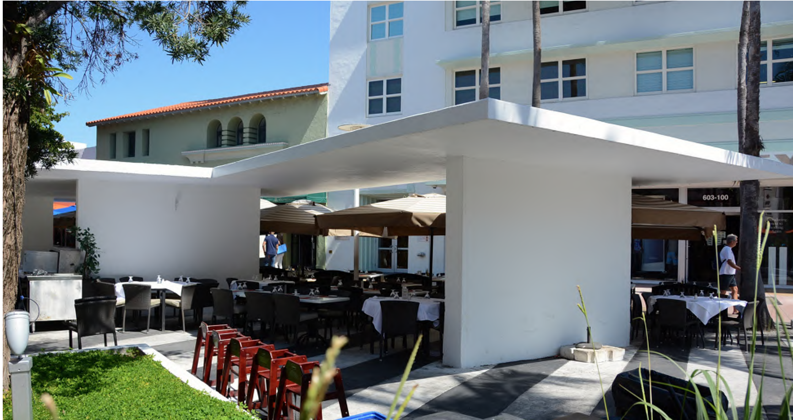
EXISTING CONDITION - FALL 2016
