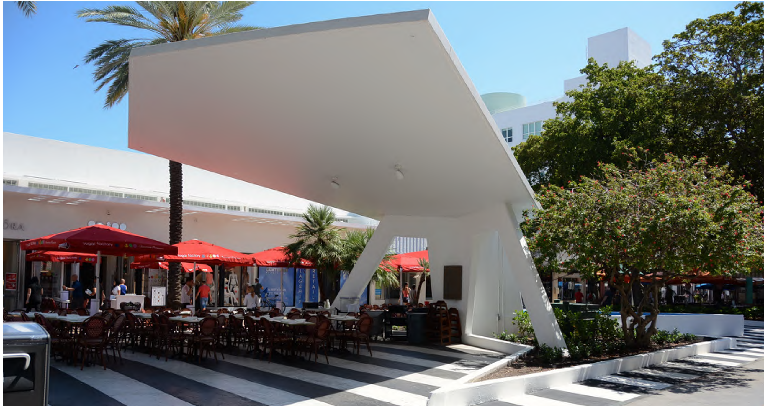
EXISTING CONDITION - FALL 2016
