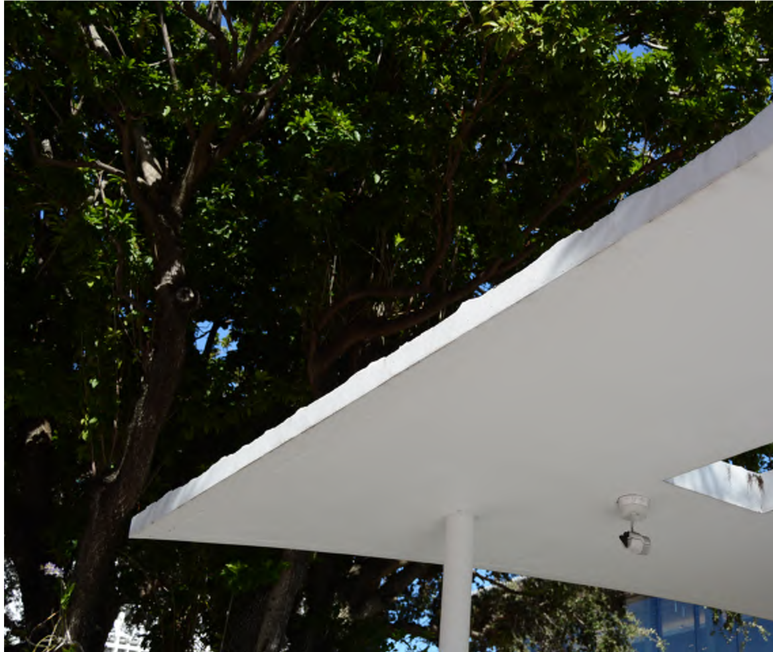
EXISTING CONDITION - FALL 2016
