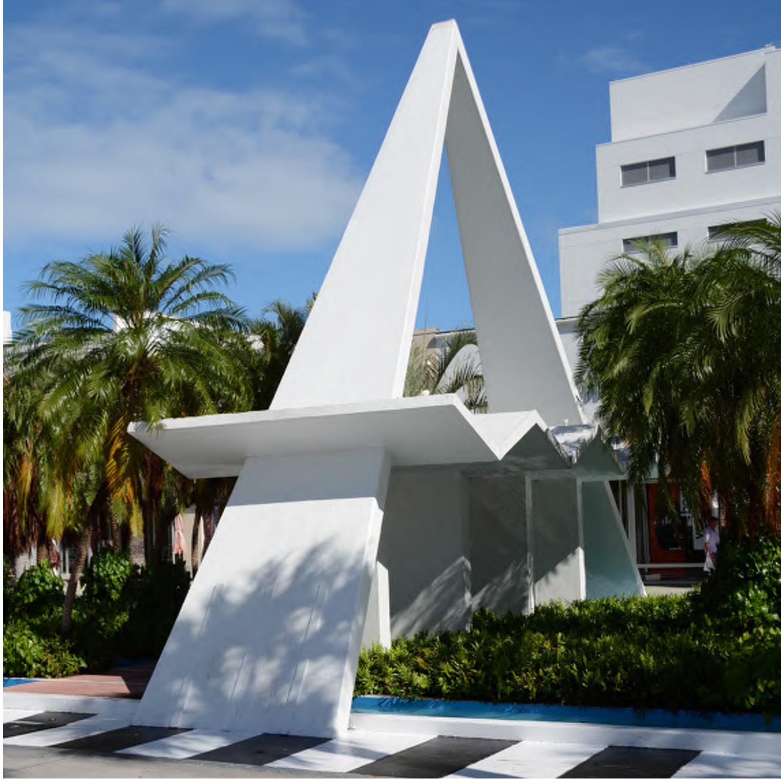
EXISTING CONDITION - FALL 2016
