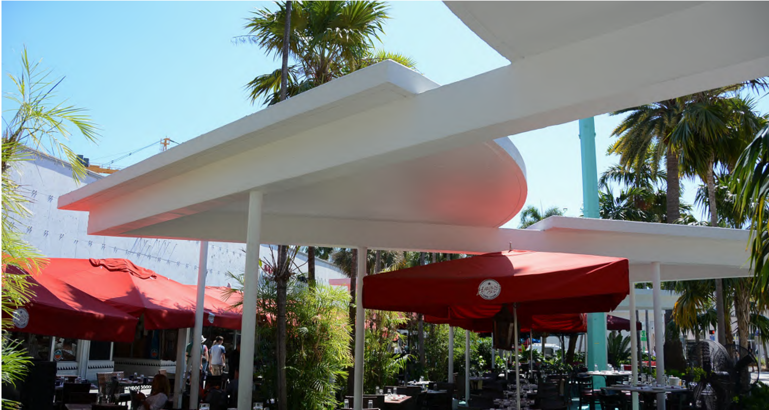
EXISTING CONDITION - FALL 2016
