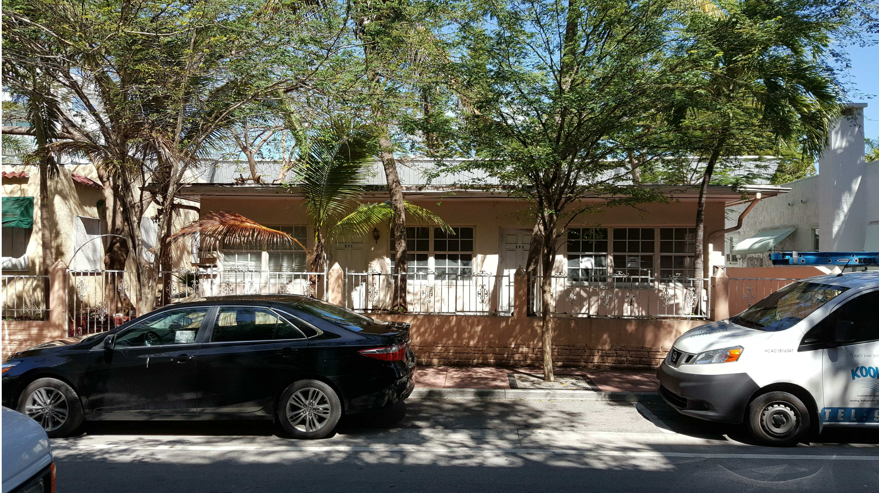
809 2ND ST. SOUTH FACADE
