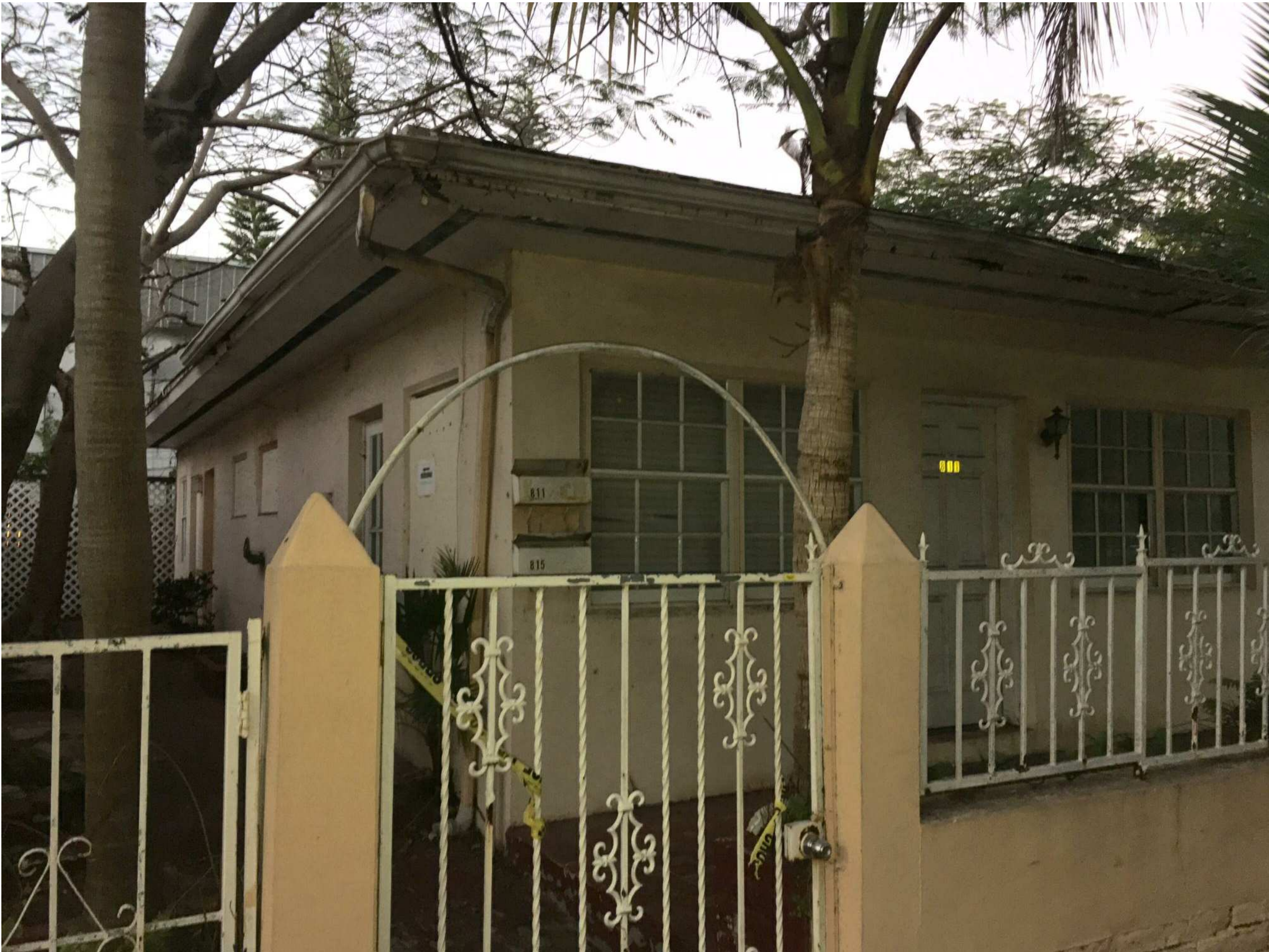
809 2ND ST. SOUTH-WEST CORNER
