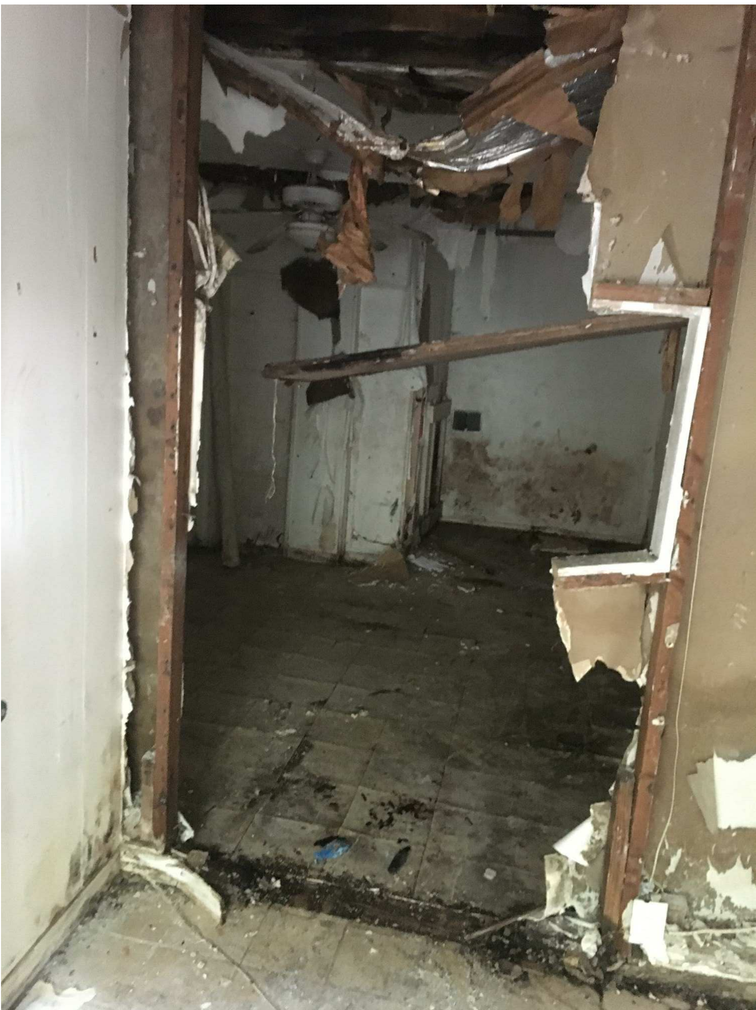
EXISTING BUILDING INTERIOR VIEW AT BEDROOM
