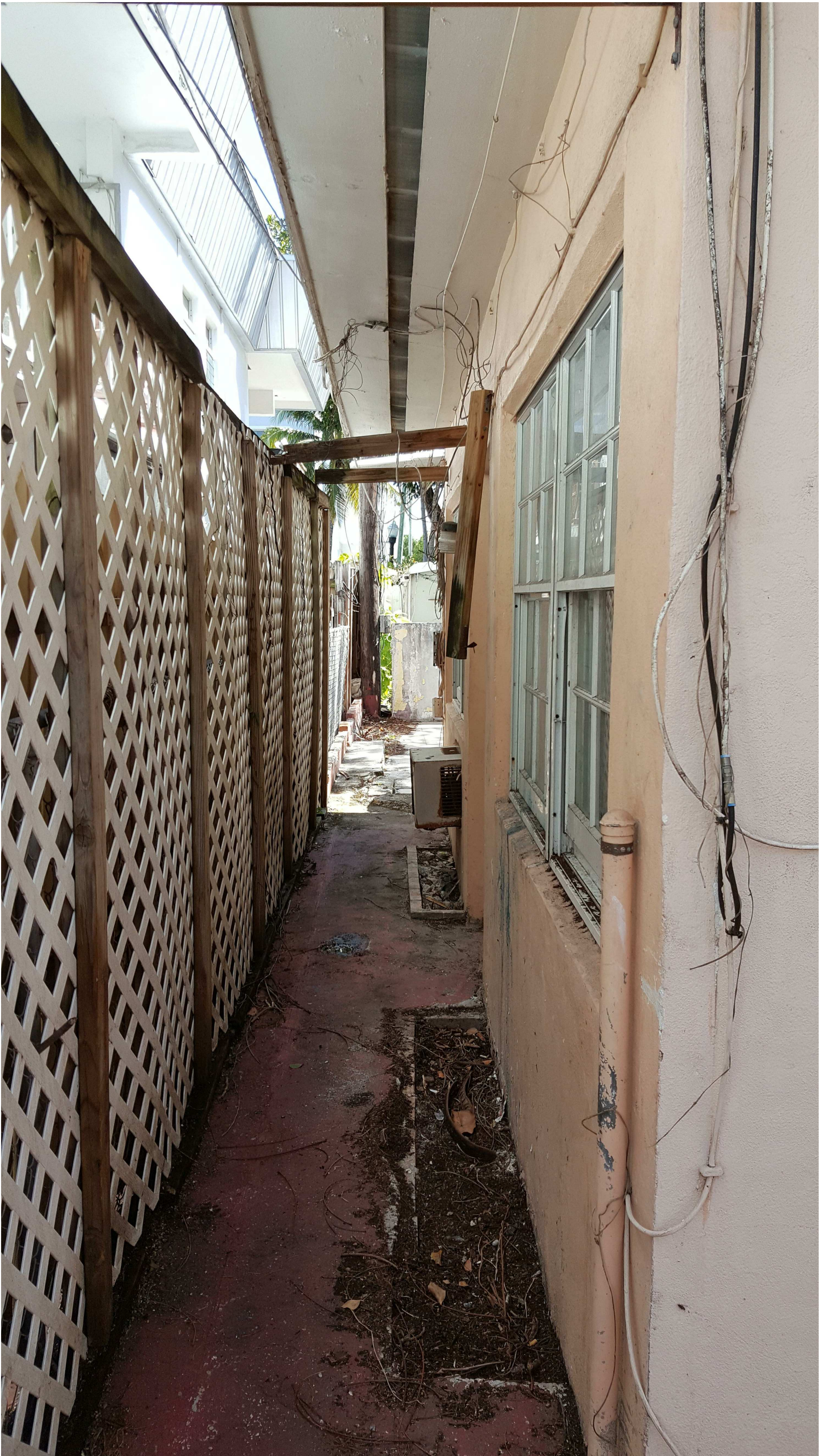
809 2ND ST. NORTH ELEVATION (REAR)
