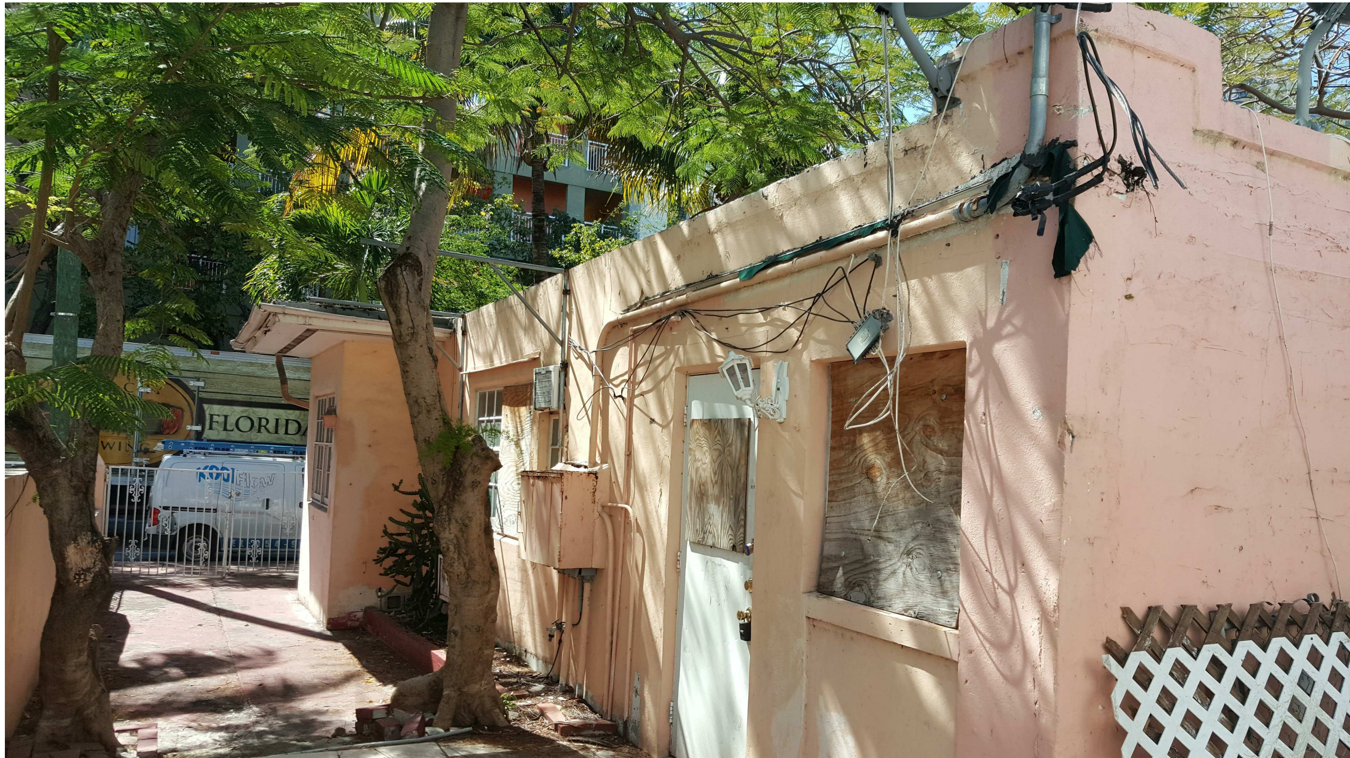
809 2ND ST. EAST ELEVATION (FROM NORTH)
