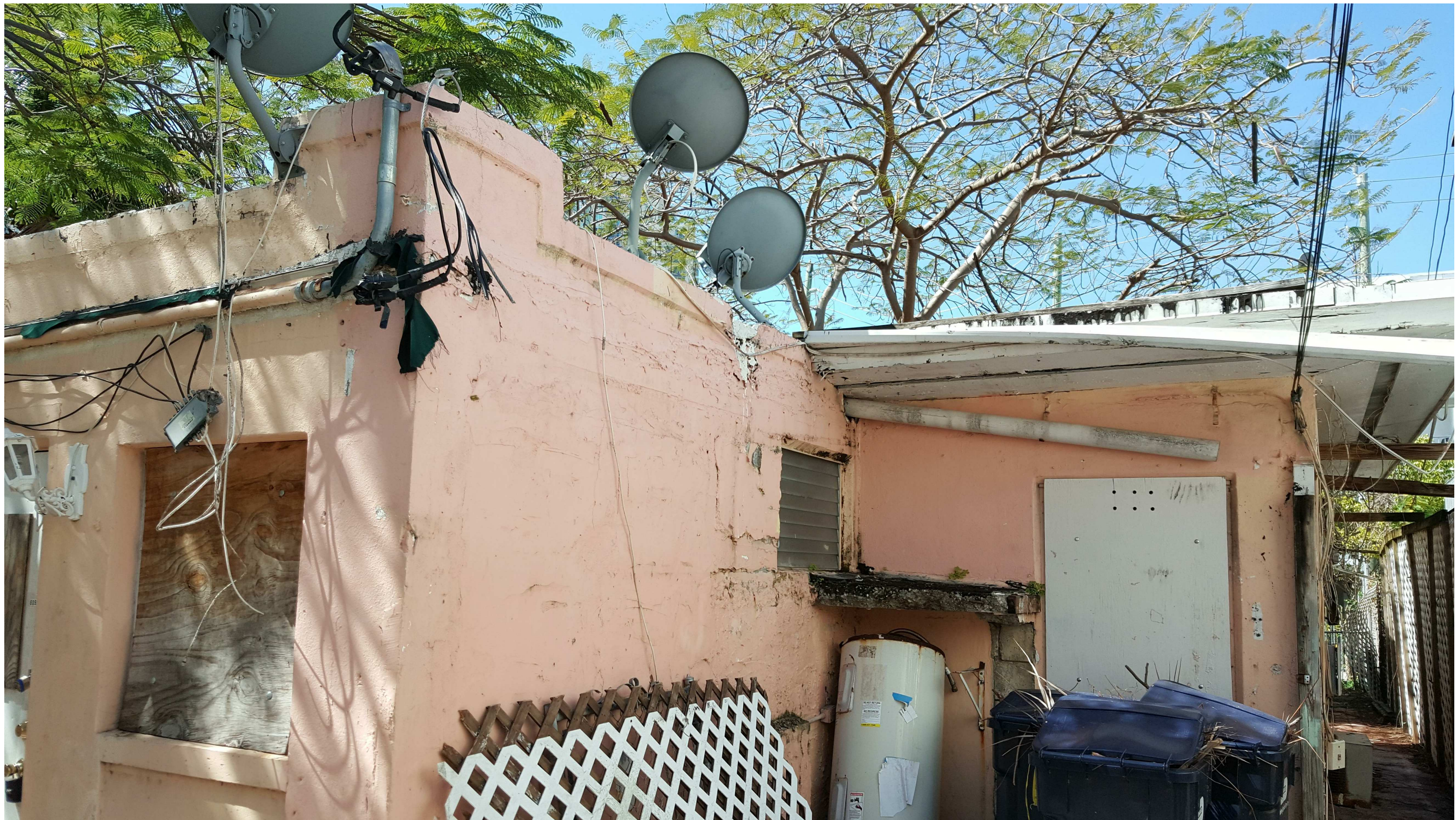
809 2ND ST. EAST ELEVATION (FROM NORTH)
