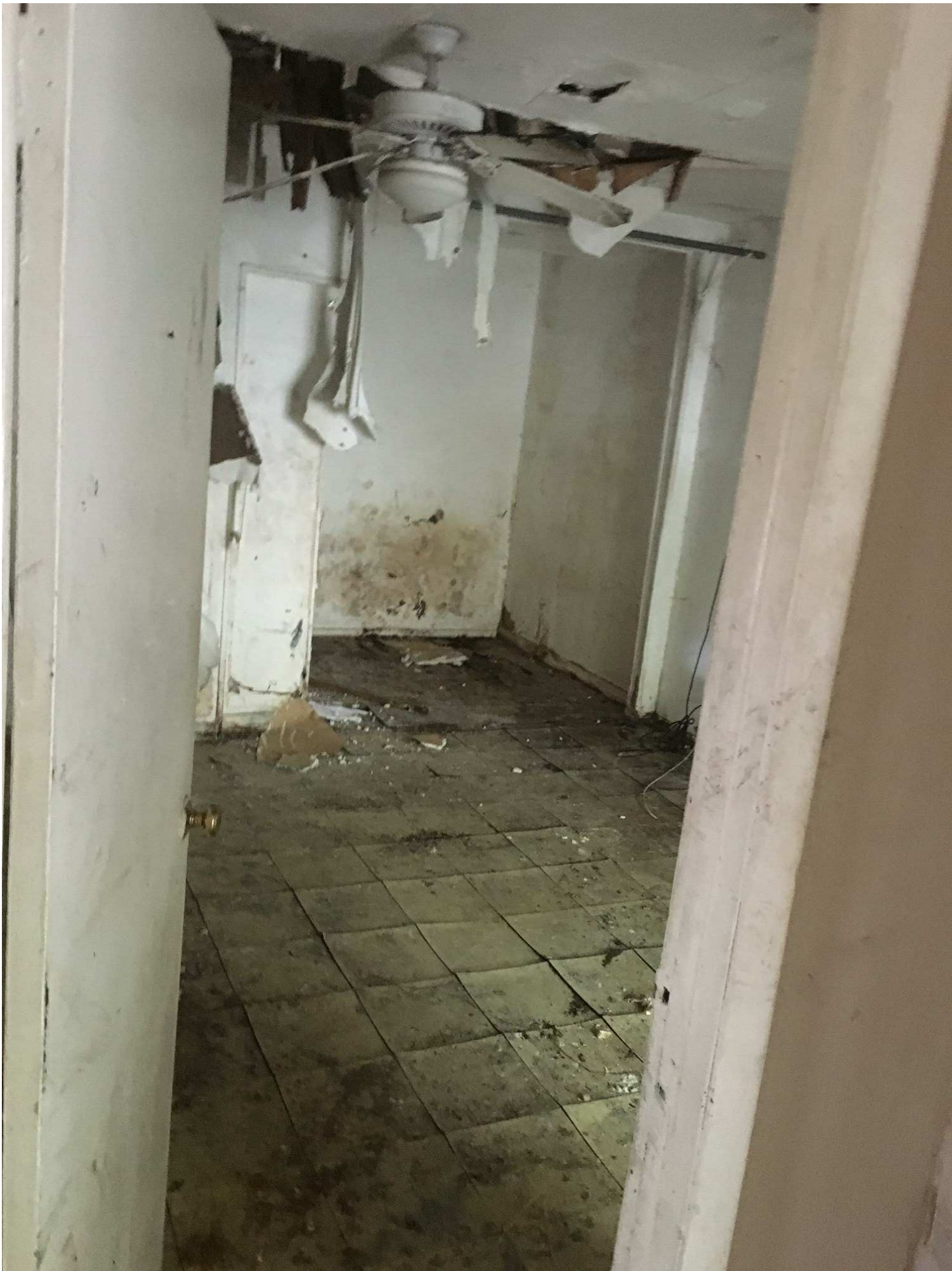
EXISTING BUILDING INTERIOR VIEW AT BEDROOM
