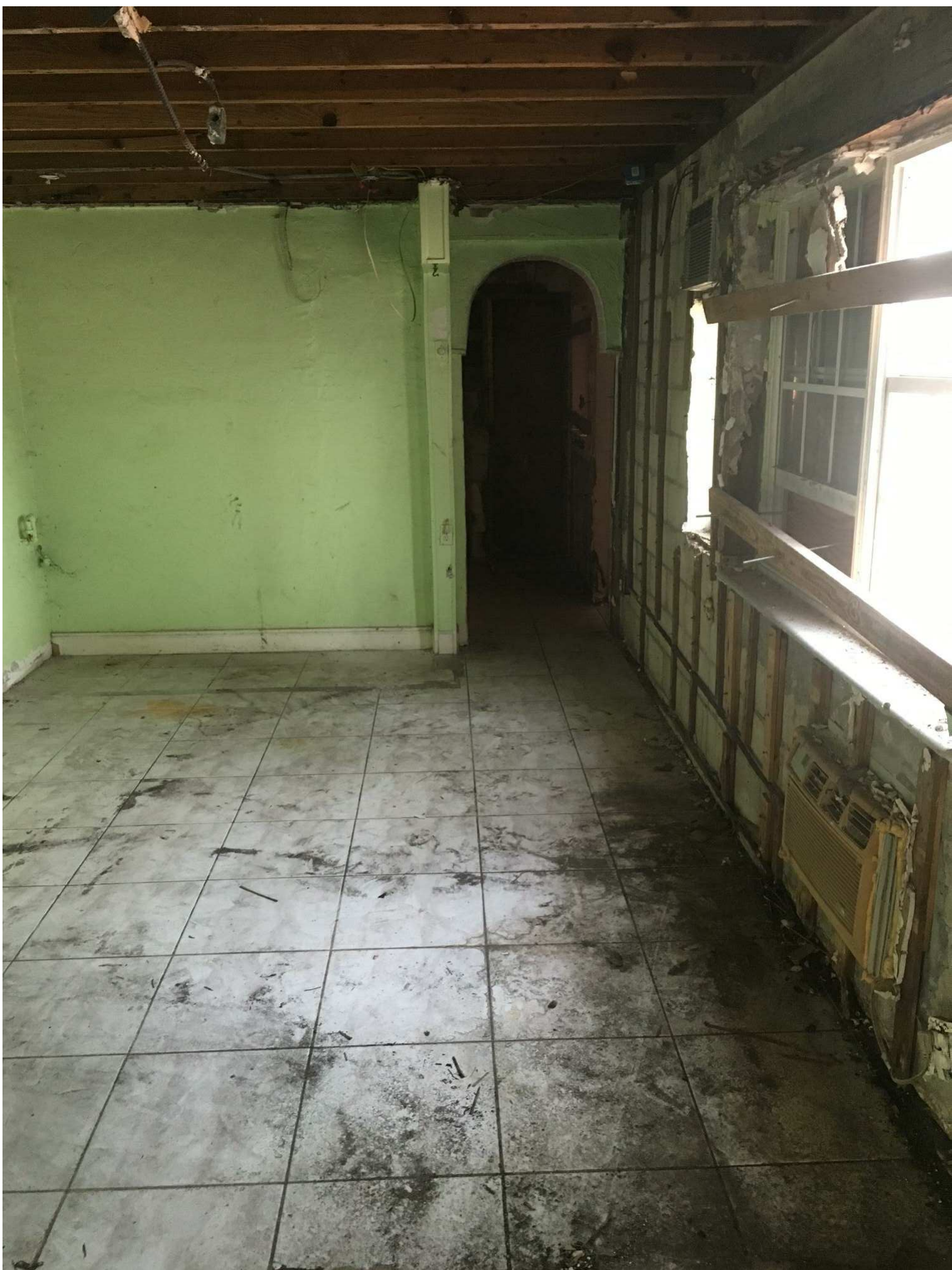
EXISTING BUILDING INTERIOR VIEW AT LIVING ROOM
