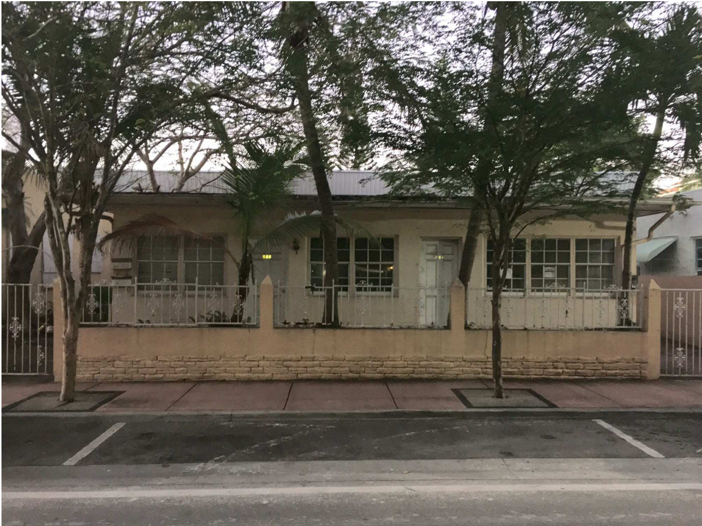
809 2ND ST. SOUTH FACADE
