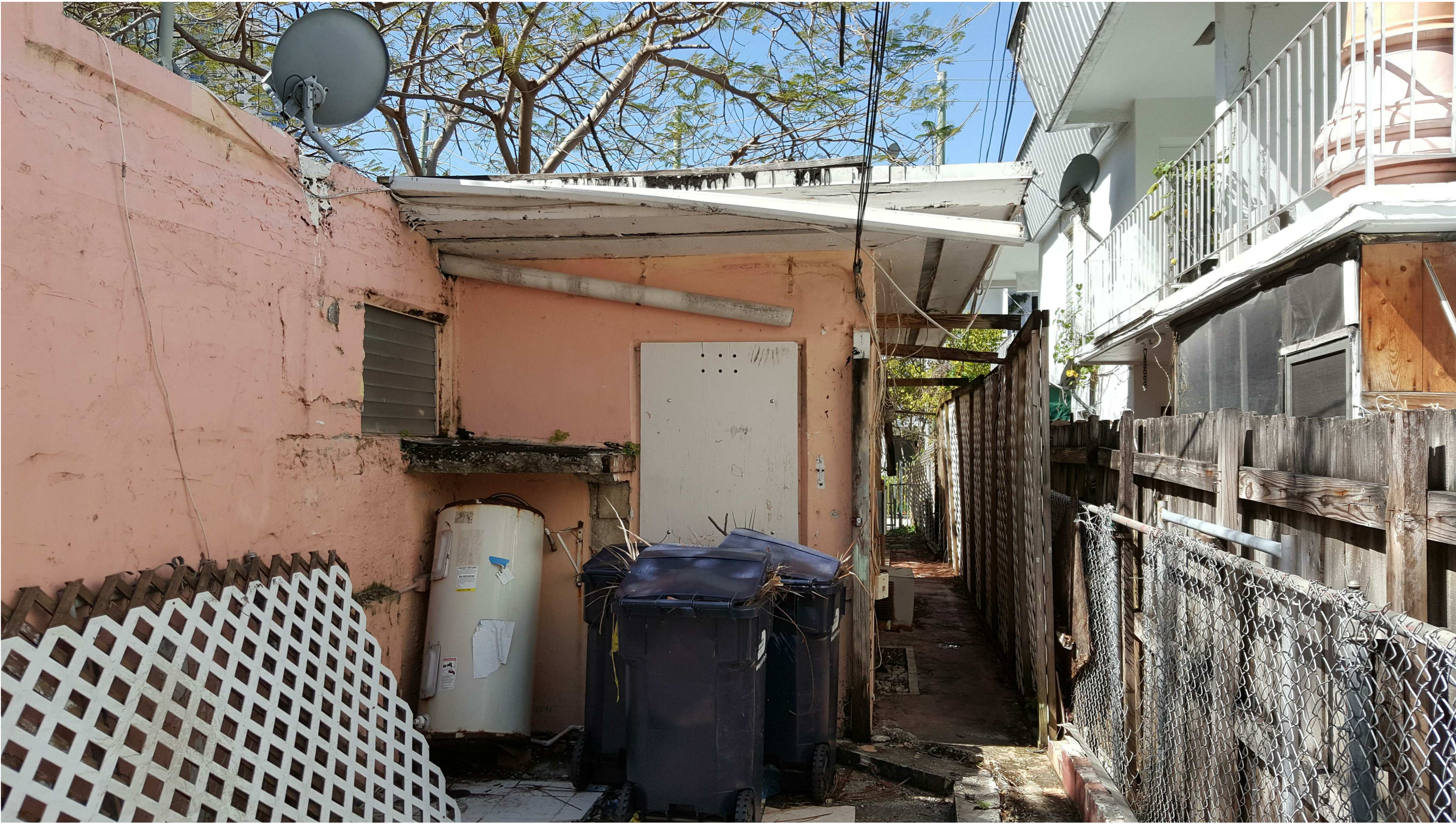
809 2ND ST. EAST ELEVATION (NORTH END)
