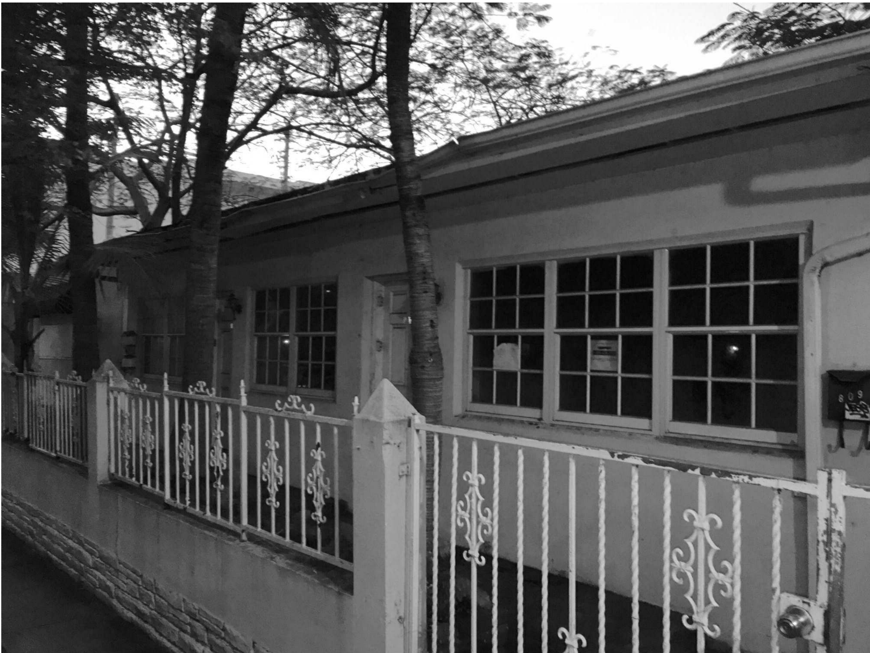
809 2ND ST. SOUTH ELEVATION (FROM EAST)
