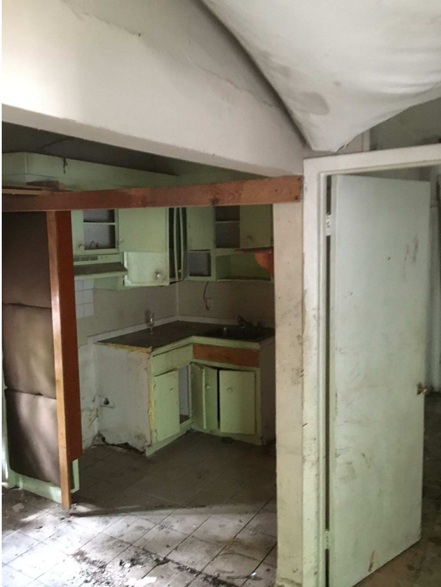
EXISTING BUILDING INTERIOR VIEW AT KITCHEN
