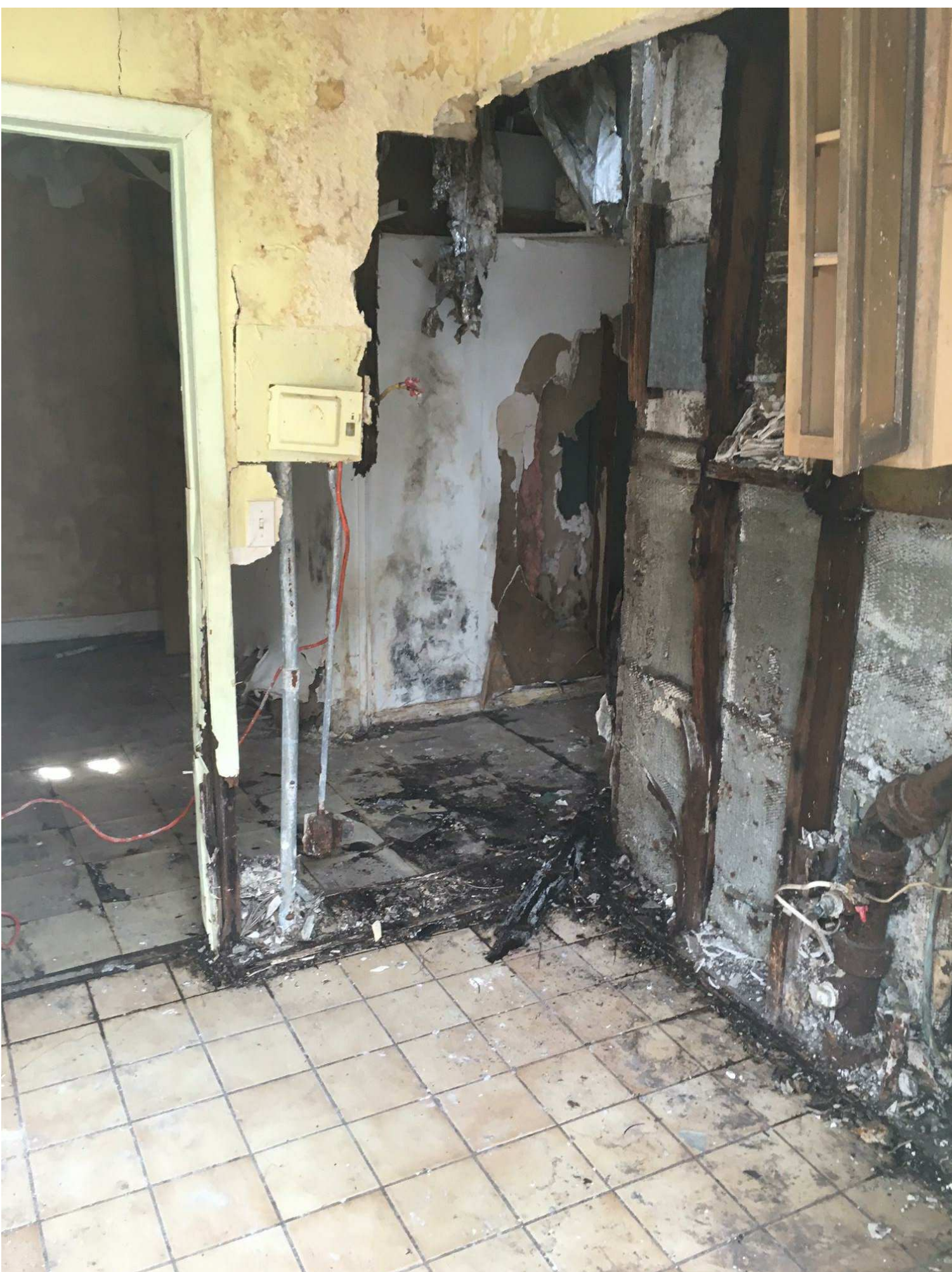
EXISTING BUILDING INTERIOR VIEW AT BATHROOM
