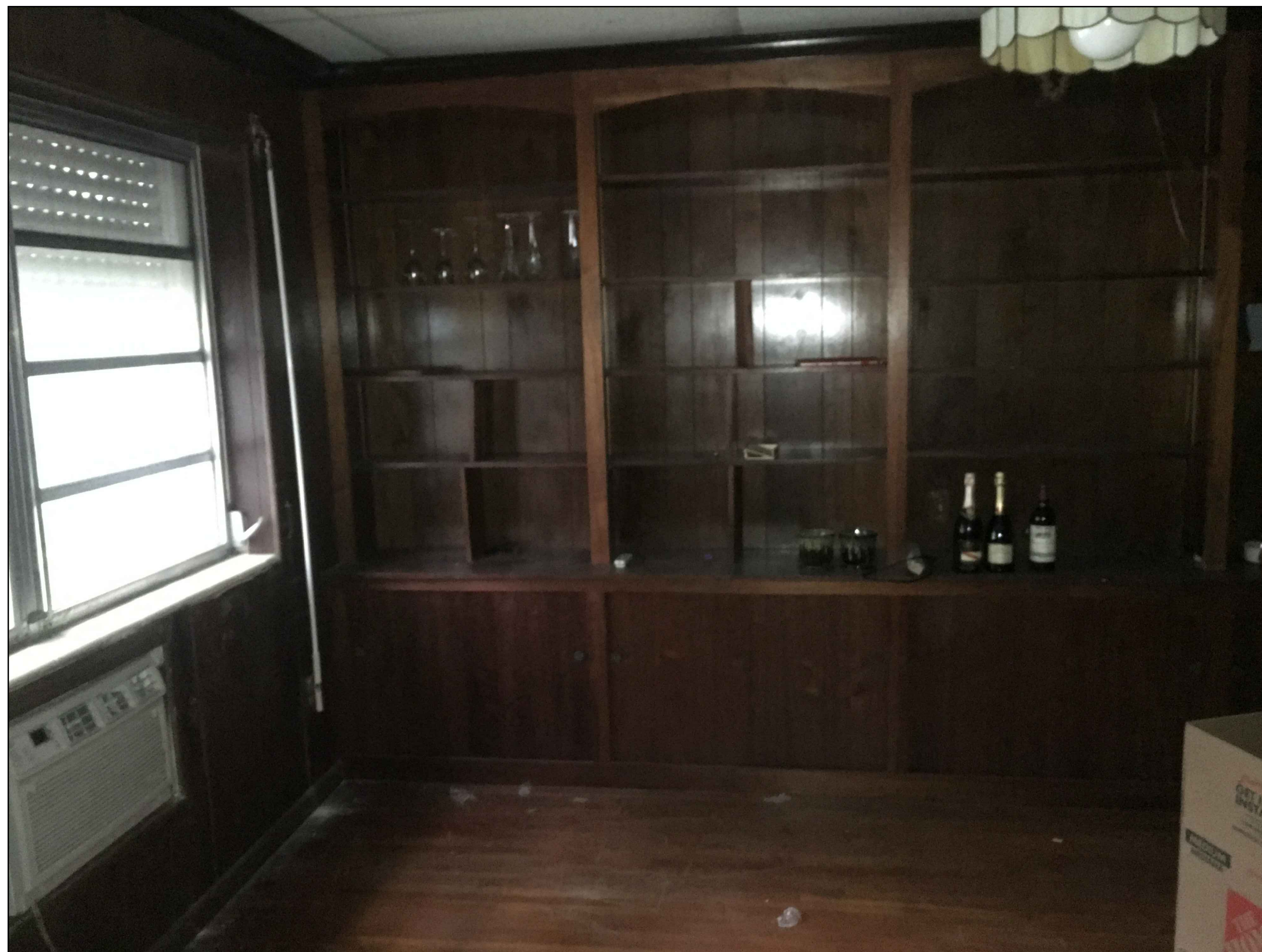
Ⓔ13 (03/04/2016) EXISTING EAST ADDITION
