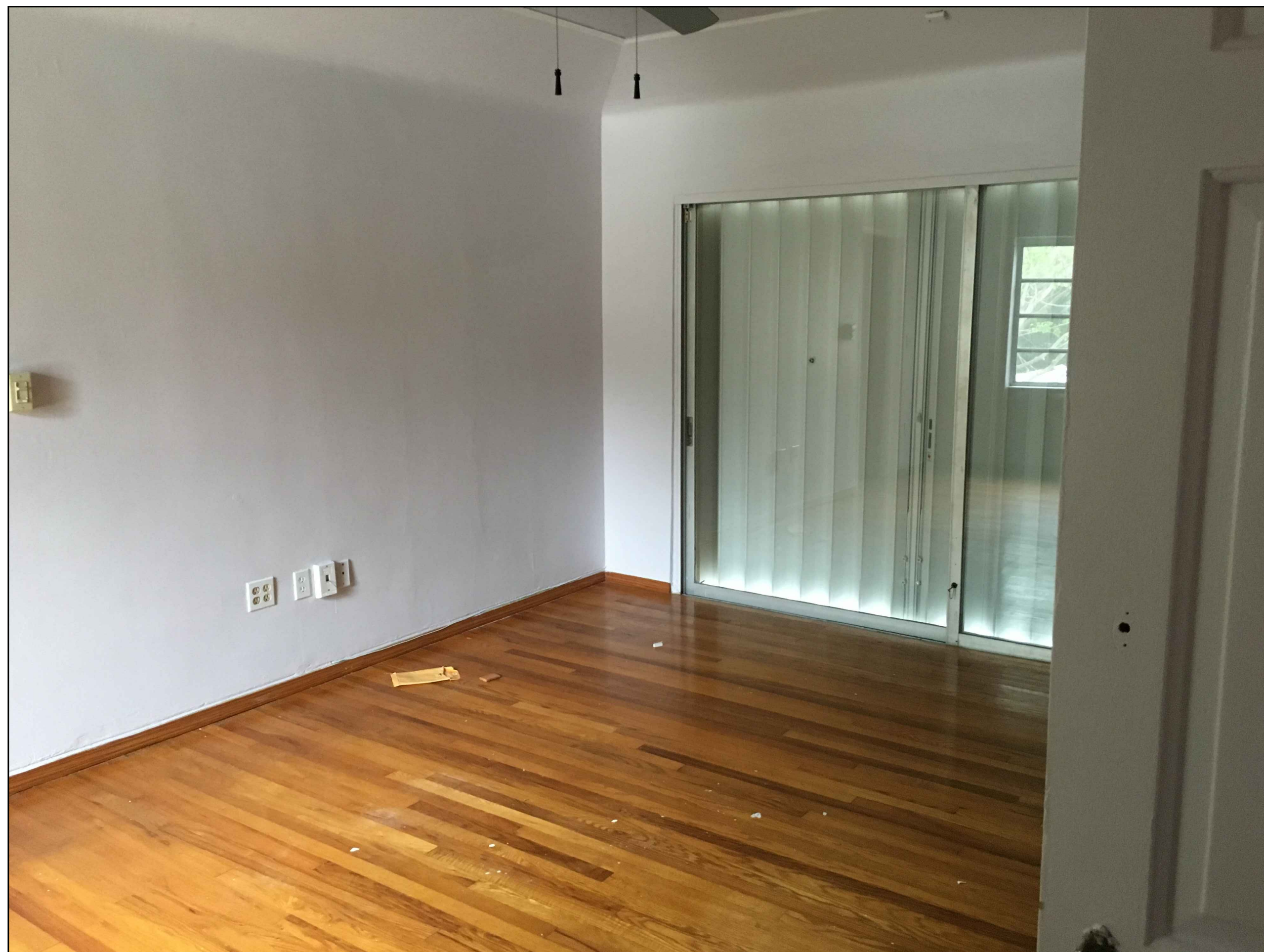
Ⓔ21 (03/04/2016) EXISTING MASTER BEDROOM
