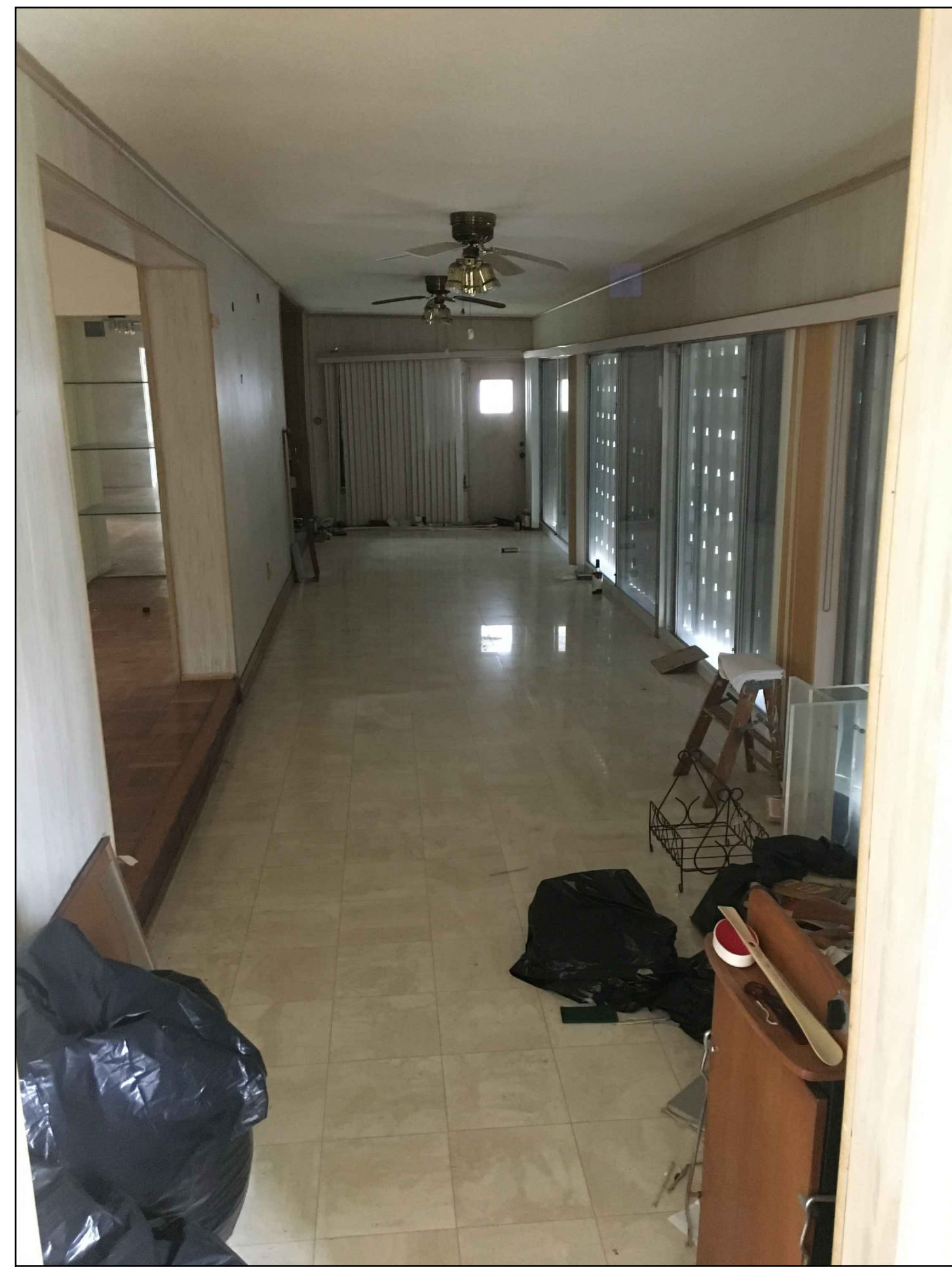
Ⓔ15 (03/04/2016) EXISTING FLORIDA ROOM ADDITION
