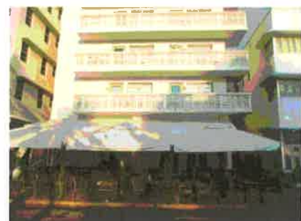
BUILDING FRONT VIEW
