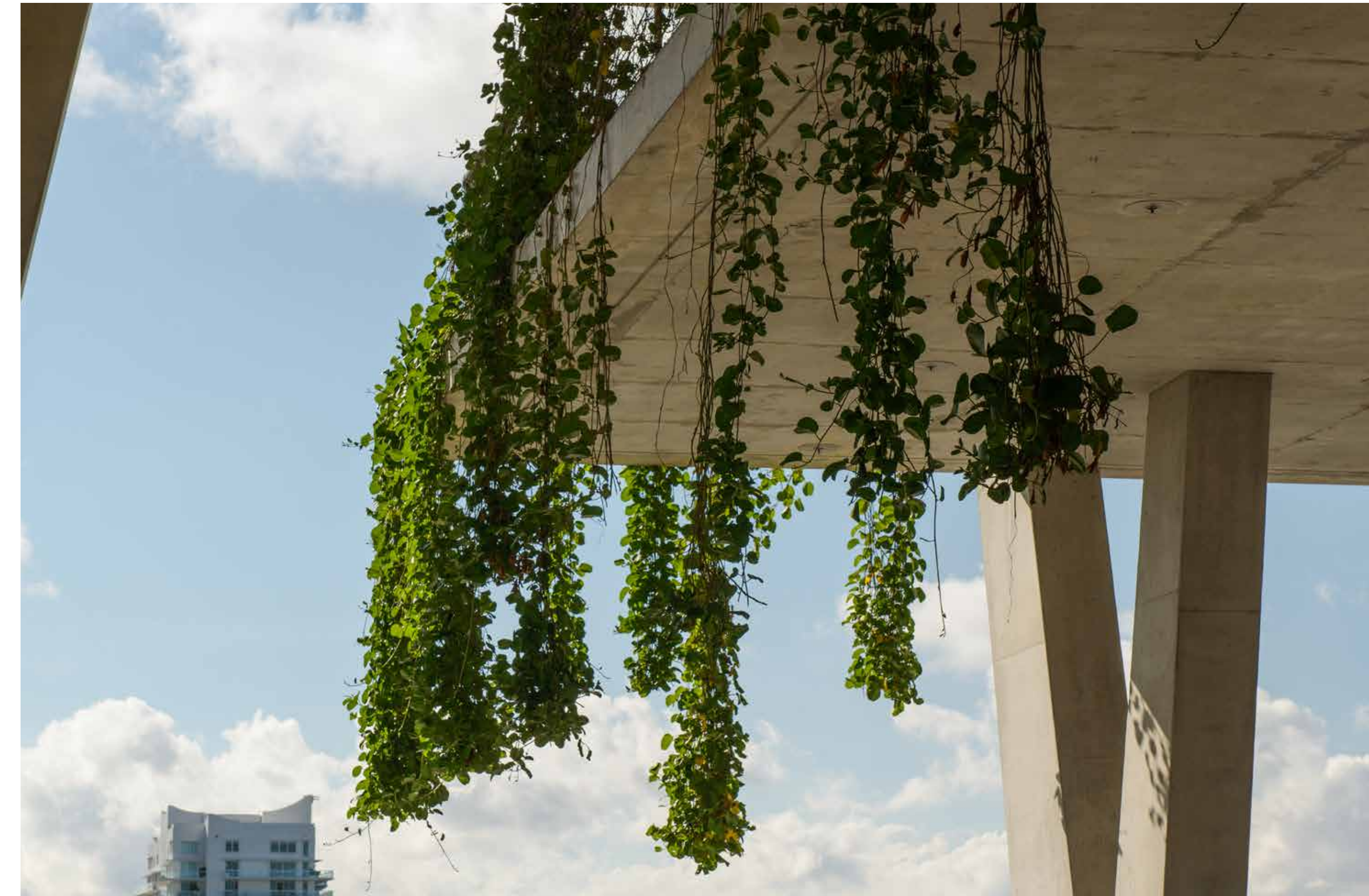
CANTILEVERED CONCRETE ROOF WITH CASCADING VINES
