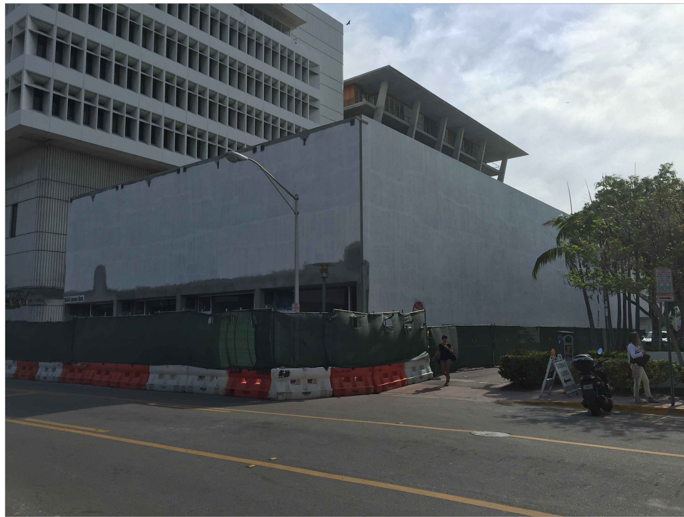
NORTH EAST CORNER OF SUBJECT PROPERTY
