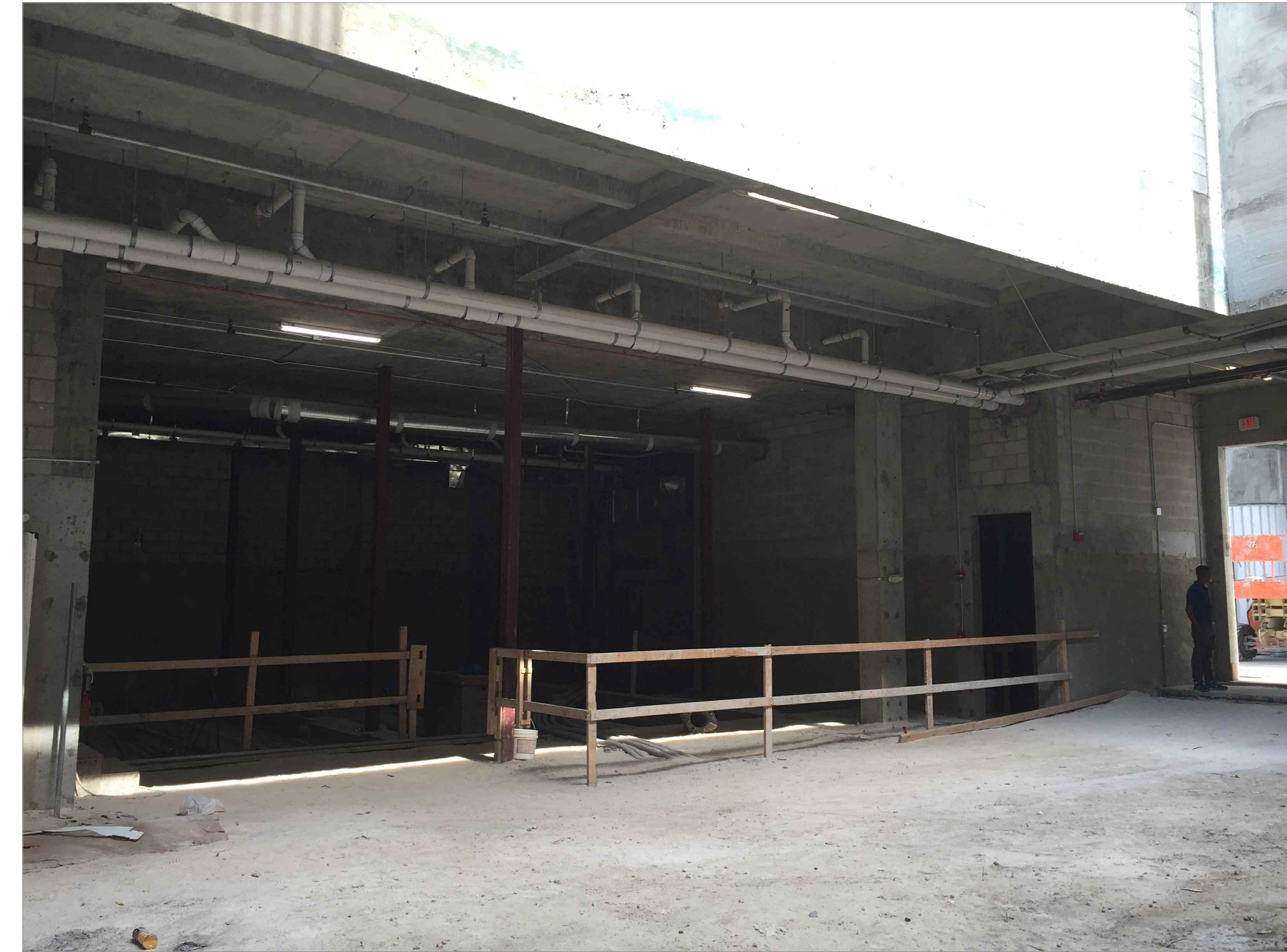
INTERIOR: SOUTH EAST VIEW
