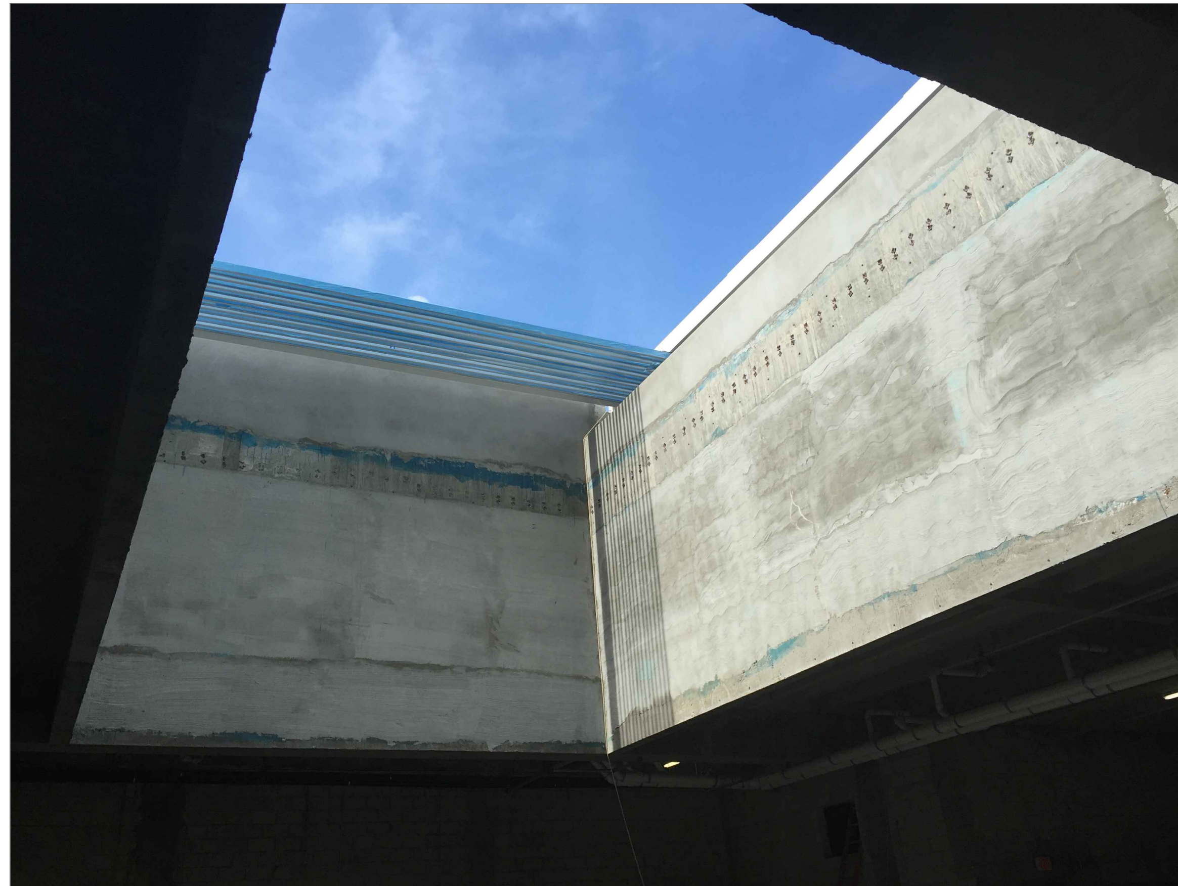
INTERIOR: NORTH EAST VIEW OF ROOF OPENING
