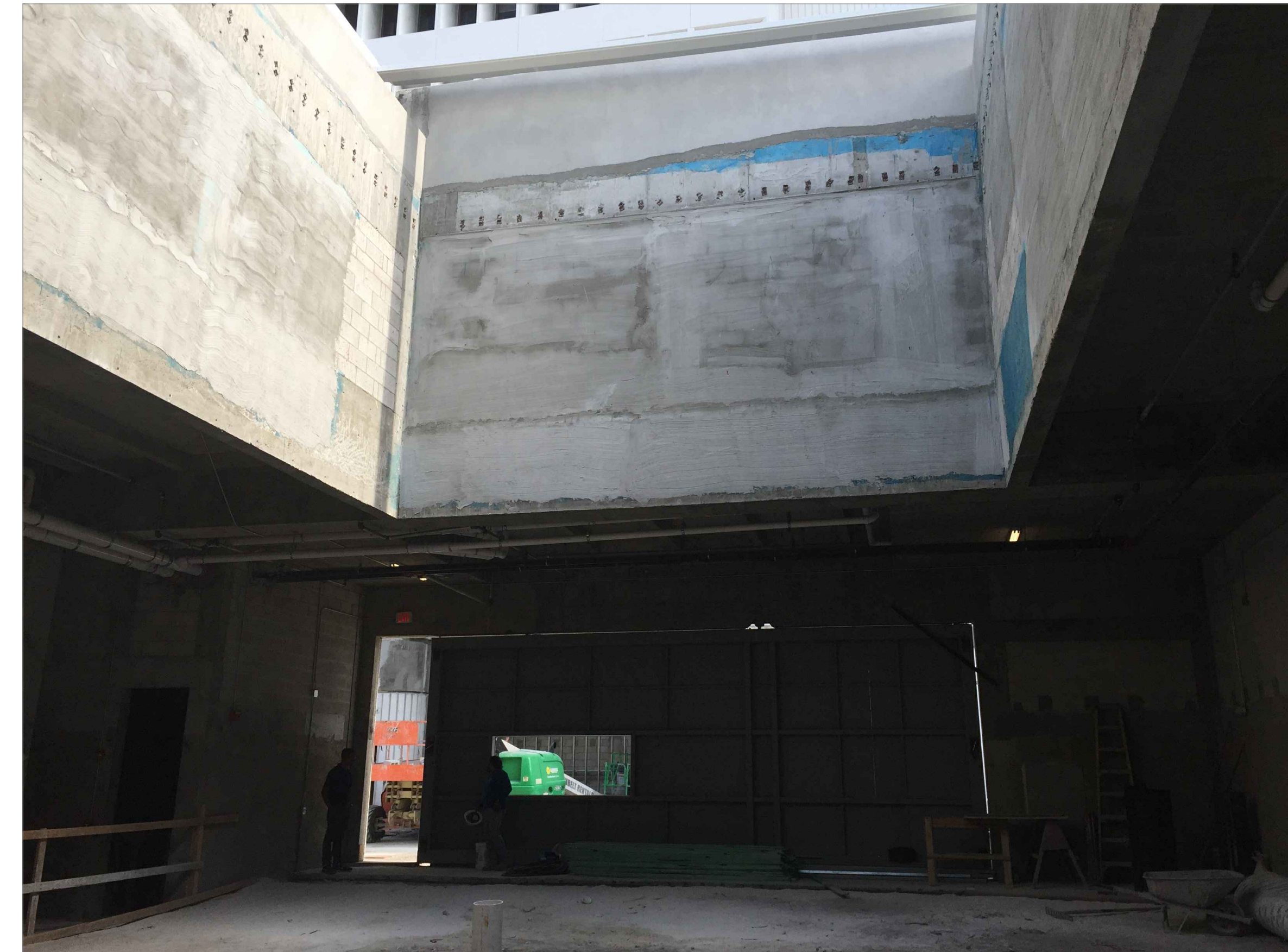
INTERIOR: SOUTH VIEW
