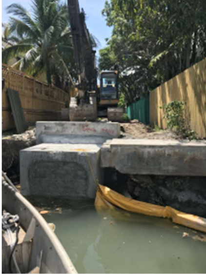
Figure 6: Outfall below construction with open soil surface
