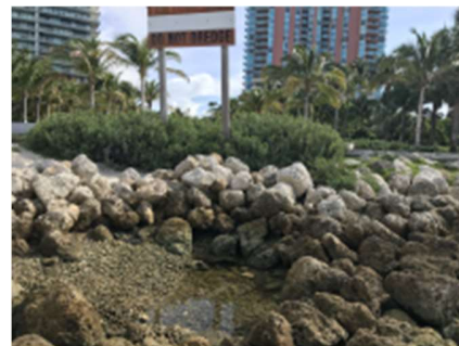
Figure 5: Rip-rap energy dissipation near outfall
