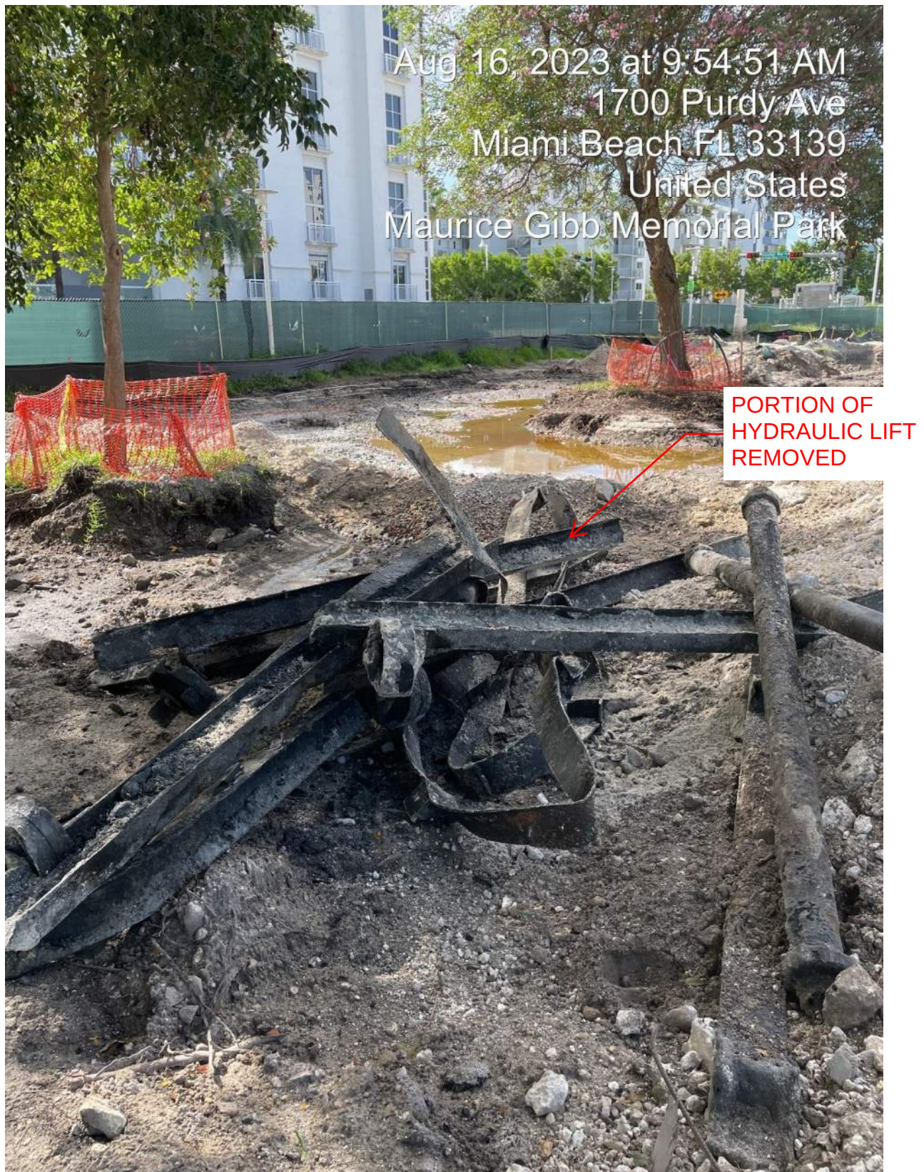
Area F: Portions of hydraulic lift exposed and removed.
