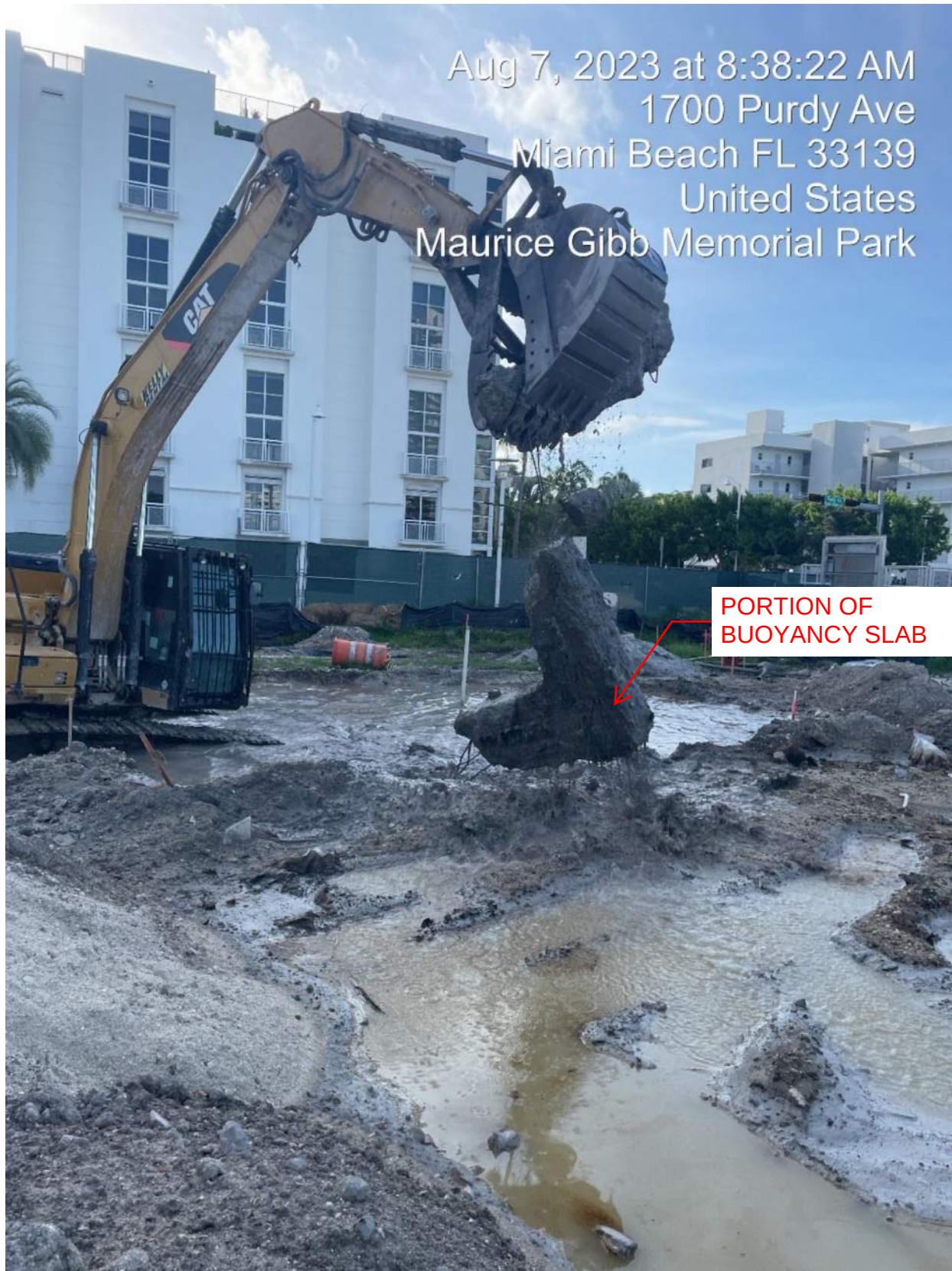
Area D: Concrete slab removed in search of source of fuel encountered.
