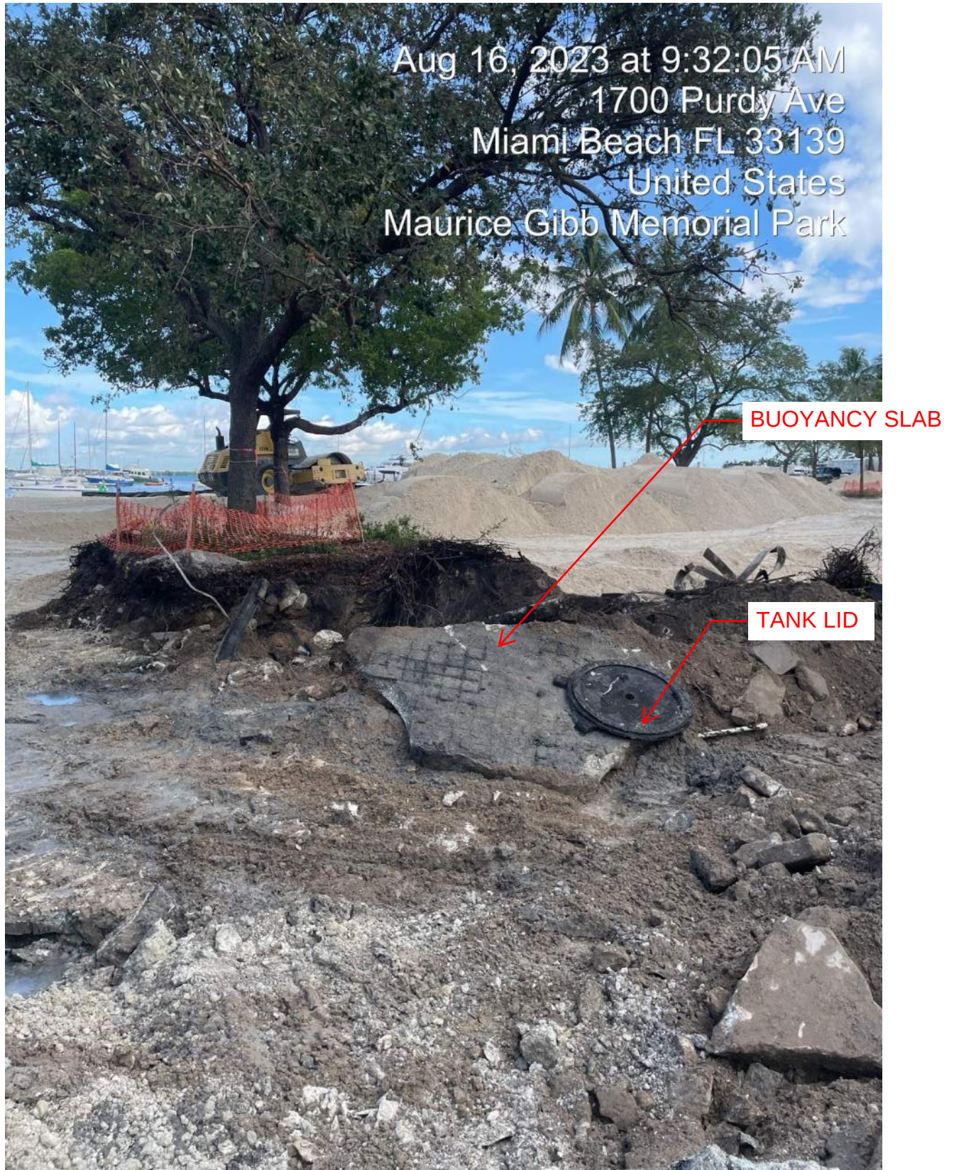
Area F: Concrete slab removal exposed a tank cover.
