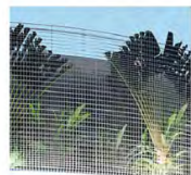
3 S.S. OR ALUMINUM SQUARE OPENING WIRE MESH PAINTED WHITE. OPENINGS 4"
