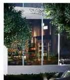
2 ALUMINUM-FRAMED STOREFRONT SYSTEM, W/ IMPACT-RESISTANT GLASS
