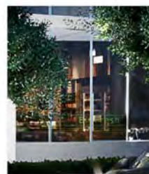
2 ALUMINUM-FRAMED STOREFRONT SYSTEM, W/ IMPCT-RESISTANT GLASS
