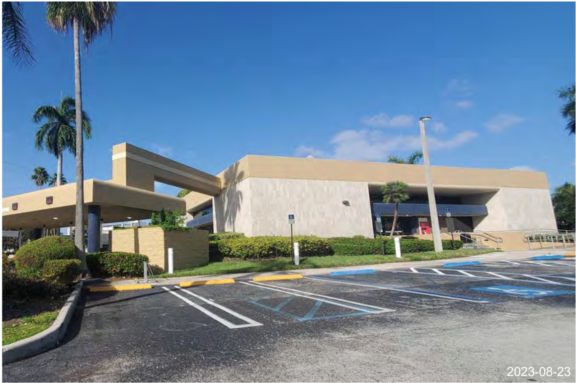
24. VIEW OF WELLS FARGO FROM EXISTING PARKING
