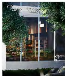
2 ALUMINUM-FRAMED STOREFRONT SYSTEM, W/ IMPCT-RESISTANT GLASS
