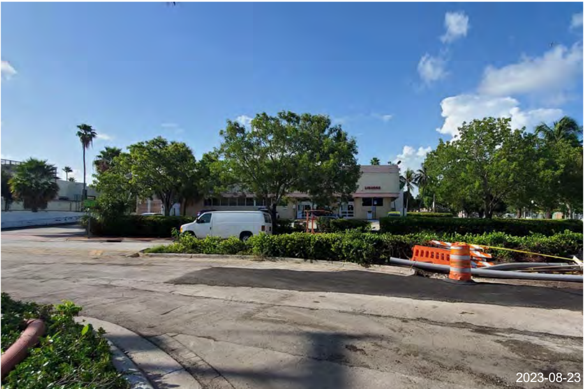
22. VIEW OF PARALLEL BUILDINGS FROM 19TH ST.
