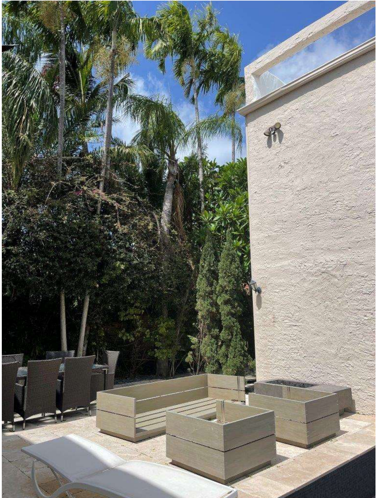
North Edge of Main House and Pool Deck (Area Where Variance is Requested)
