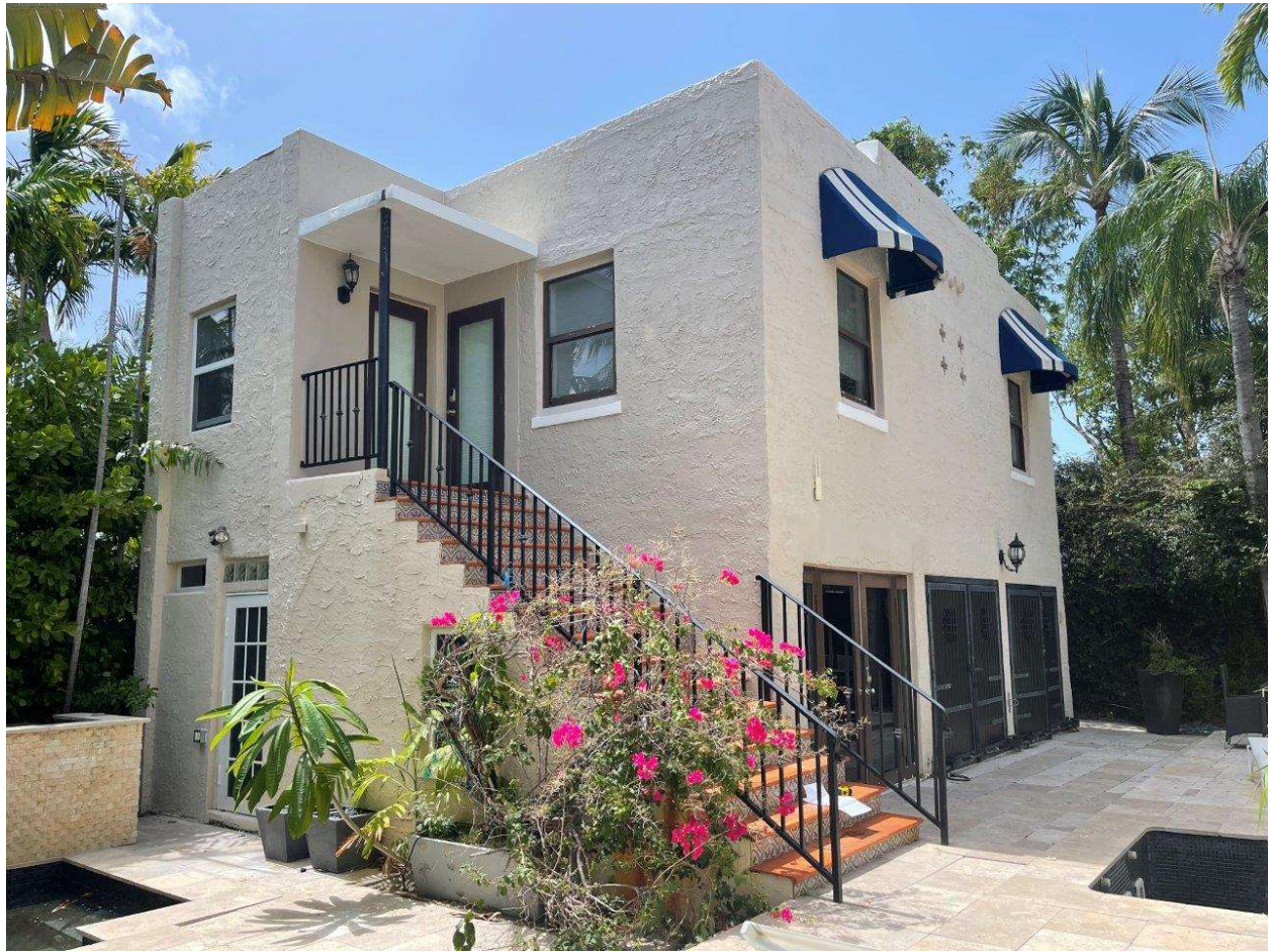
Guest House with 2 nd Floor Entrance Stair and Corner of Existing Pool
