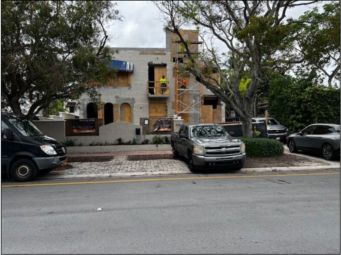
5768 Pine Tree Drive (Subject Residence)
