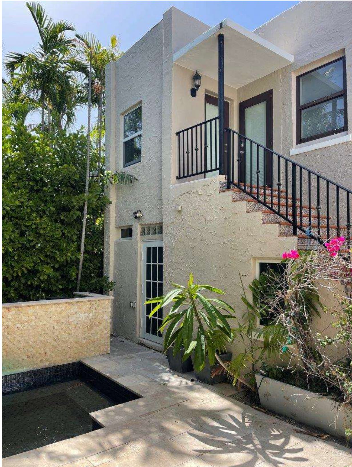
South Side of Guest House Showing Non-Conforming Spa in Rear Yard
