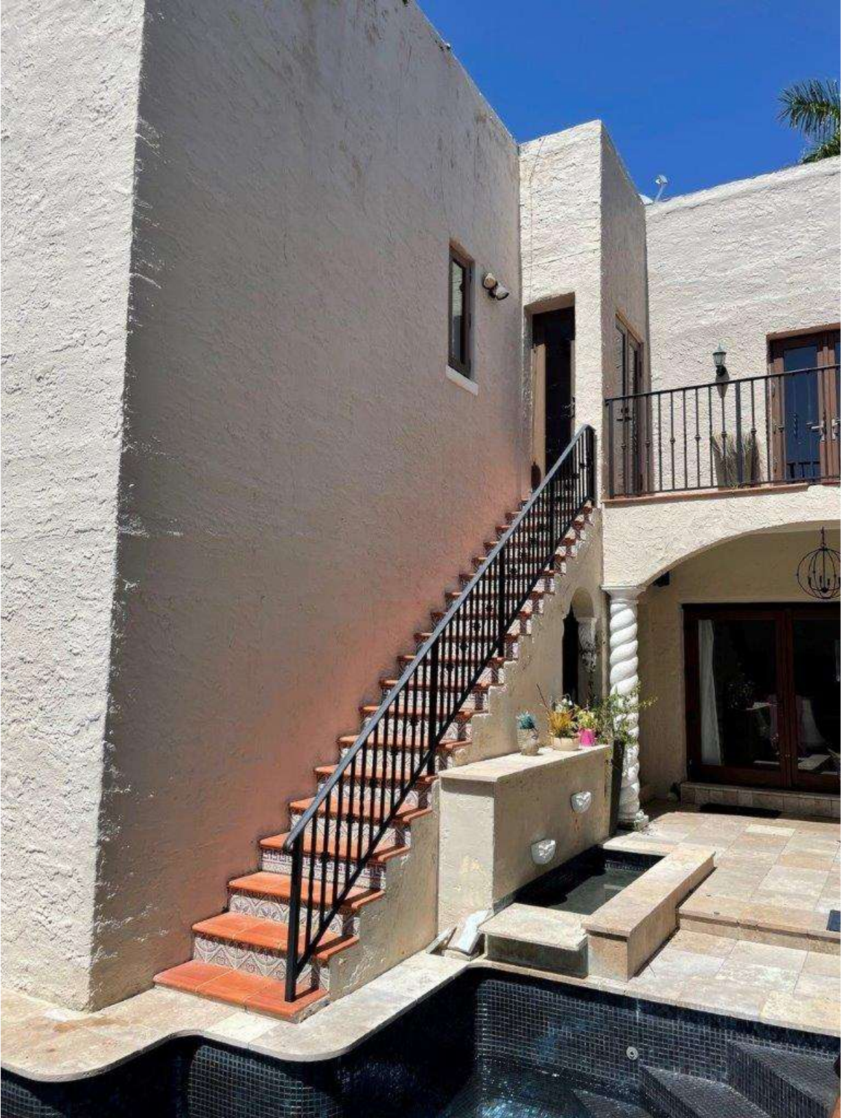
Existing Swimming Pool- Showing Proximity to House Wall
