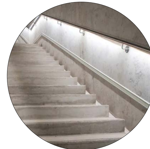
4 CONCRETE SMOOTH FINISH SEALED & FLAT PROFILE HANDRAIL
