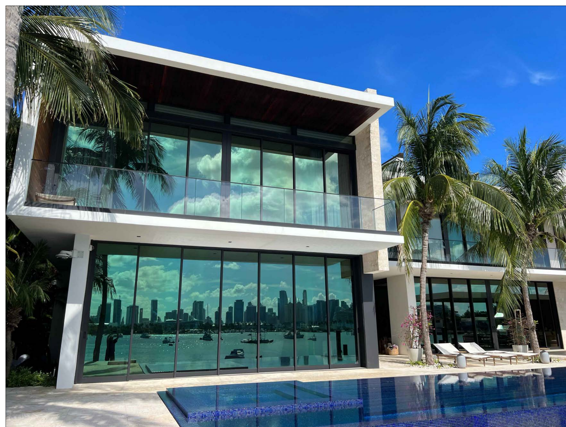
③ REAR LOOKING NORTH
