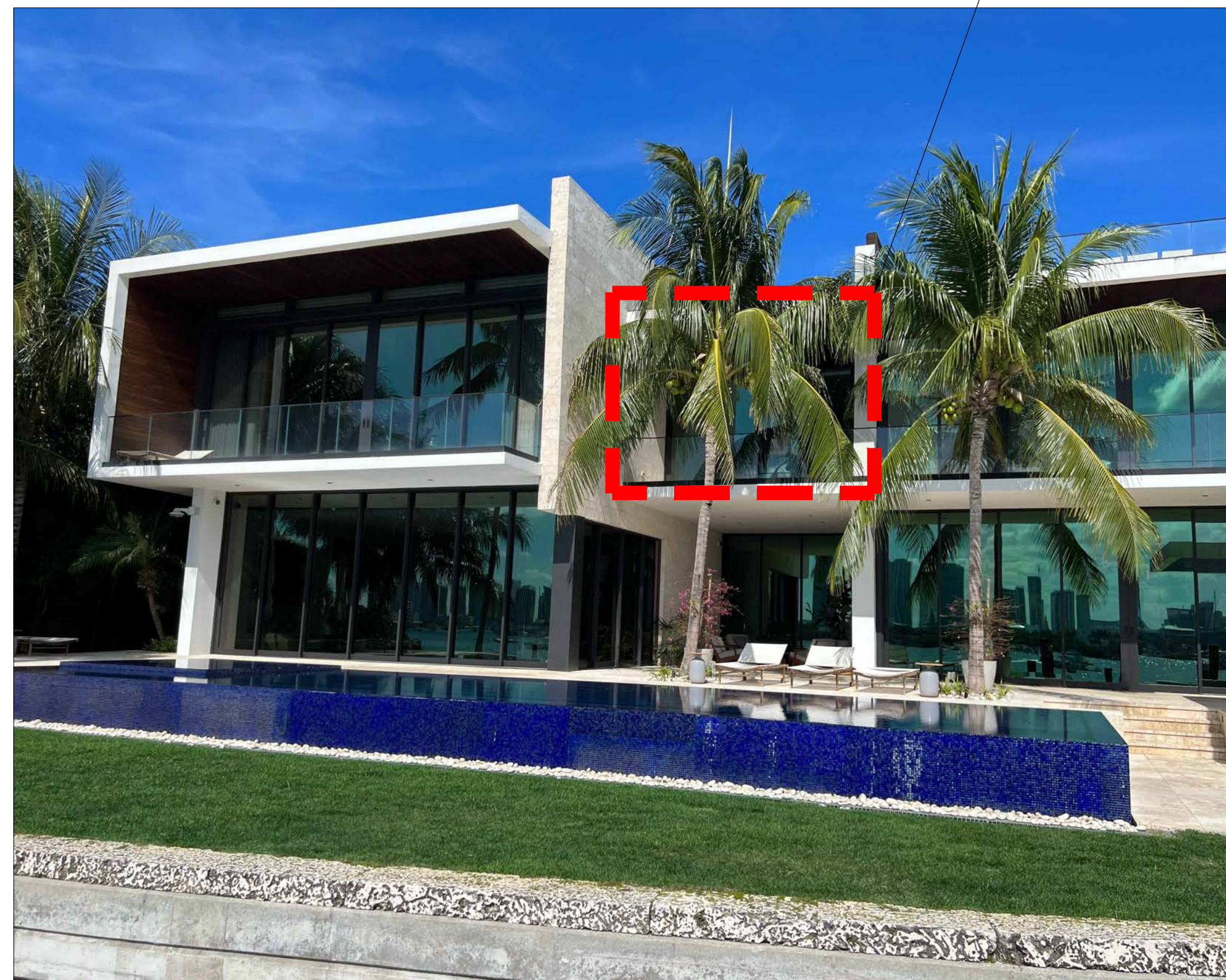
① REAR - LOOKING NORTH EXISTING
