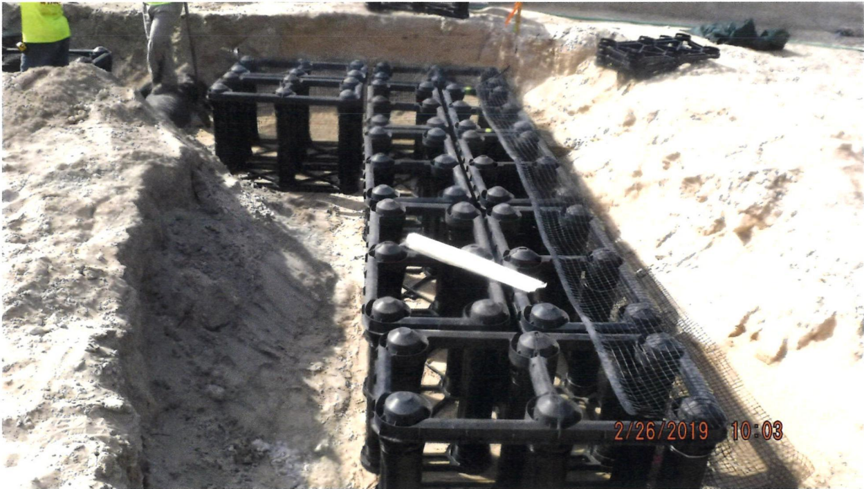
Suspended Pavement System Installation Progress Photo
