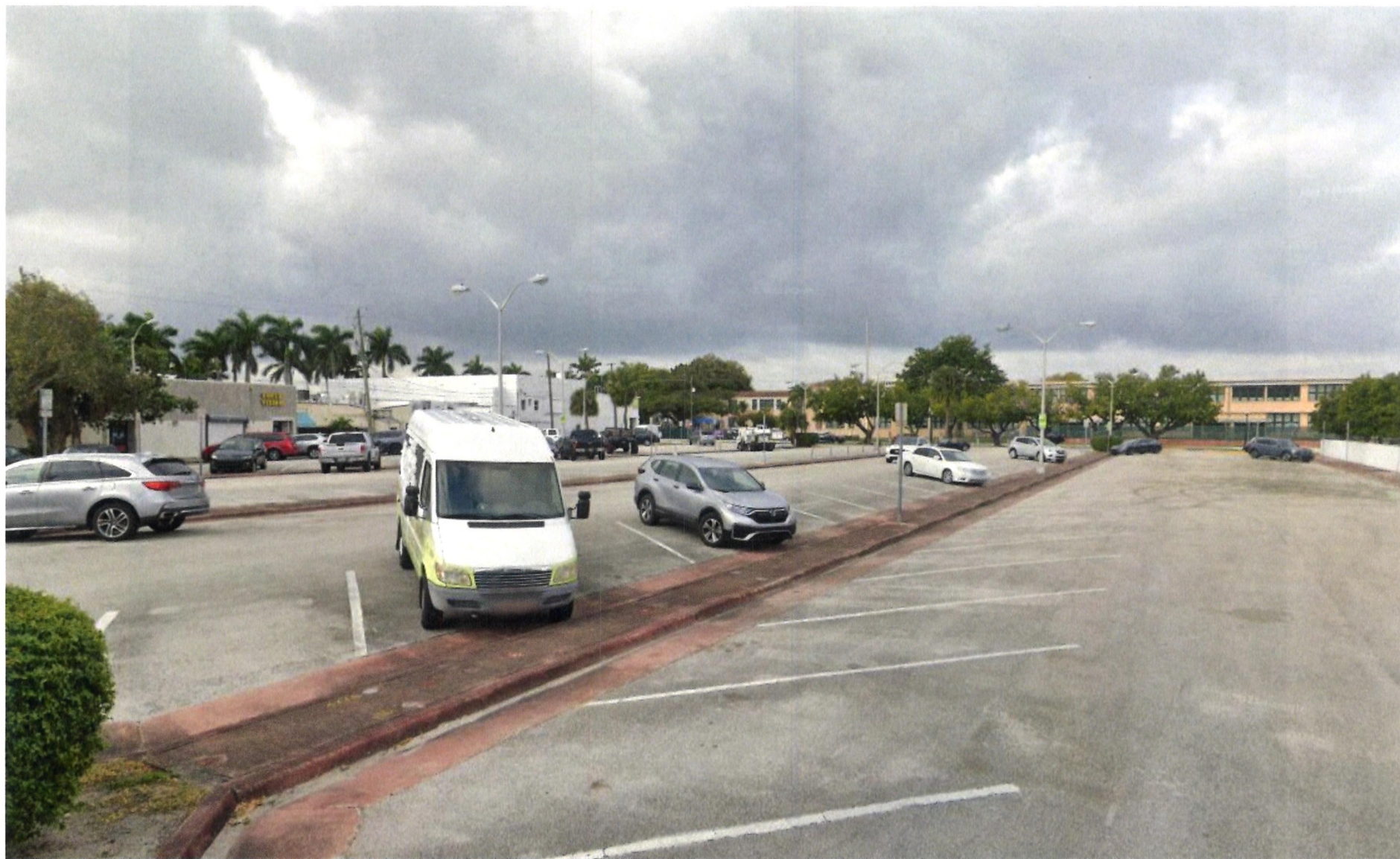
P-63 Existing Conditions
