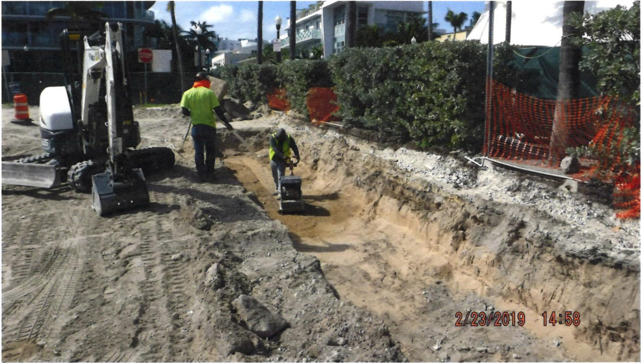
Suspended Pavement System Installation Progress Photo
