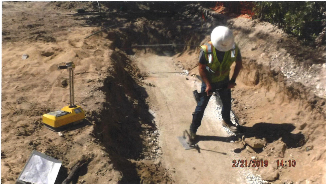
Suspended Pavement System Installation Progress Photo
