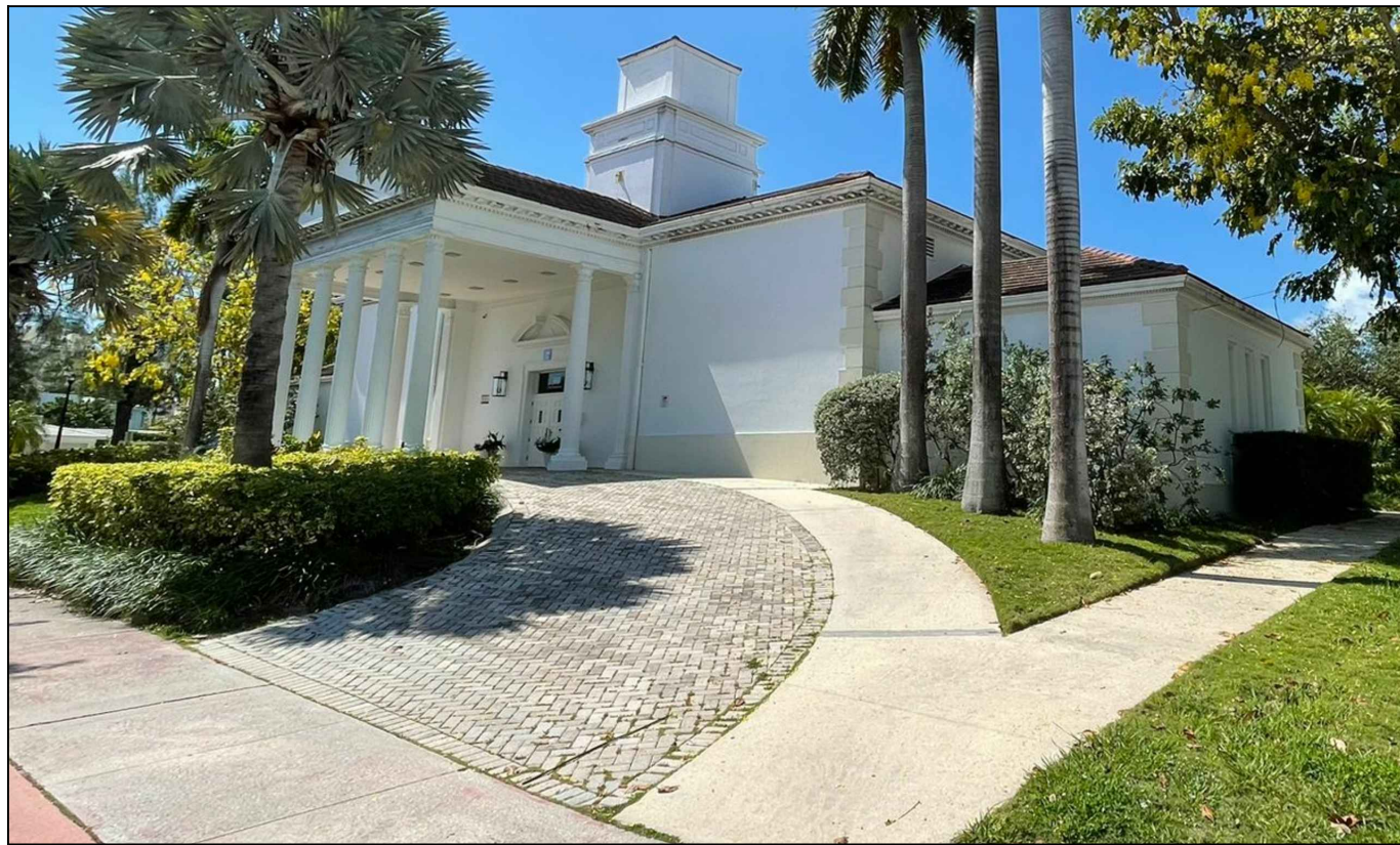
NORTHWEST (FRONT VIEW)
