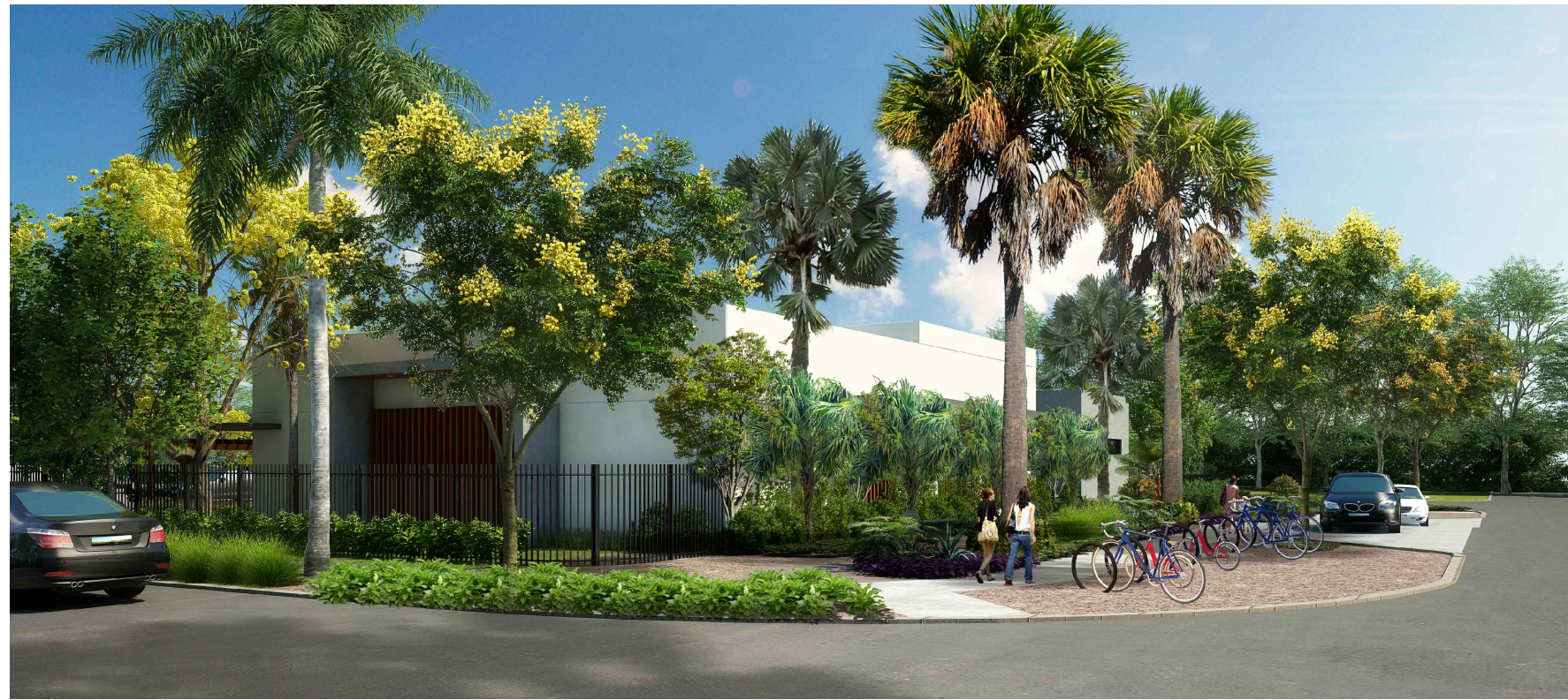
VIEW # 1 (40TH STREET & PINETREE DRIVE)
