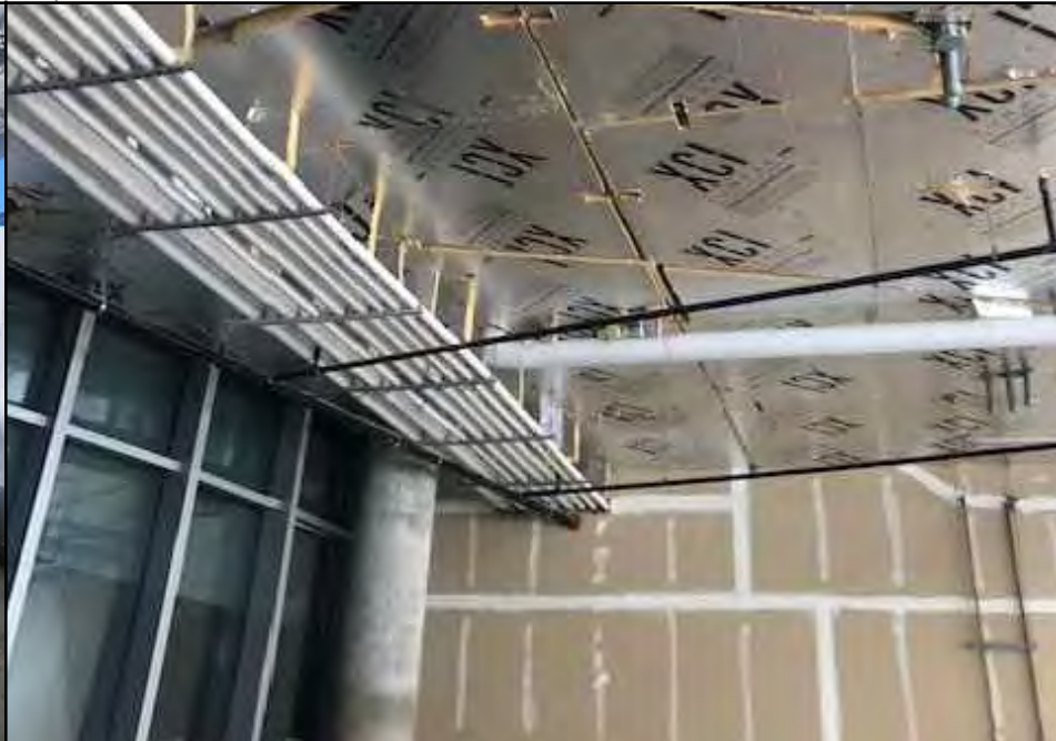
G INTERIOR - EXISTING CONDITIONS SCALE: NTS
