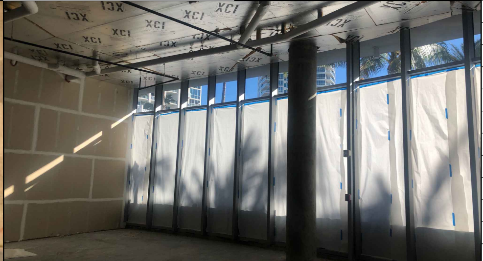
E INTERIOR - EXISTING CONDITIONS SCALE: NTS
