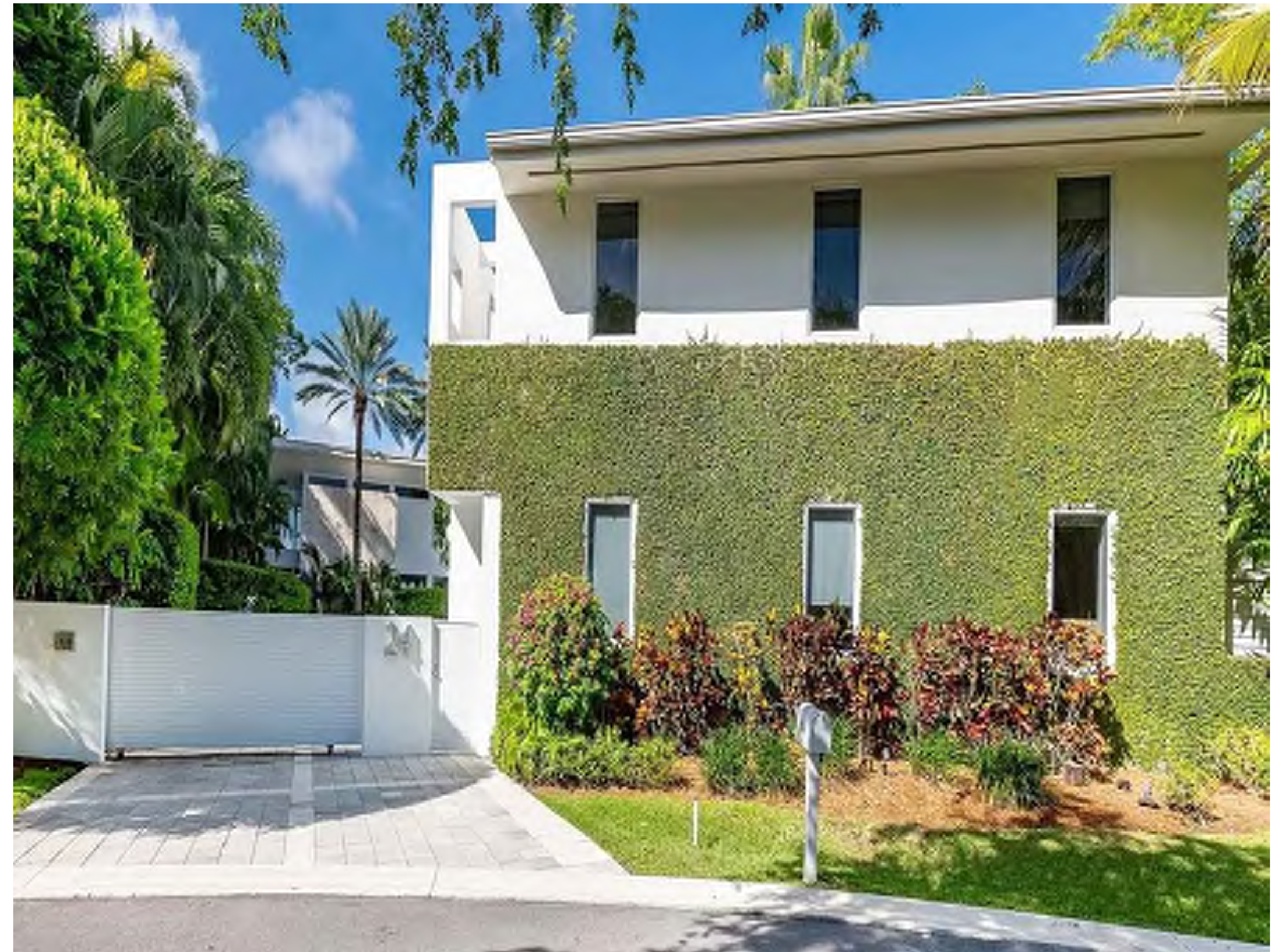
07 24 PALM AVENUE (5/23/2022) PRIOR TO CONSTRUCTION
