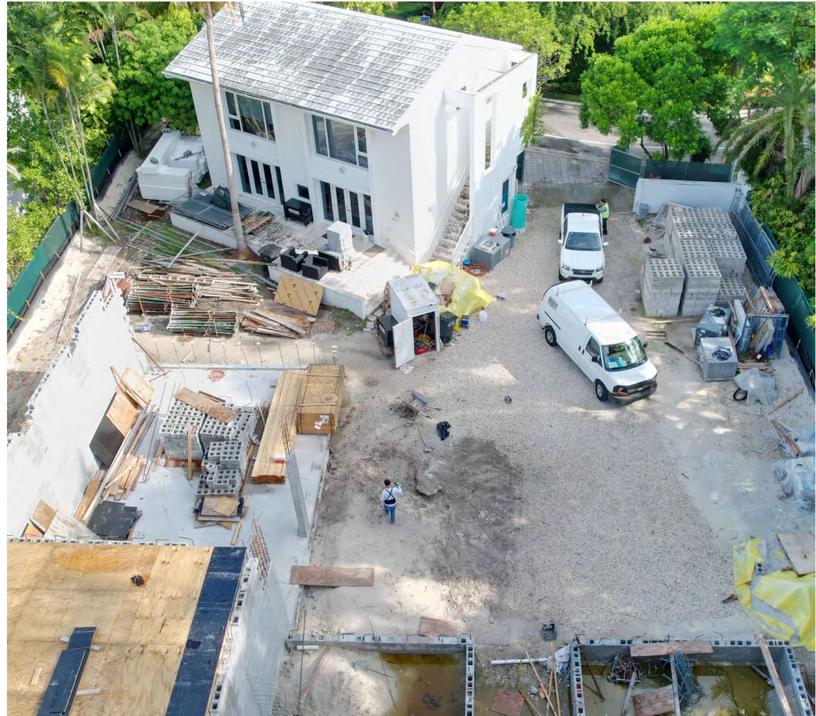
03 GUEST HOUSE - AERIAL SITE PHOTO (10/10/2023)
