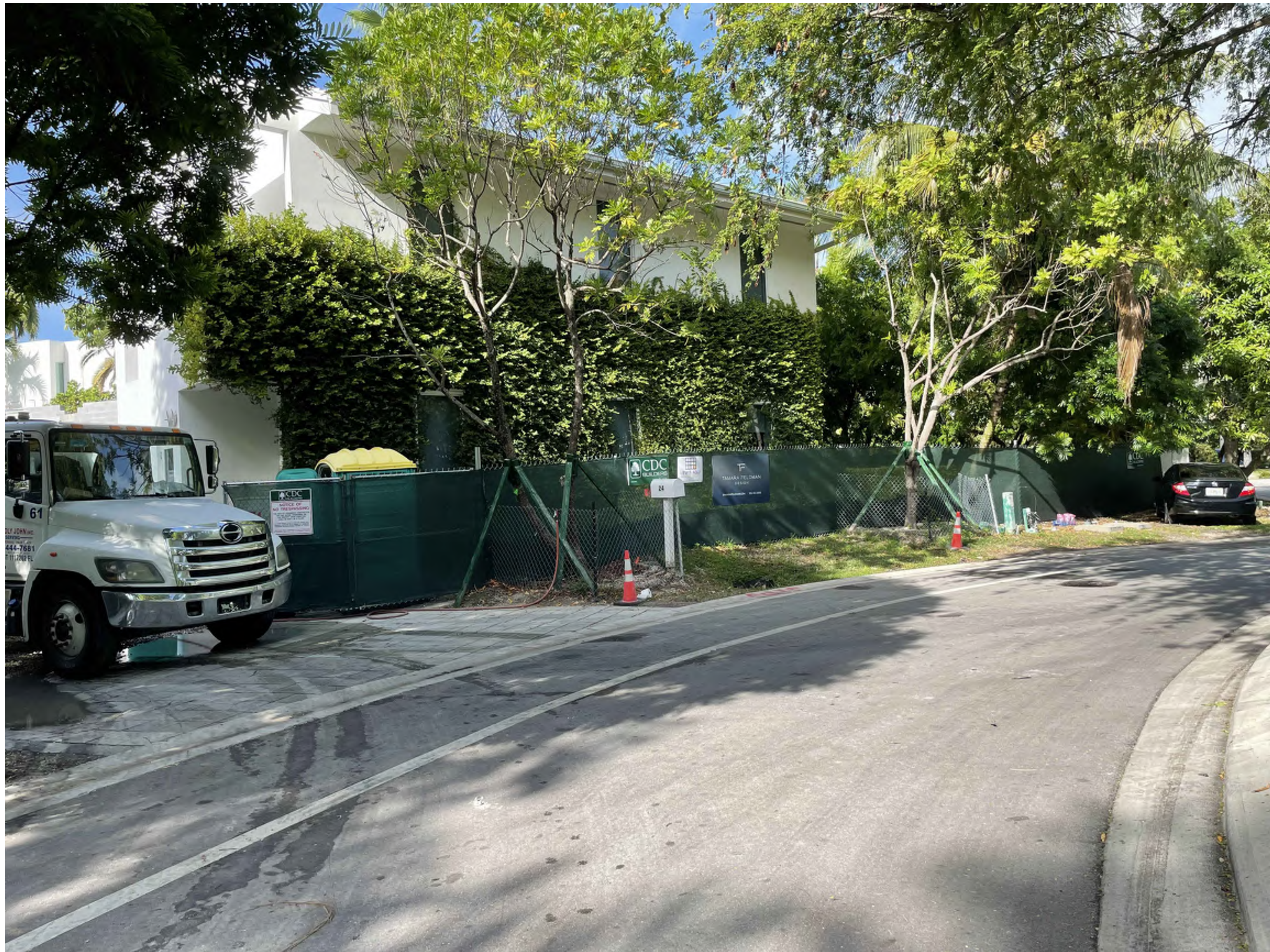
07 24 PALM AVENUE (11/3/2023) CURRENTLY UNDER CONSTRUCTION
