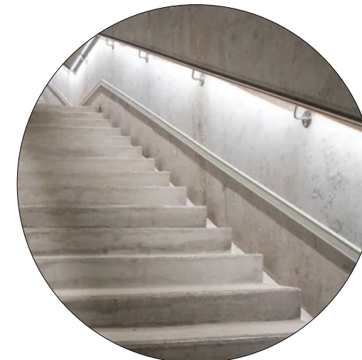
4 CONCRETE SMOOTH FINISH SEALED & FLAT PROFILE HANDRAIL
