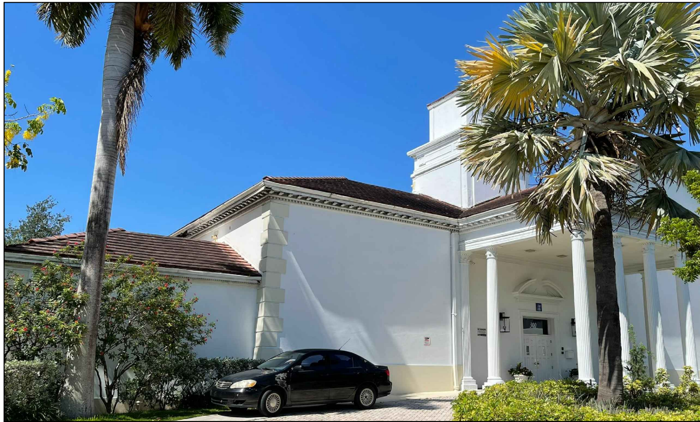
NORTHEAST (FRONT VIEW)
