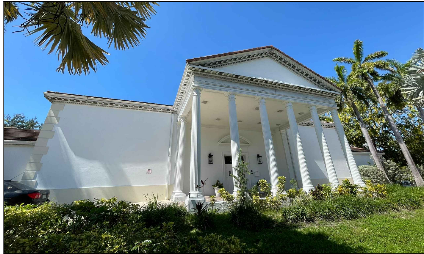
NORTH (FRONT VIEW)
