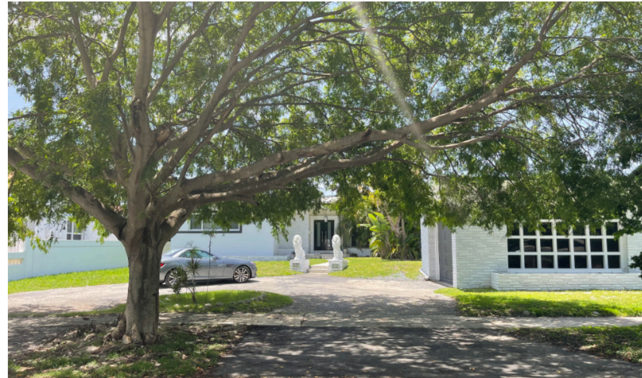
2 1820 DAYTONIA DRIVE EXISTING ONE-STORY RESIDENCE
