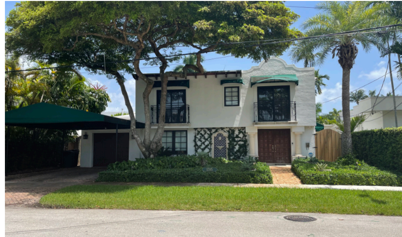
10 1785 DAYTONIA DRIVE EXISTING TWO-STORY RESIDENCE
