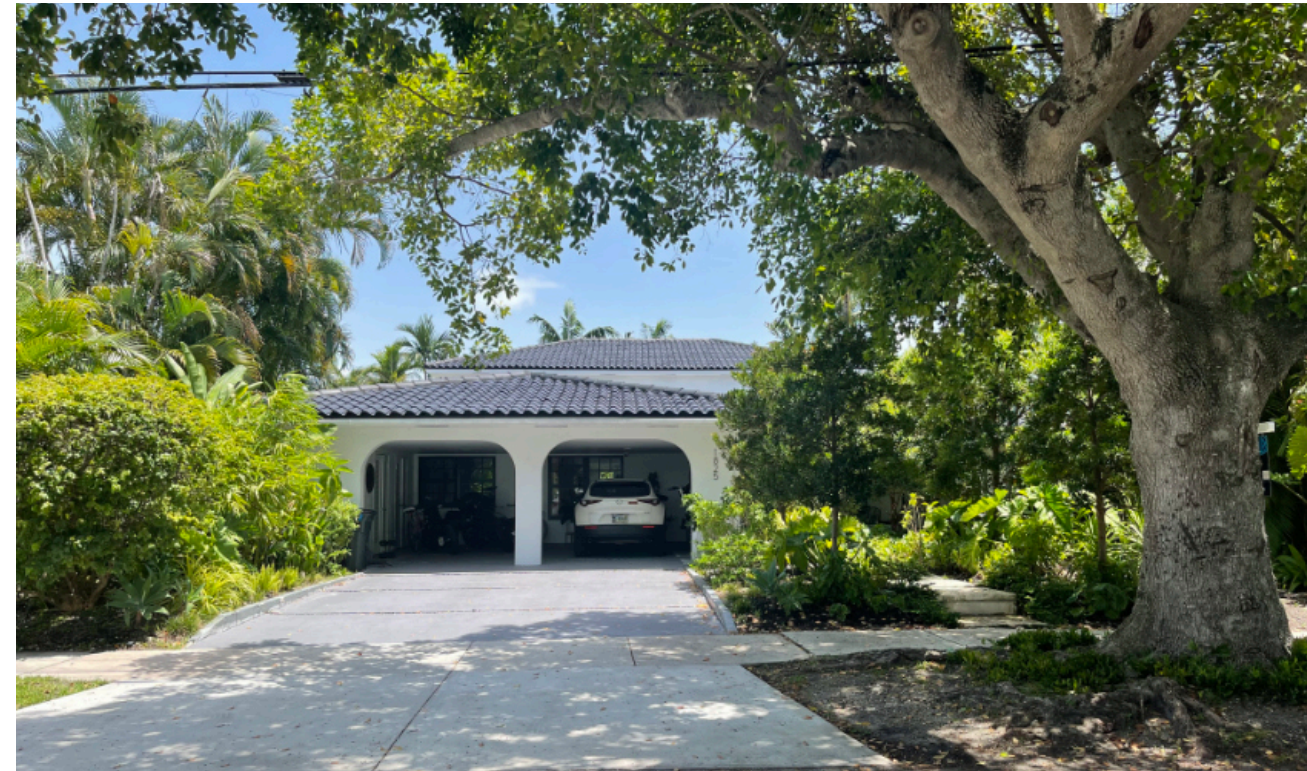
6 1825 DAYTONIA DRIVE EXISTING TWO-STORY RESIDENCE
