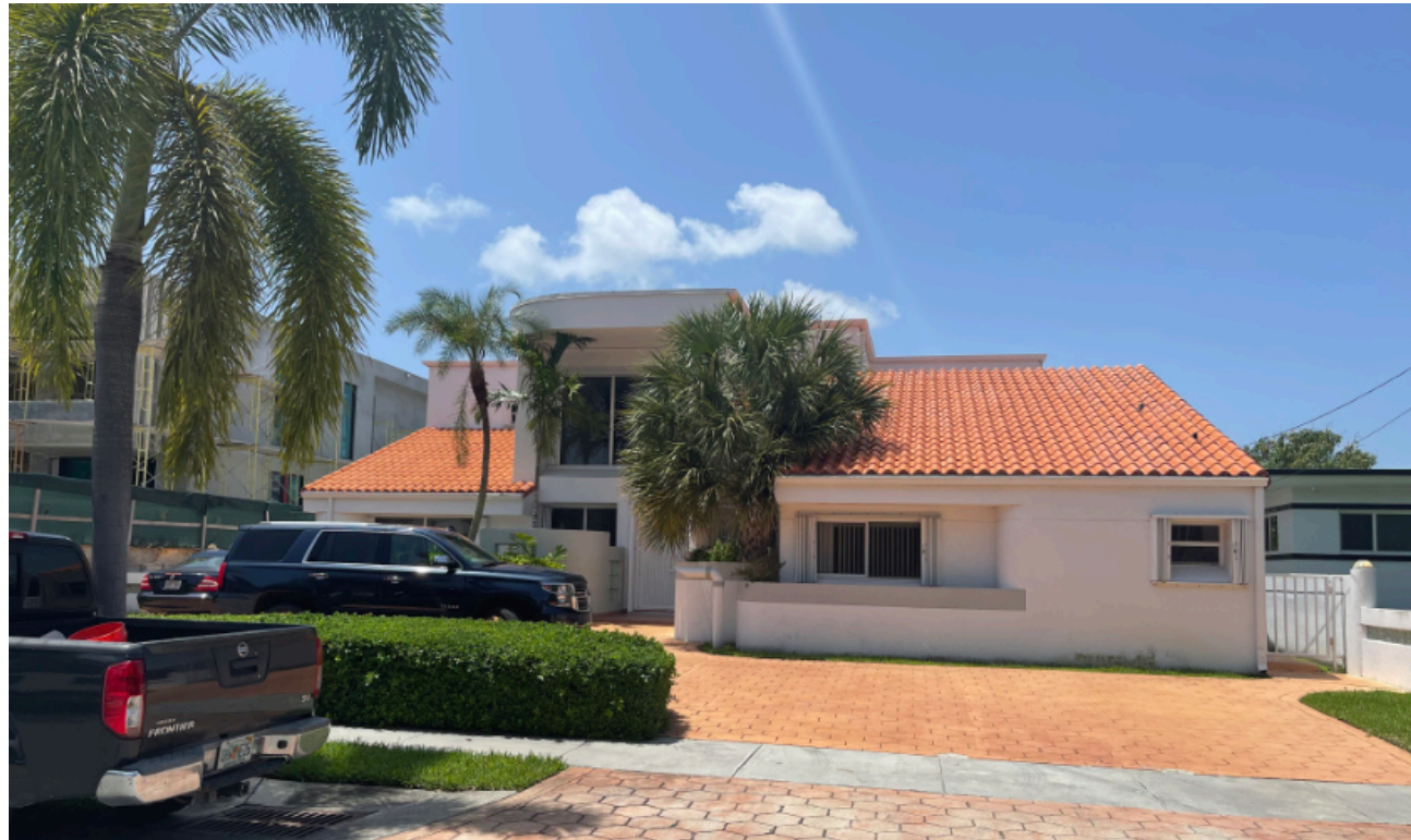
1 1810 DAYTONIA DRIVE EXISTING TWO-STORY RESIDENCE
