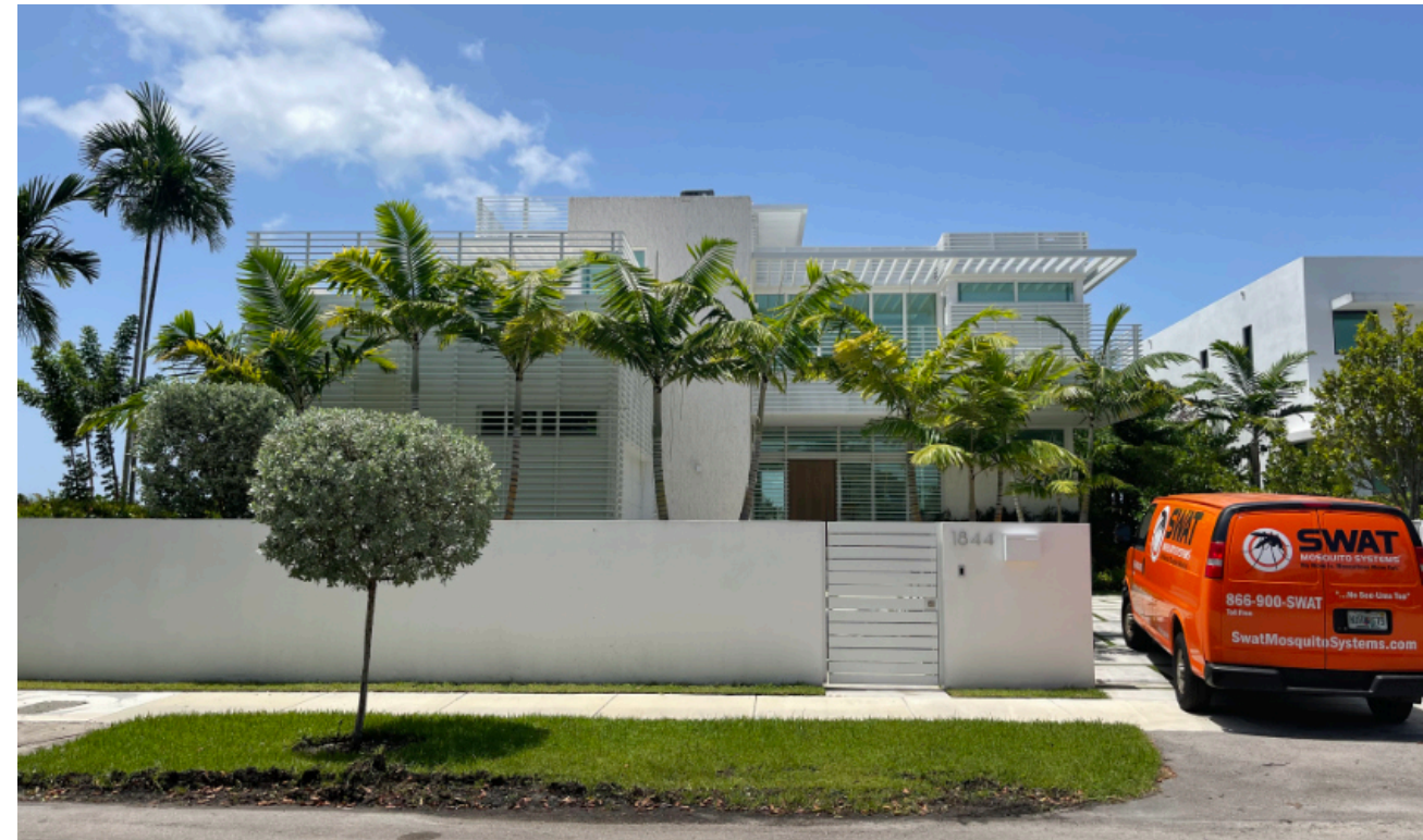
4 1844 DAYTONIA DRIVE EXISTING TWO-STORY RESIDENCE
