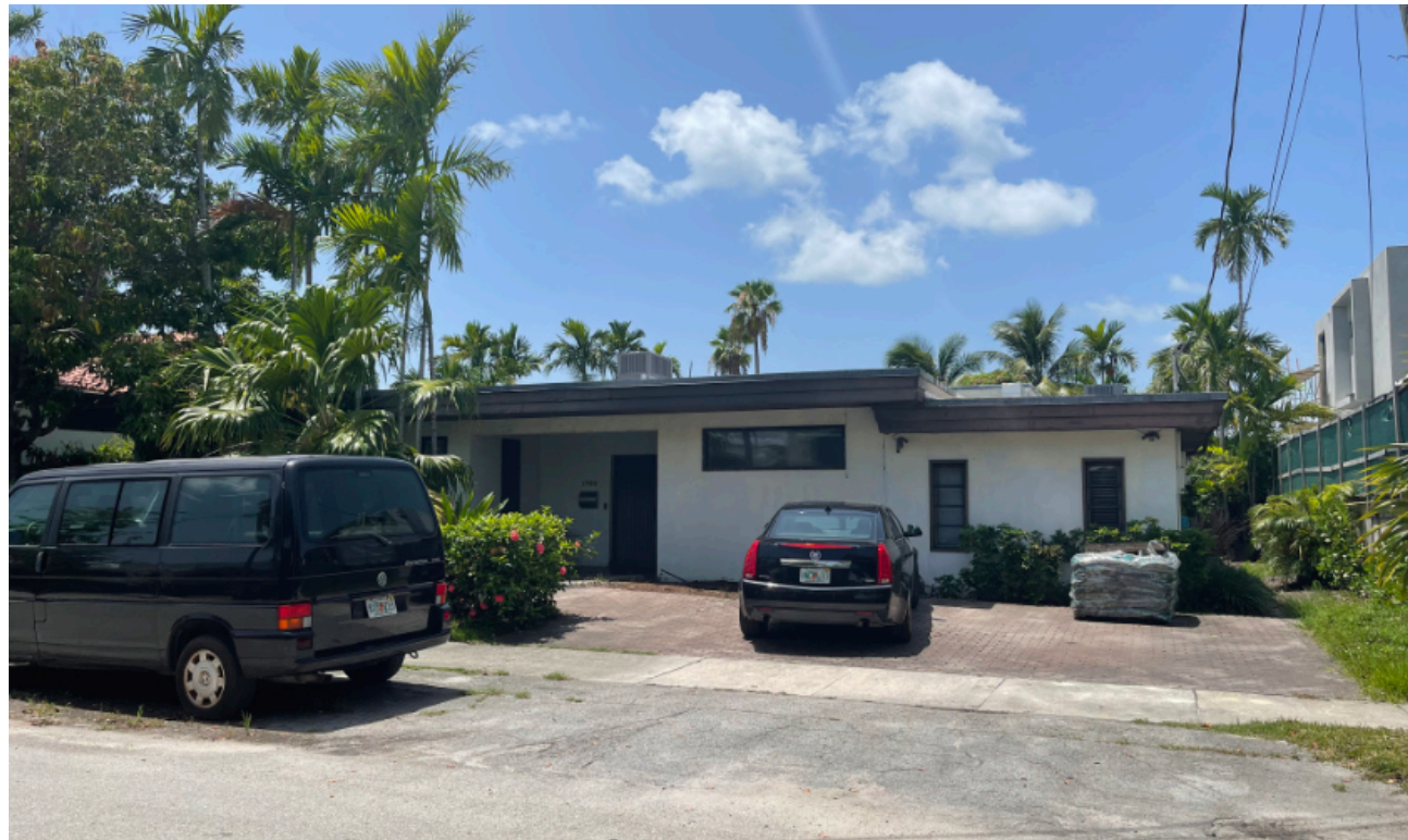
11 1780 DAYTONIA DRIVE EXISTING ONE-STORY RESIDENCE
