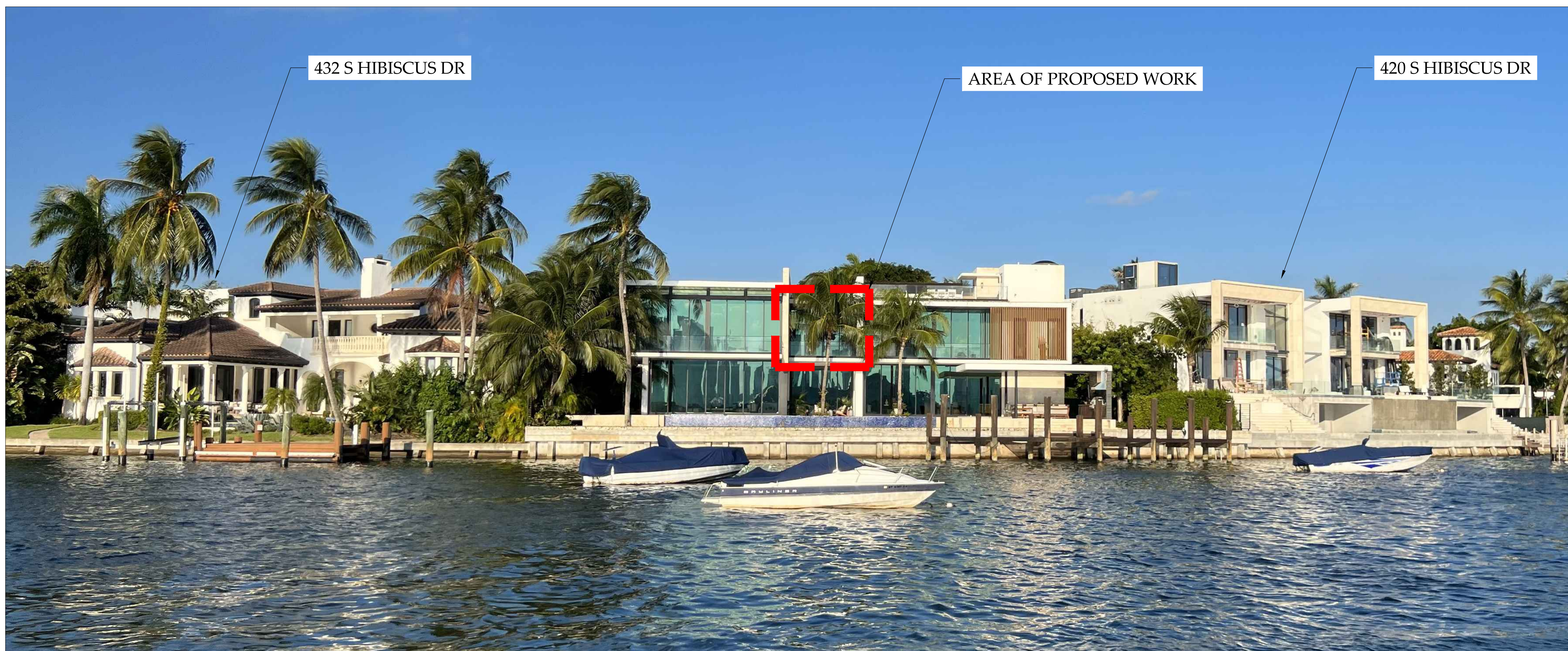
① REAR - LOOKING NORTH EXISTING
