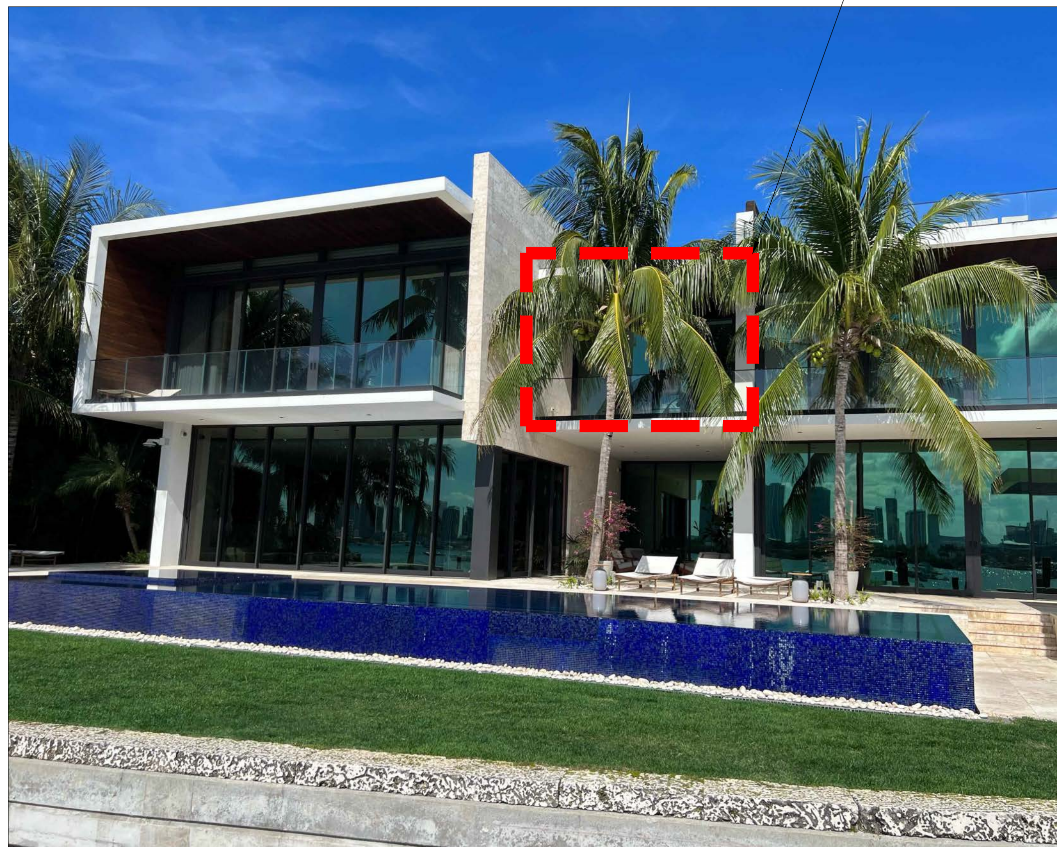
① REAR - LOOKING NORTH EXISTING
