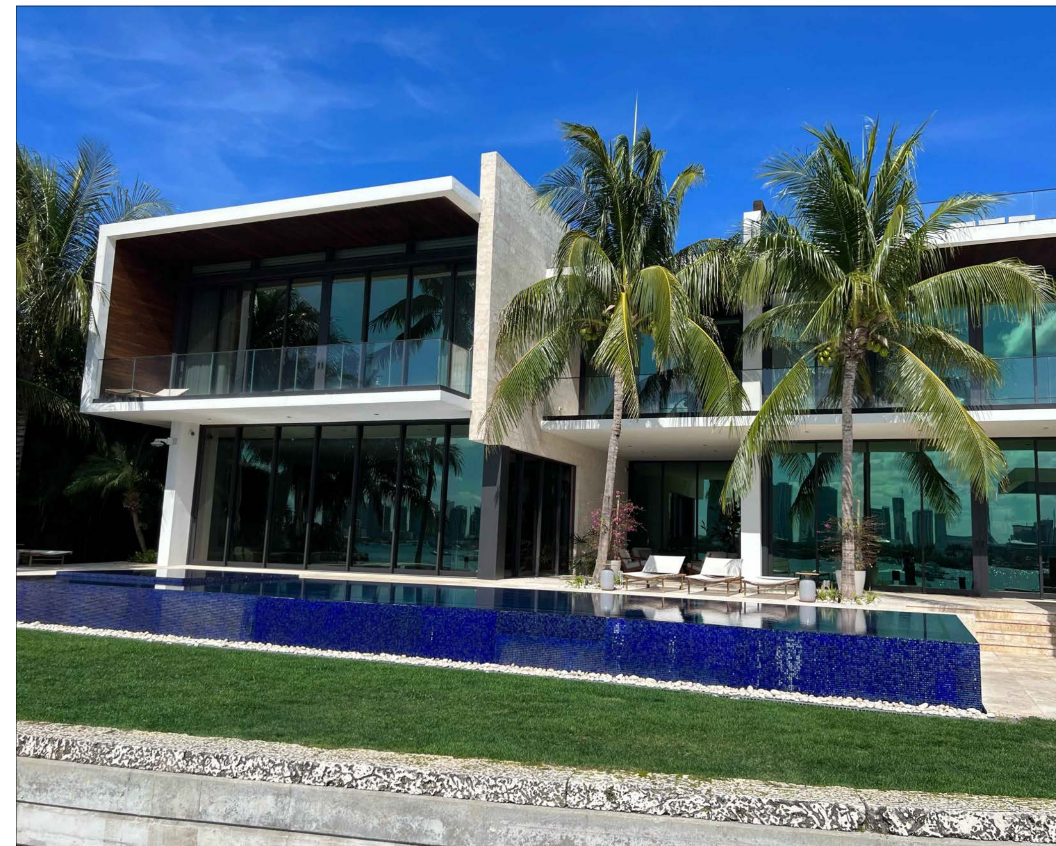
④ REAR - LOOKING NORTH
