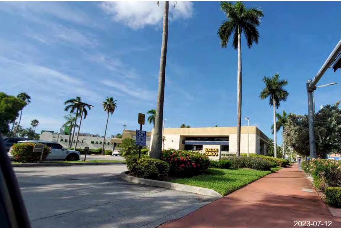
2. VIEW OF SITE FROM NORTH PEDESTRIAN WALKWAY
