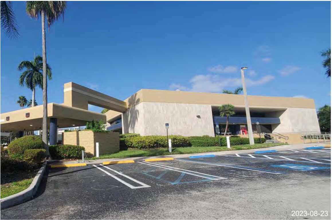
24. VIEW OF WELLS FARGO FROM EXISTING PARKING
