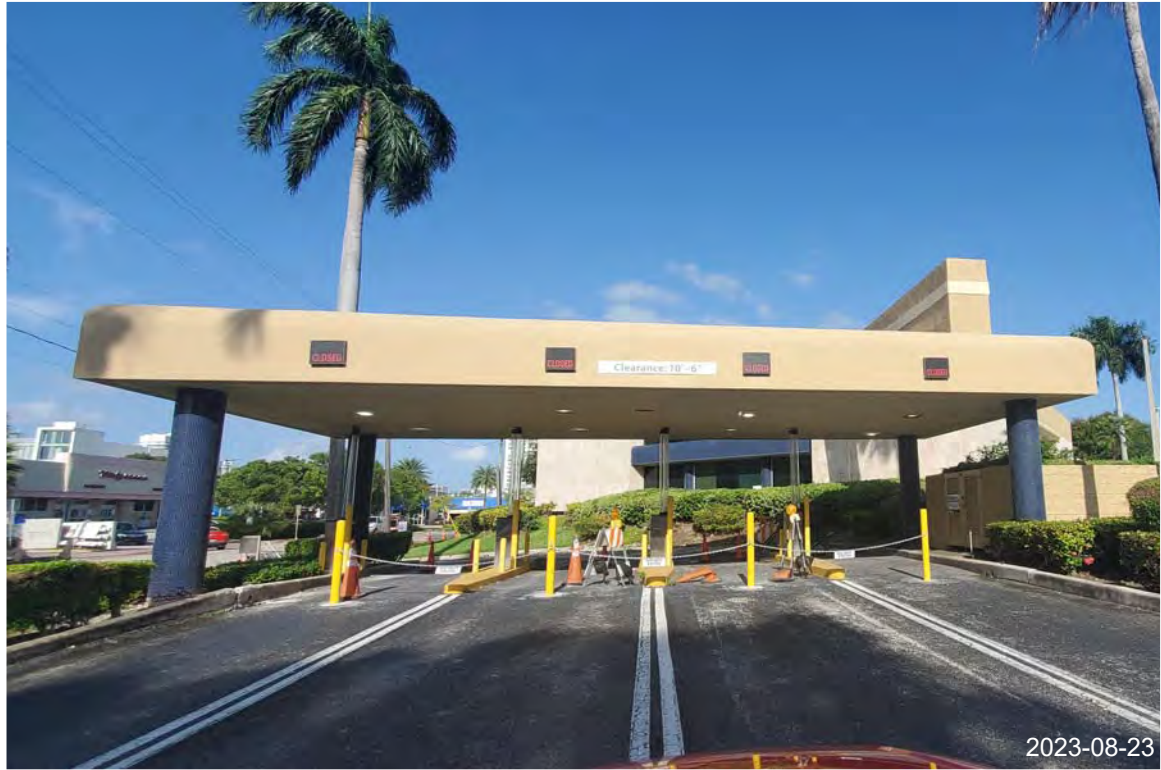
23.EXISTING DRIVE THRU BANK ON SITE
