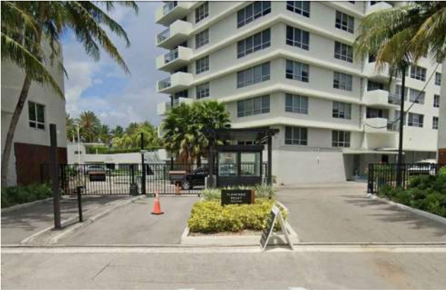
25 1508 BAY ROAD (FLAMINGO POINT SOUTH TOWER ENTRANCE)
