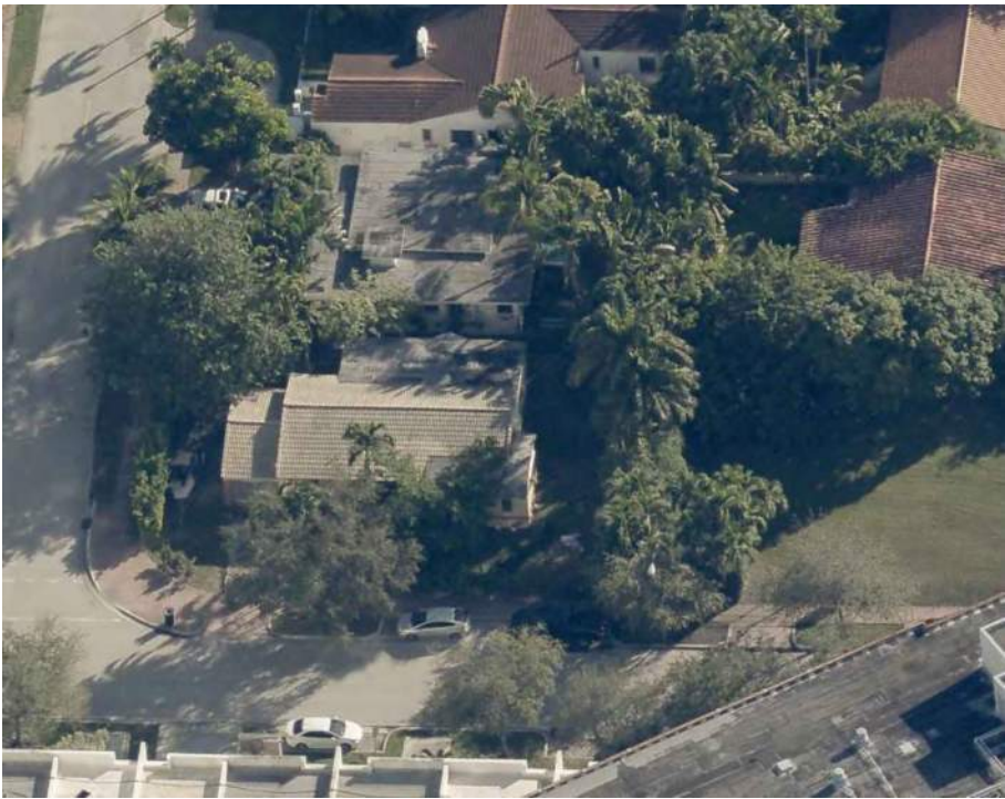
2 1435 BAY ROAD-1340 FLAMINGO WAY (VIEW FROM BAY ROAD)
