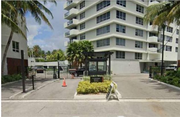
25 1508 BAY ROAD (FLAMINGO POINT SOUTH TOWER ENTRANCE)
