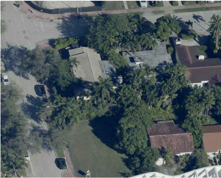
1 1435 BAY ROAD-1340 FLAMINGO WAY (VIEW FROM 14TH TERRACE)
