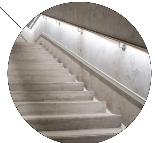
CONCRETE SMOOTH FINISH SEALED & FLAT PROFILE HANDRAIL
