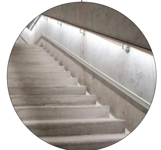
CONCRETE SMOOTH FINISH SEALED
