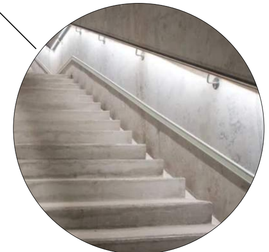
CONCRETE SMOOTH FINISH SEALED & FLAT PROFILE HANDRAIL
