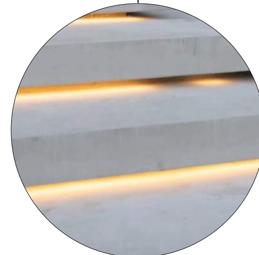
CONCRETE STAIR UNDERSIDE LIT
