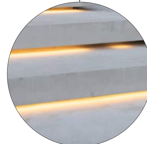
CONCRETE STAIR UNDERSIDE LIT
