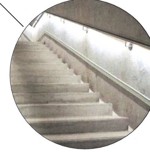
CONCRETE SMOOTH FINISH SEALED & FLAT PROFILE HANDRAIL
