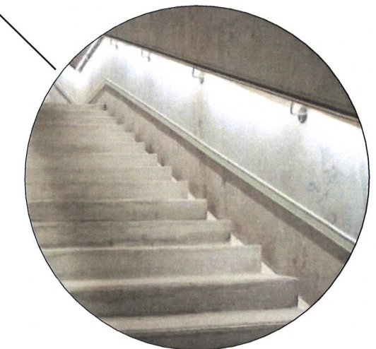
CONCRETE SMOOTH FINISH SEALED & FLAT PROFILE HANDRAIL
