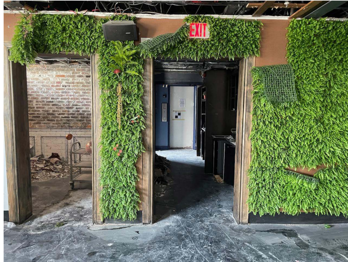
② CORRIDOR ACCESS - EXISTING CONDITIONS - GROUND FLOOR LEVEL
