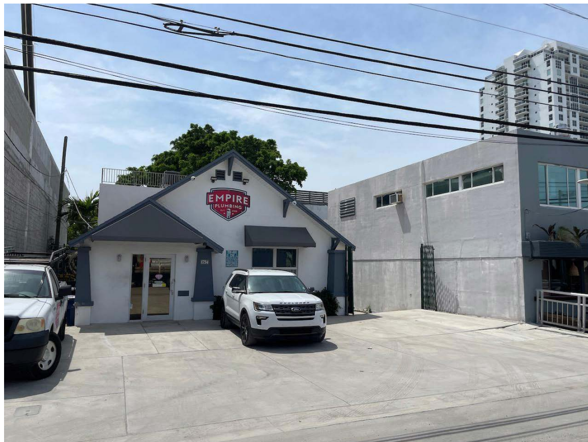
⑥ ADJACENT BUILDING EAST FACADE
