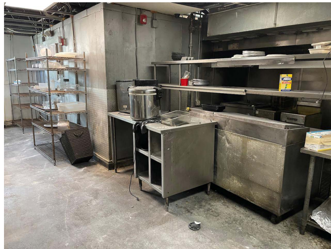
③ KITCHEN - EXISTING CONDITIONS - SECOND FLOOR LEVEL
