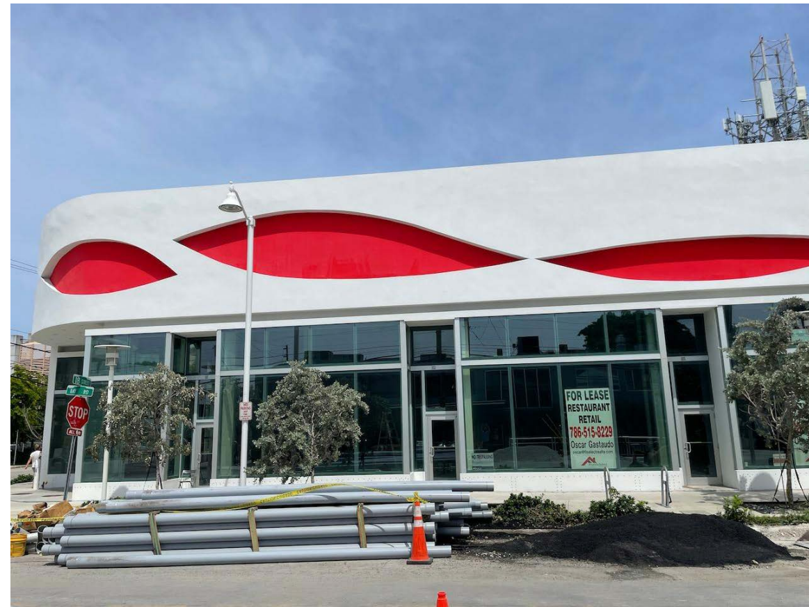
⑤ FRONT BUILDING AT EAST FACADE
