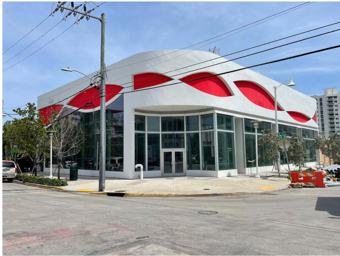
④ SHOOPING BUILDING CORNER AT EAST FACADE
