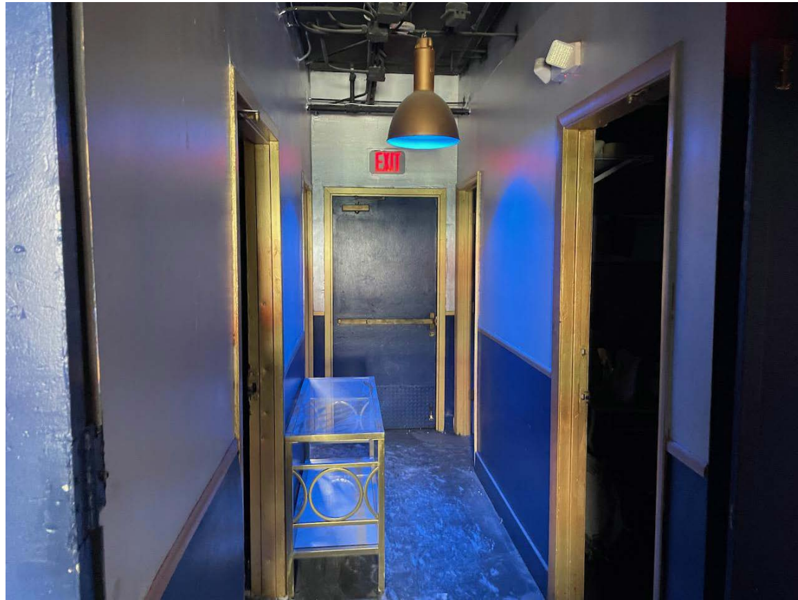
① BATHROOM HALLWAY - EXISTING CONDITIONS - SECOND FLOOR LEVEL
