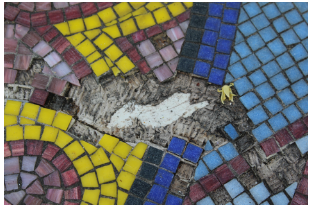
Detail of the bedding mortar and underlying fiberglass and mesh.
