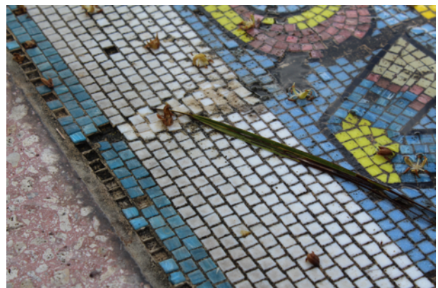
Detail of tile loss, standing water, dirt, and debris sitting on the mosaic
