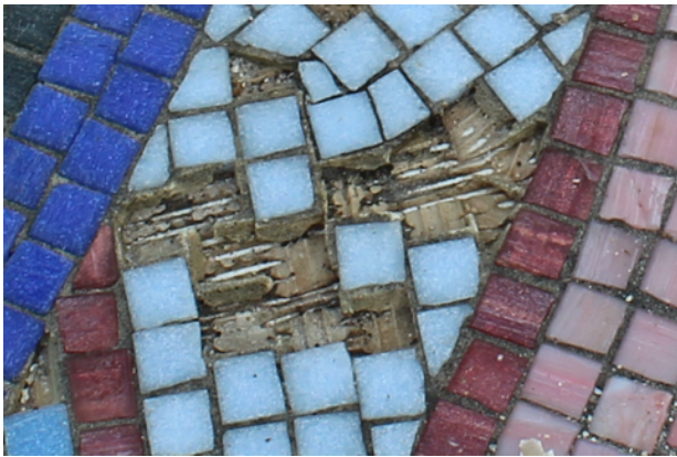
Detail of visible fiberglass mesh
