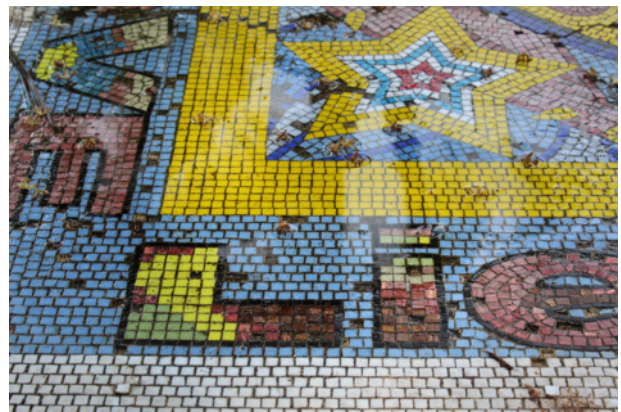
Detail of pooling water with visible algae on the grout and in areas where tiles have been displaced.
