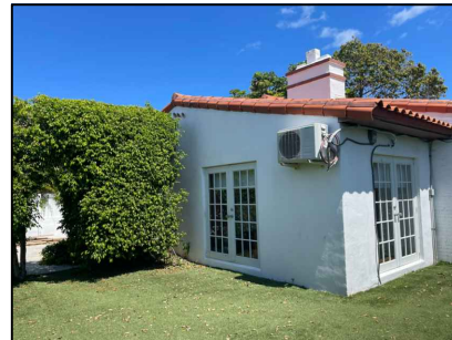
WEST (EXISTING HOUSE) (LEFT SIDE)
