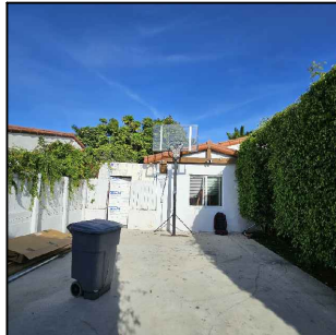
WEST (EXISTING HOUSE) (LEFT SIDE)
