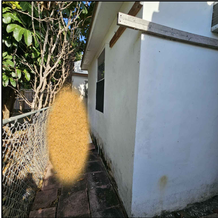
NORTH (LAUNDRY ROOM ADDITION) (REAR SIDE)
