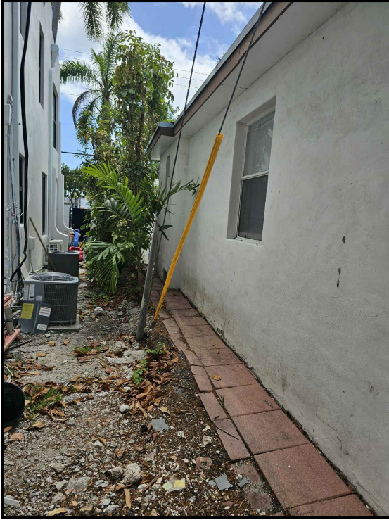
EAST (BEDROOM ADDITION) (RIGHT SIDE)
