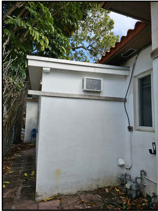
WEST (LAUNDRY ROOM ADDITION) (LEFT SIDE)
