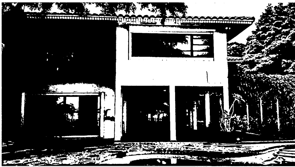
BUILDING REAR VIEW PHOTO TAKEN (06-17-2015)
