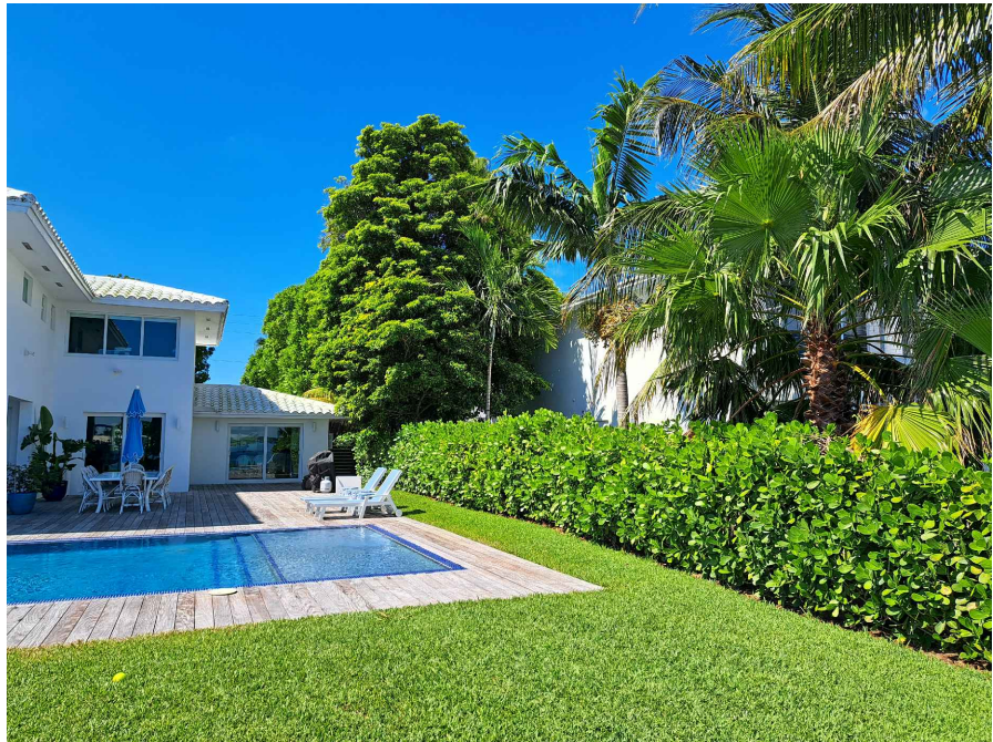
03 North Elevation (Rear View)
