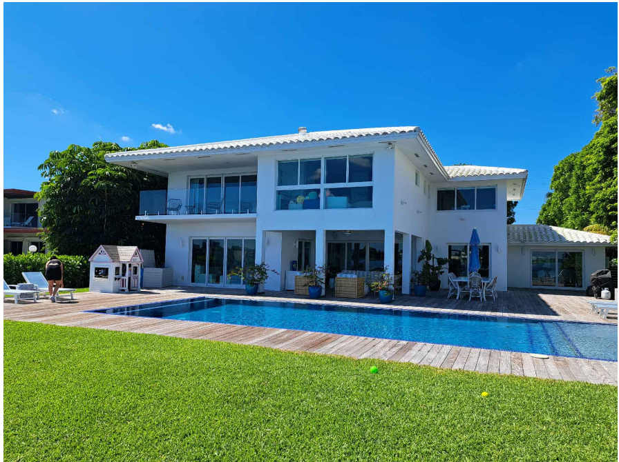
04 North Elevation (Rear View)
