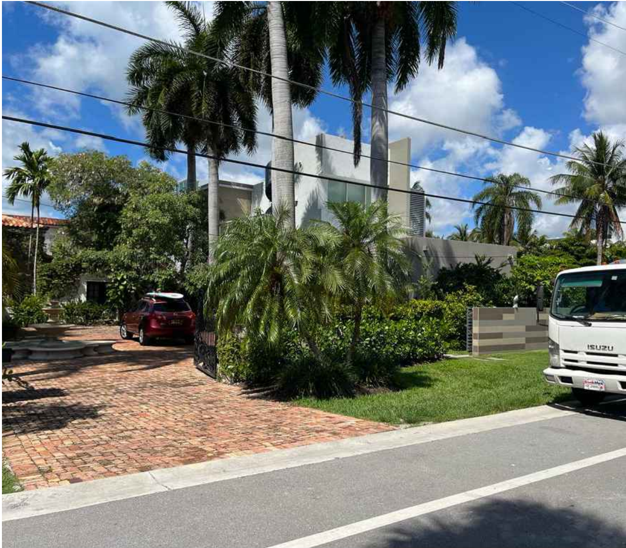
EXISTING HOUSE VIEW B
