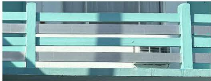
EXTERIOR BALCONY EXISTING PHOTO
