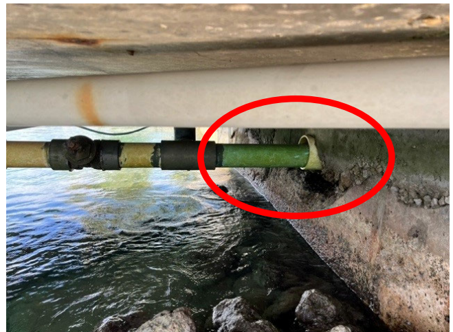
Opening in Seawall
