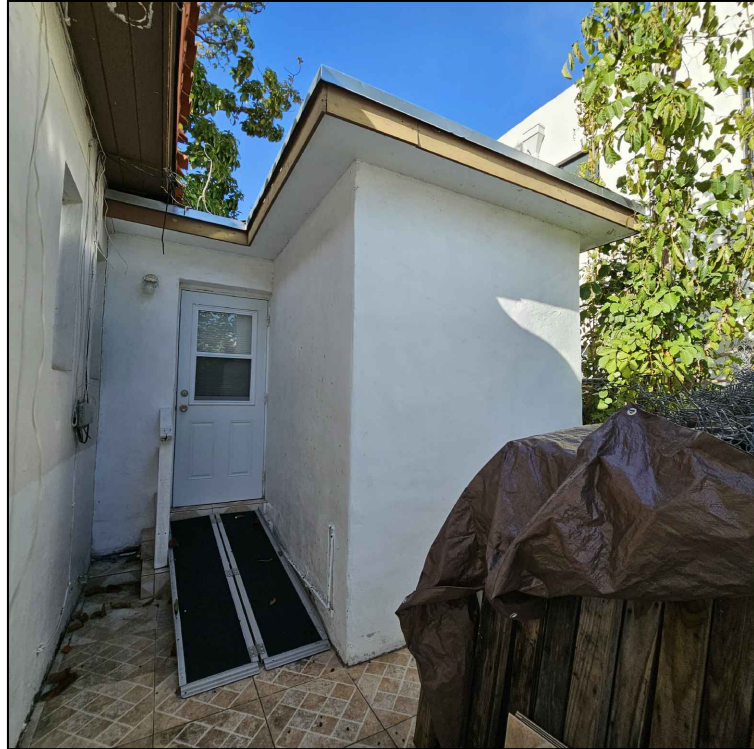
SOUTH (BEDROOM ADDITION) (FRONT SIDE)
