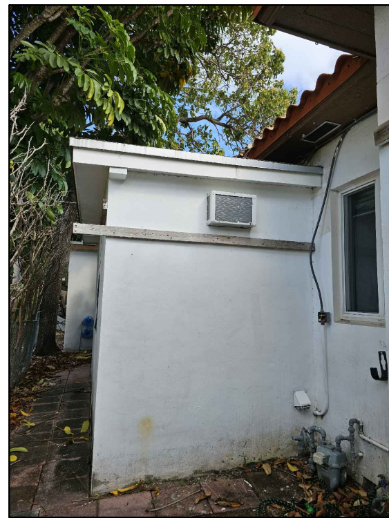
WEST (LAUNDRY ROOM ADDITION) (LEFT SIDE)
