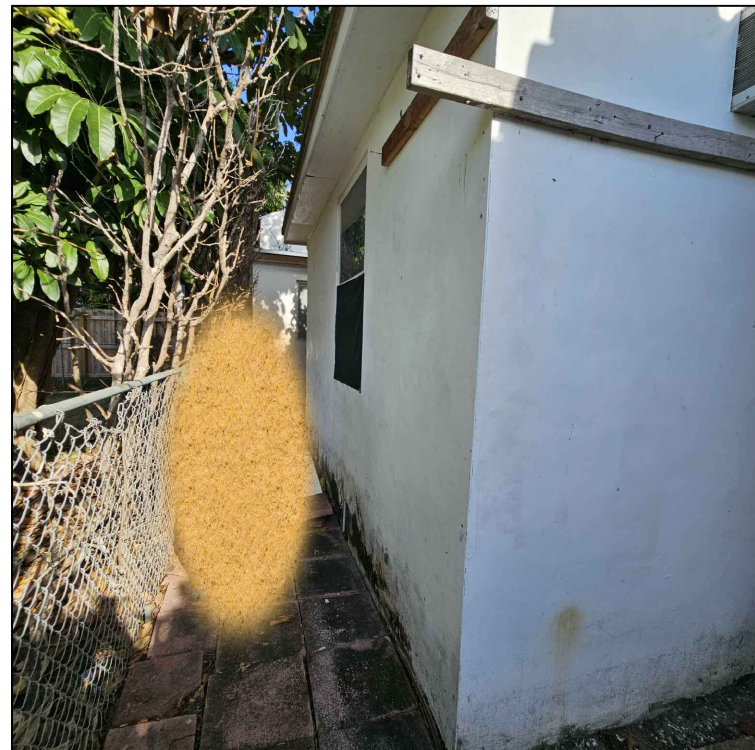
NORTH (LAUNDRY ROOM ADDITION) (REAR SIDE)
