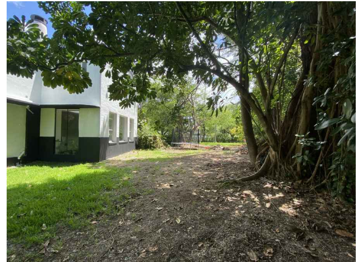
EXISTING HOUSE - LOT 2
