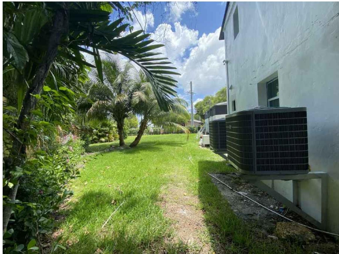
EXISTING HOUSE - LOT 2
