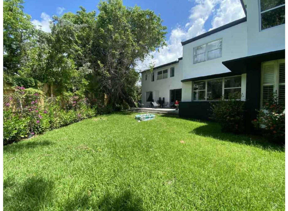
EXISTING HOUSE - LOT 2
