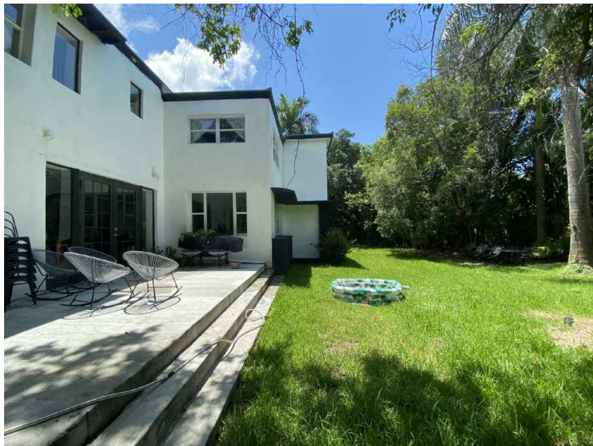
EXISTING HOUSE - LOT 2
