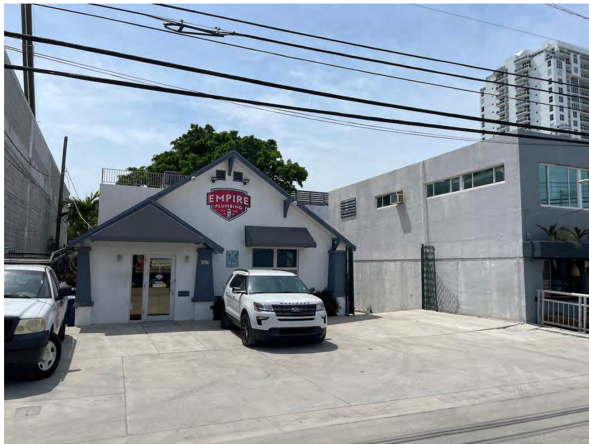
⑥ ADJACENT BUILDING EAST FACADE
