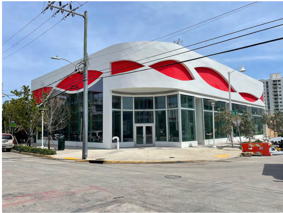
④ SHOOPING BUILDING CORNER AT EAST FACADE
