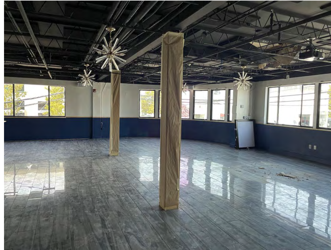
② LOUNGE DINING - EXISTING CONDITIONS - SECOND FLOOR LEVEL
