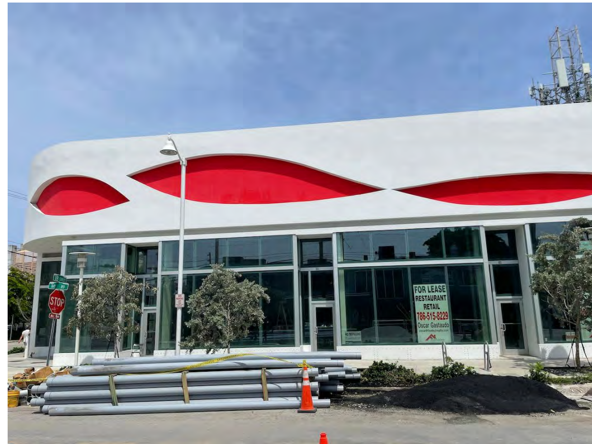
⑤ FRONT BUILDING AT EAST FACADE
