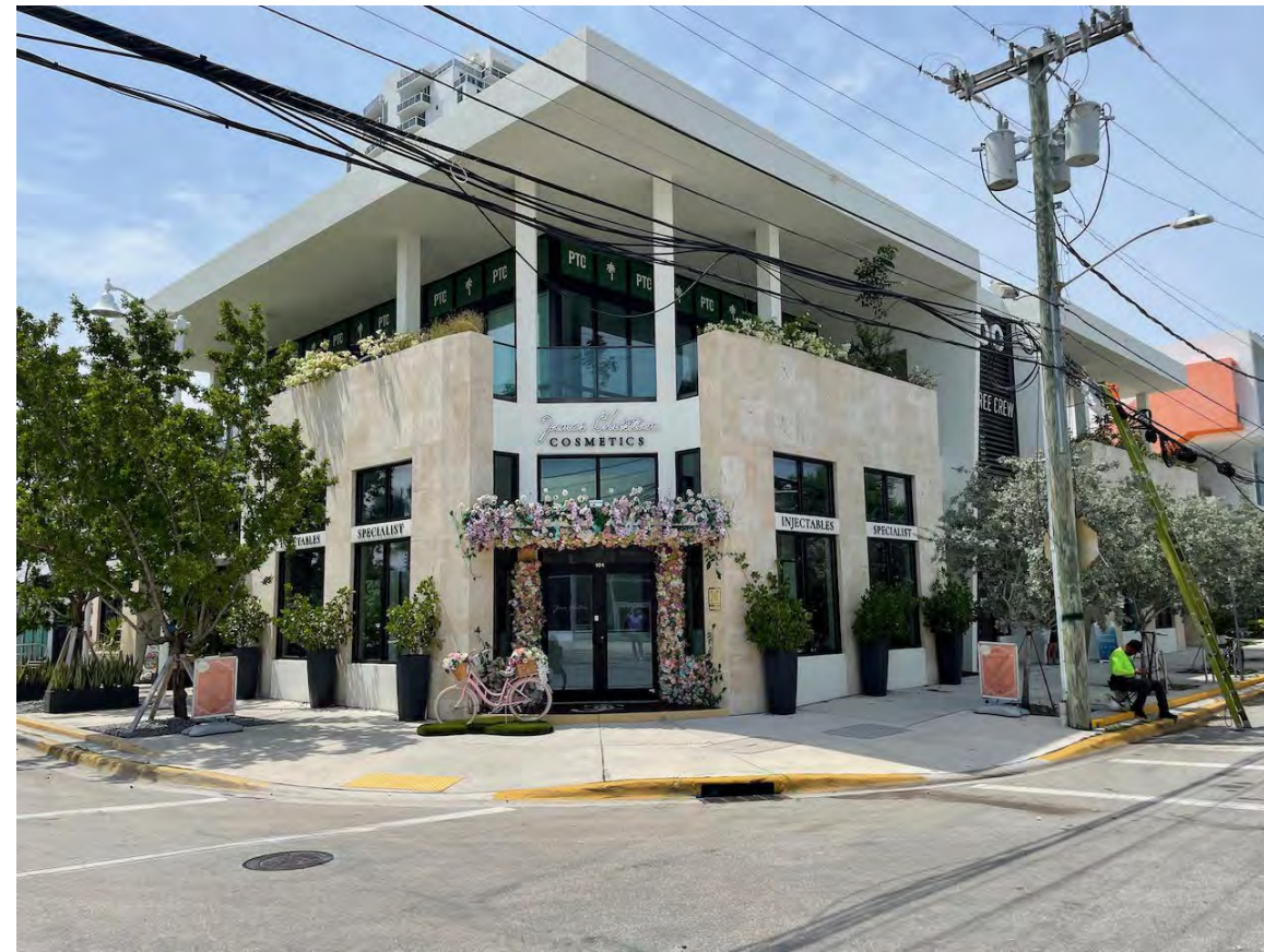
② FRONT BUILDING CONER ON THE NORTH FACADE
