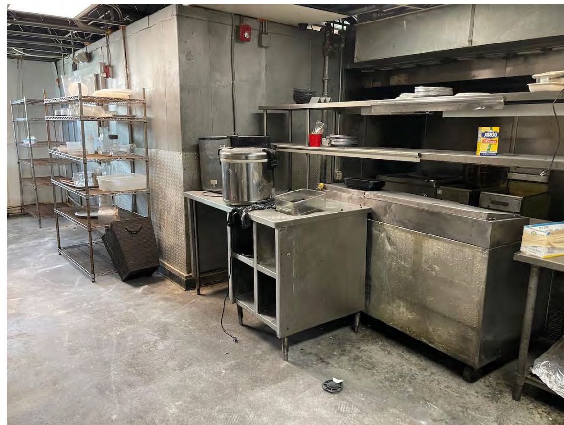
③ KITCHEN - EXISTING CONDITIONS - SECOND FLOOR LEVEL
