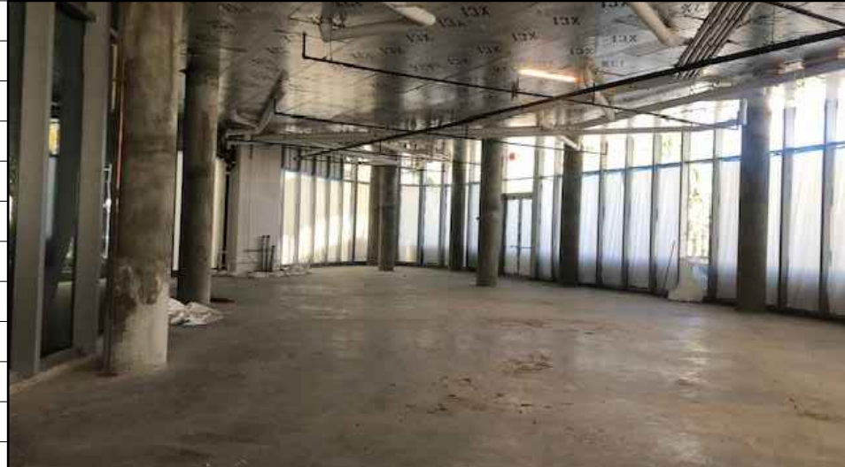
C INTERIOR - EXISTING CONDITIONS SCALE: NTS
