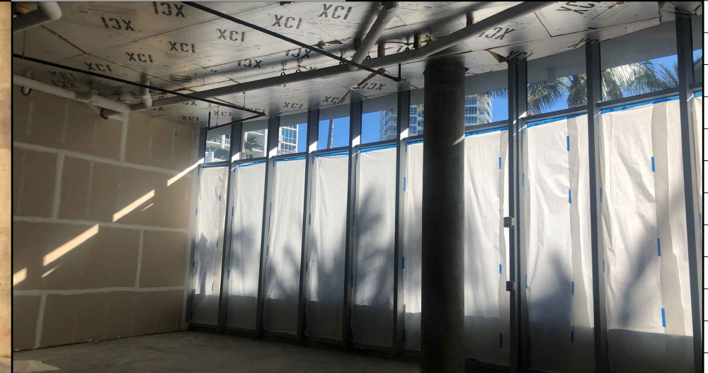
E INTERIOR - EXISTING CONDITIONS SCALE: NTS
