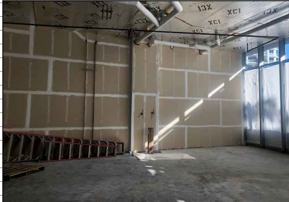
F INTERIOR - EXISTING CONDITIONS SCALE: NTS
