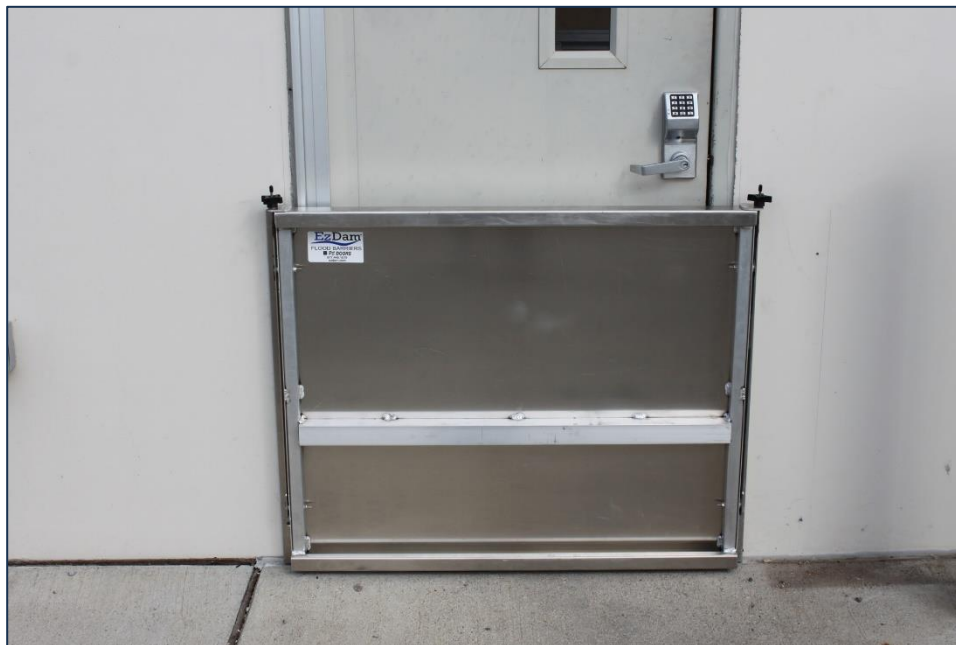
Figure 4. A temporary opening barrier deployed in front of a doorway. 5 Permanent components for anchoring the barrier to the building must be installed.
