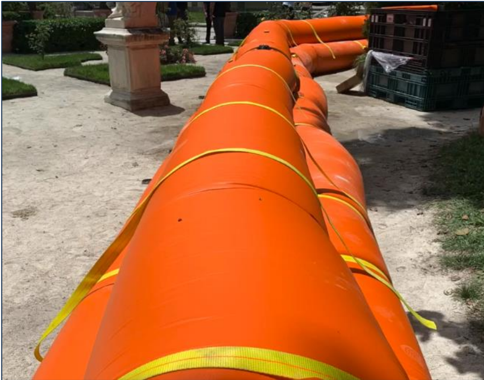
Figure 3. A temporary perimeter barrier installed at Vizcaya Museum & Gardens. The system shown is a bladder-style system which is filled with water and anchored to the ground as part of the deployment. 4
