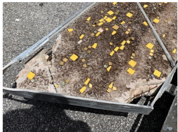
Detail of exposed aluminum tube, cracks, concrete loss and exposed corroded wire mesh on 'ground' panel during excavation.
