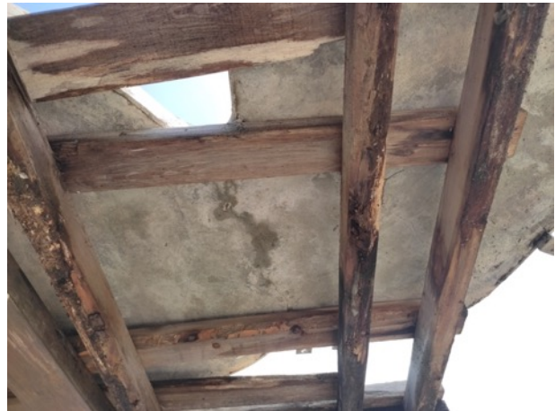
Detail of water infiltration at crack on the back of panel #17 during relocation.
