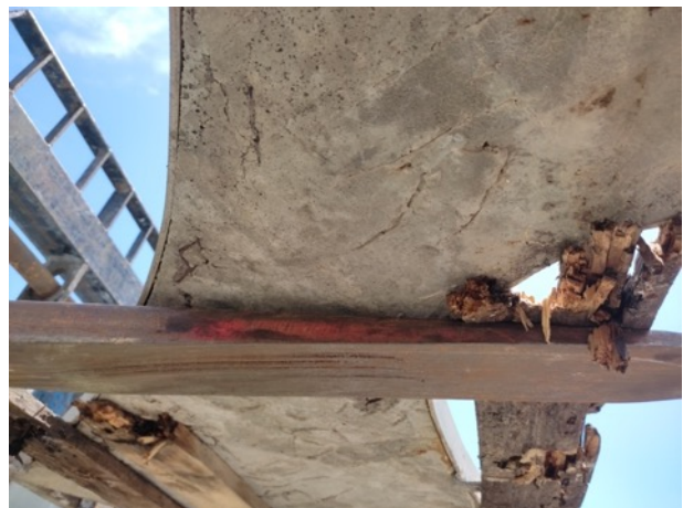
Detail of cracks, distinguishing marks and exposed wire mesh on the back of panel #18 during relocation.
